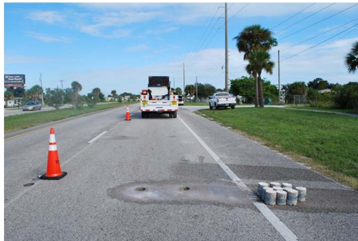
Figure 3-10. Coring on US-1 on wheel path and between the wheel paths.
