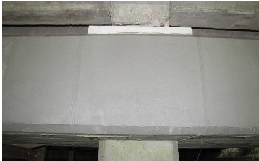
Figure 12 Final coating with short carbon fiber composite
