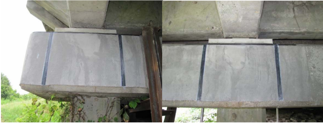
(a) View of carbon fiber tows in vertical direction at exterior column
