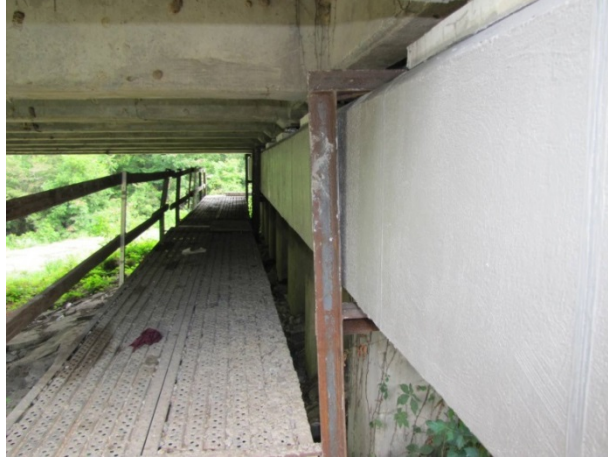
Figure 20 Appearance after the completion of second coat
