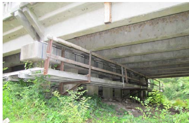
Figure 19 View of entire bent after placement of tows
