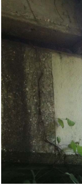
Figure 30 Self-Cleaning Property: Close-up of coated (on right) and non-coated (on left) surface highlights self-cleaning
