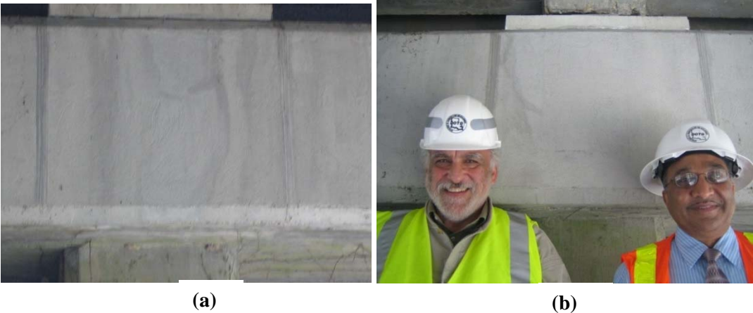
Figure 22 View of high modulus confinement composite: continuous carbon tows can be seen on both sides of the bearing plate
