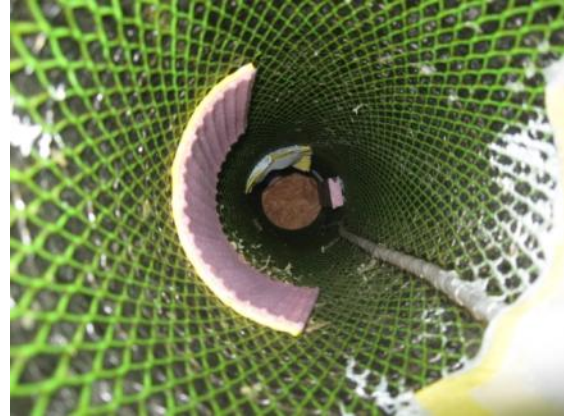
Figure 15: Inside of tube with artificial voids
