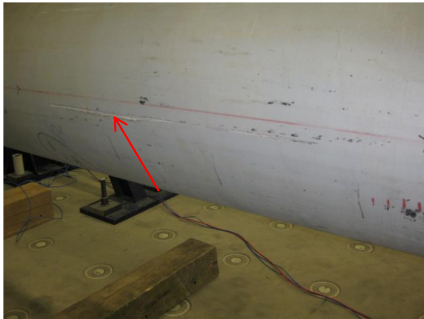
Figure 9: Scratch in FRP pile
