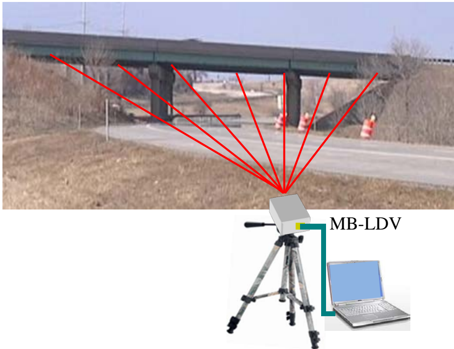
Figure 1. Concept of enhanced bridge inspection; I-55 over I-74 in Bloomington, IL (16).
