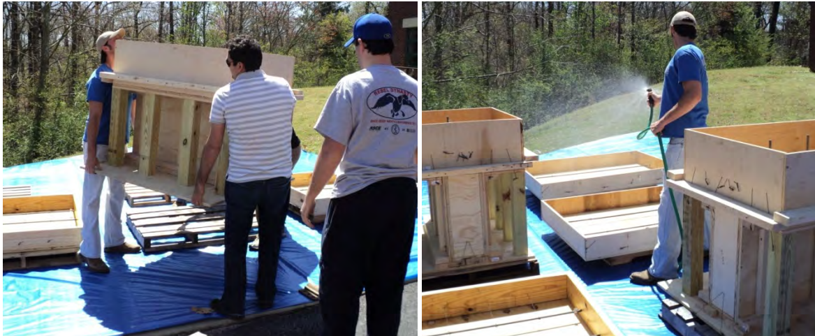
Figure 19. Moving and wetting the scale model bridge forms.
