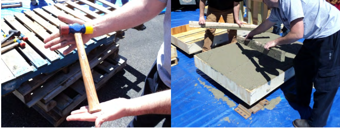
Figure 20. Hammers used for vibrating forms and volunteers striking off excess concrete.
