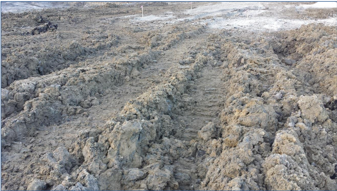
Figure 4. Glacial till soil placed in fill area
