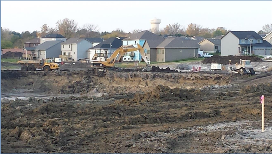
Figure 3. Excavation of the pond (middle left area of image)
