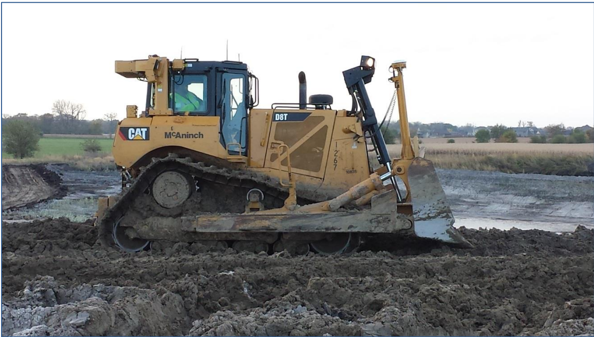
Figure 10. AMG CAT D8T bulldozer operations to spread fill
