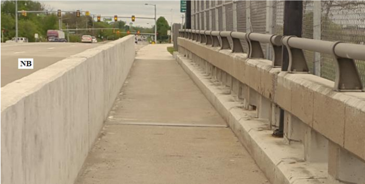
Figure 2-29. Pedestrian sidewalk on the east side of the bridge
