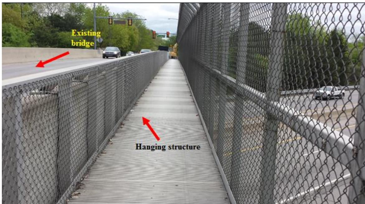
(b) Hanging structure
