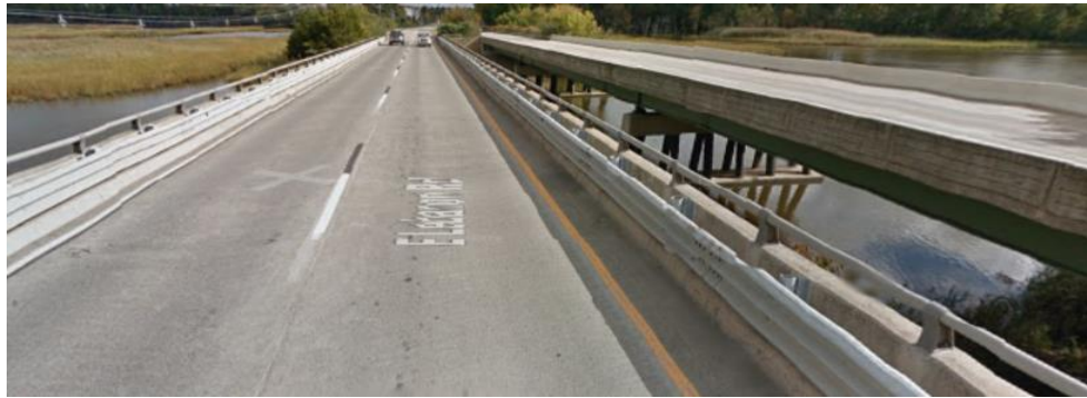
(b) Westbound bridge
