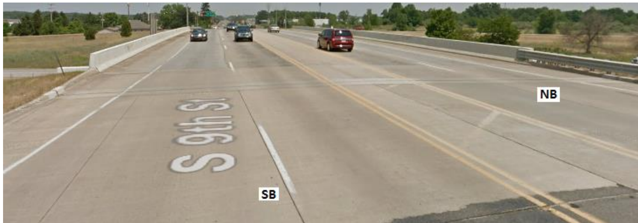
Figure 5-3. 9 th Street bridge over I-94 (Source: Google maps)
