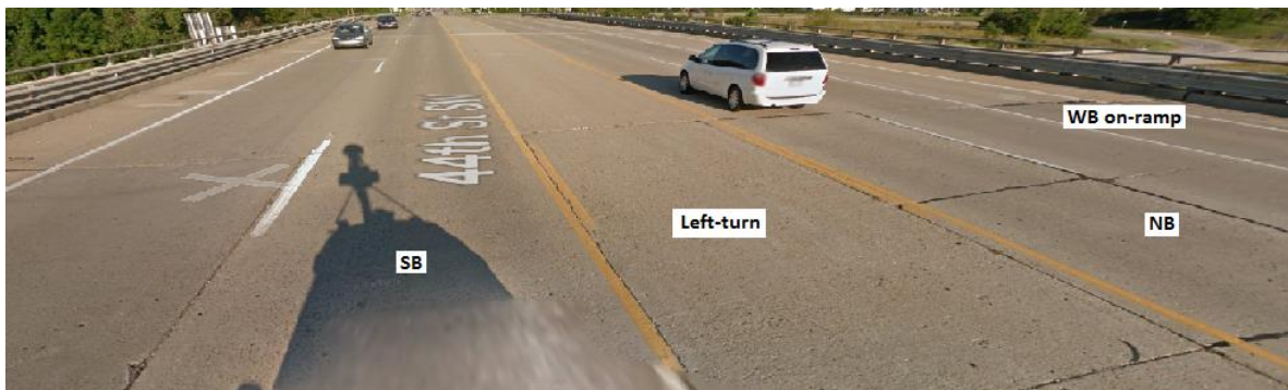
(b) A view of the bridge deck
