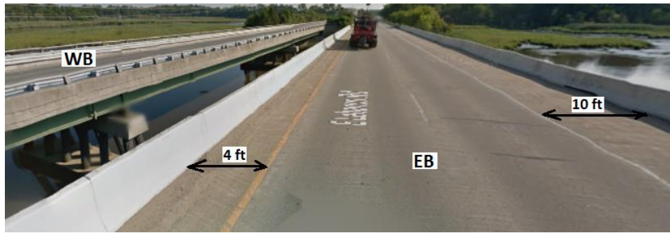
(a) Eastbound bridge
