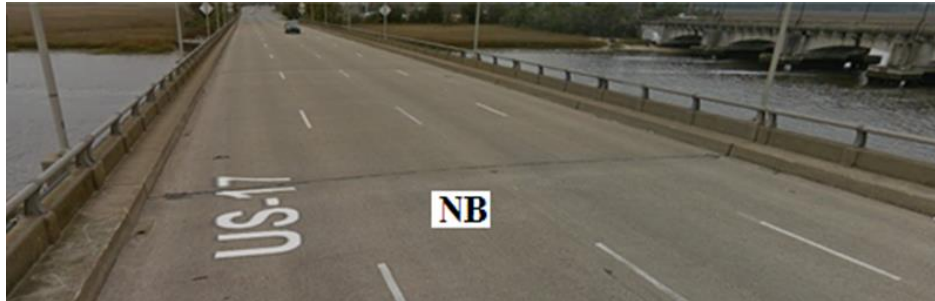
(a) Northbound bridge
