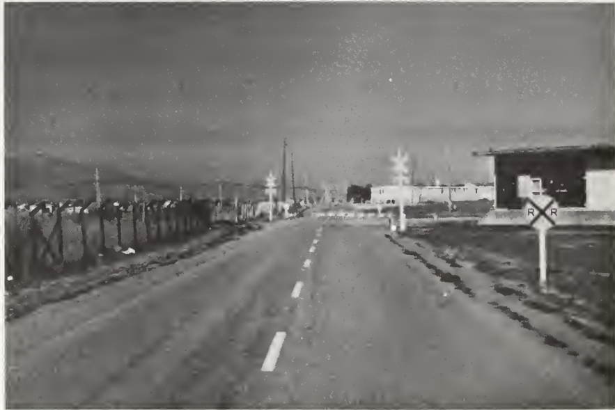
FIGURE 13 GATE PROTECTED CROSSING /GATE DOWN
