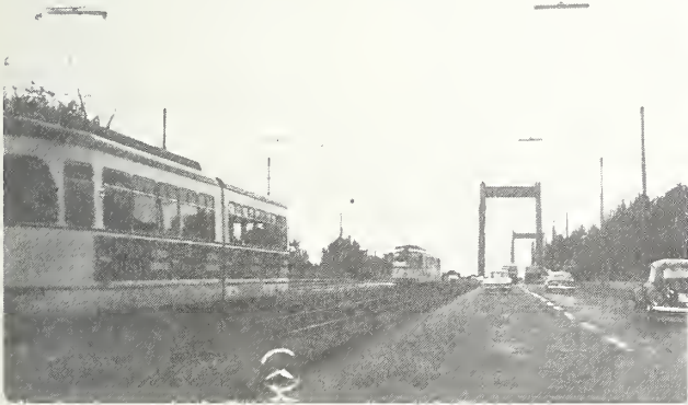
P-25. Median light rail ROW on a bridge (River Rhein, Cologne)
