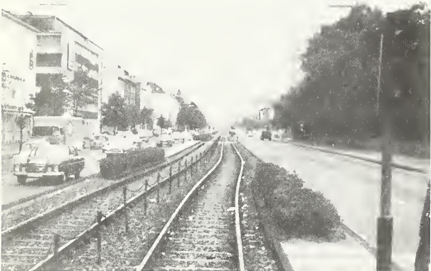
P-52. Staggered stops in a median to minimize ROW width (Cologne)
