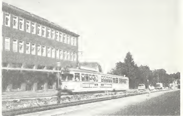
P-28. Track reconstruction from pavement into the median private ROW (Bielefeld)
