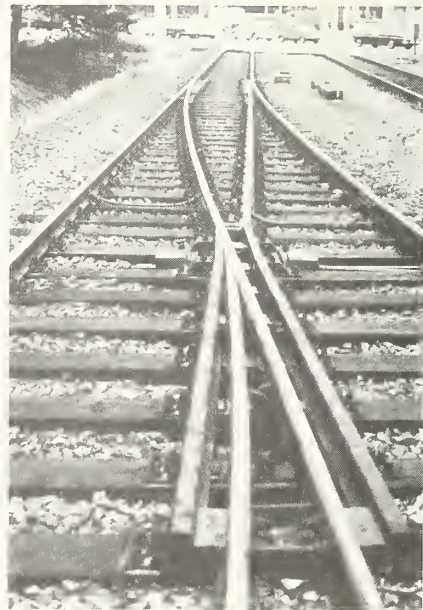
P-49 . The same switch in turning out position (Cologne)
