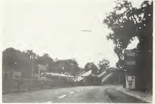
P-53. Protected median ROW and station with grade separated pedestrian access (Cologne)
