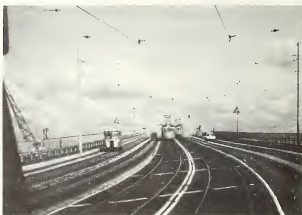
P-23. Transit lane on a bridge separated by markings, used by light rail and buses (Gothenburg)
