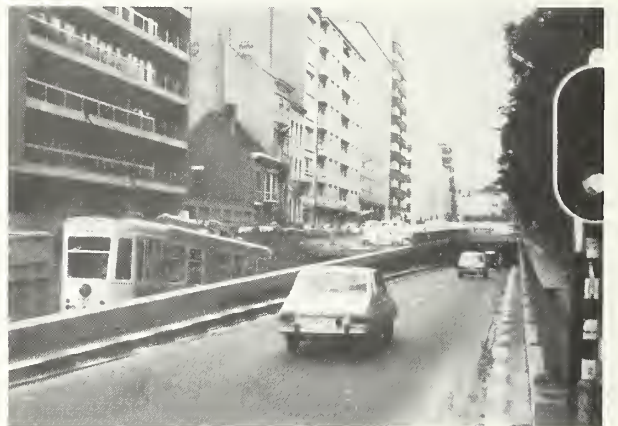
P-46. Tunnel access ramp (Brussels)
