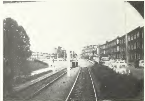
P-40 . Light rail underpass of a busy intersection (Rotterdam)
