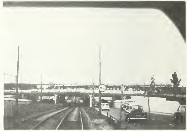
P-39 . Undercrossing of the main-line railroad (Rotterdam)
