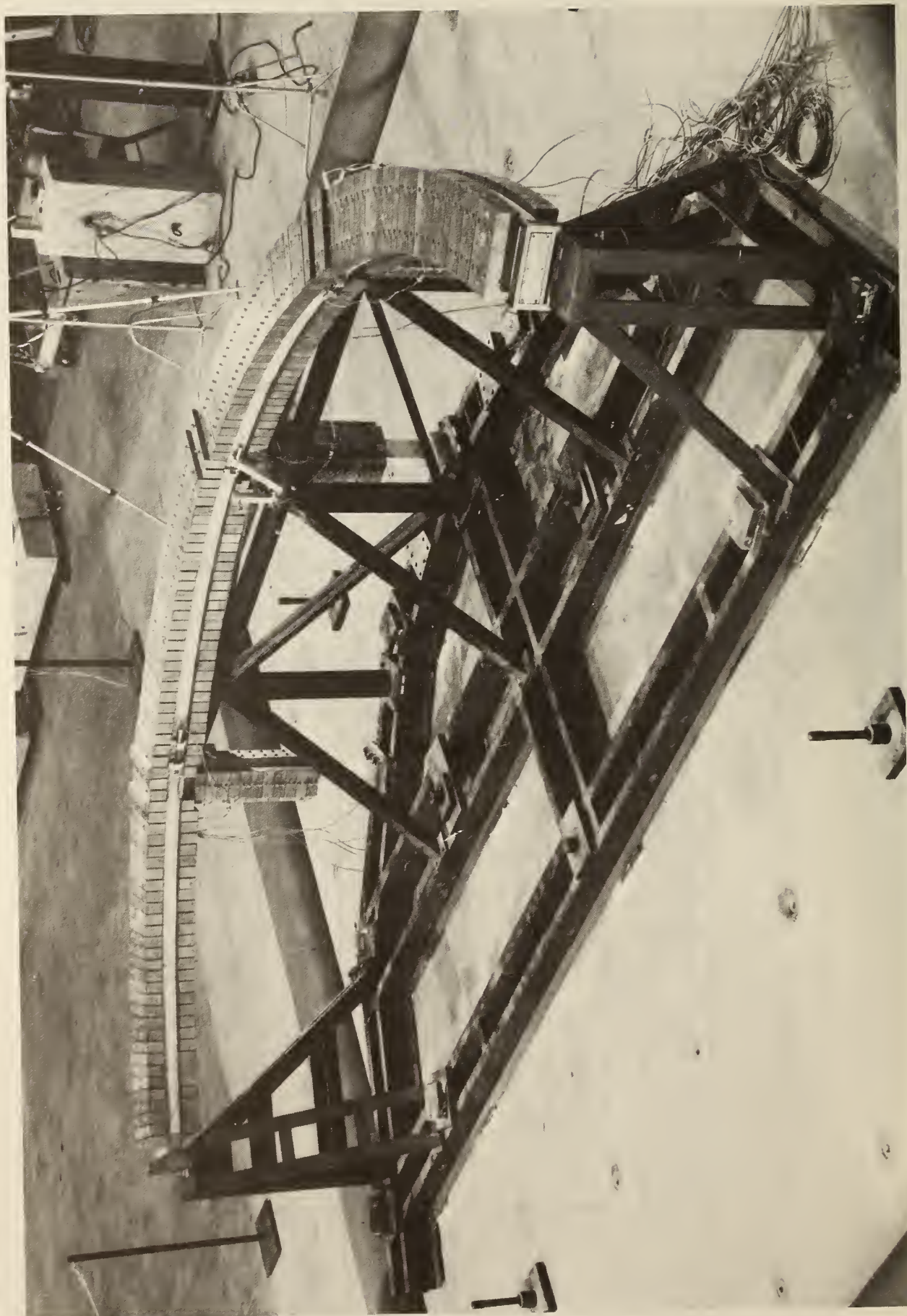
FIG. 4.1 EXPERIMENTAL MODEL BRIDGE STRUCTURE
