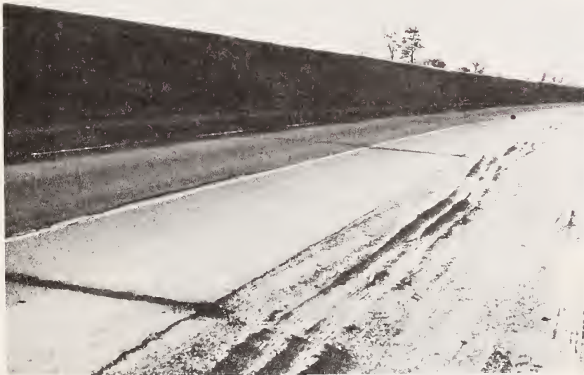
Figure 6.8. Transverse Mini-Drain System in California.
