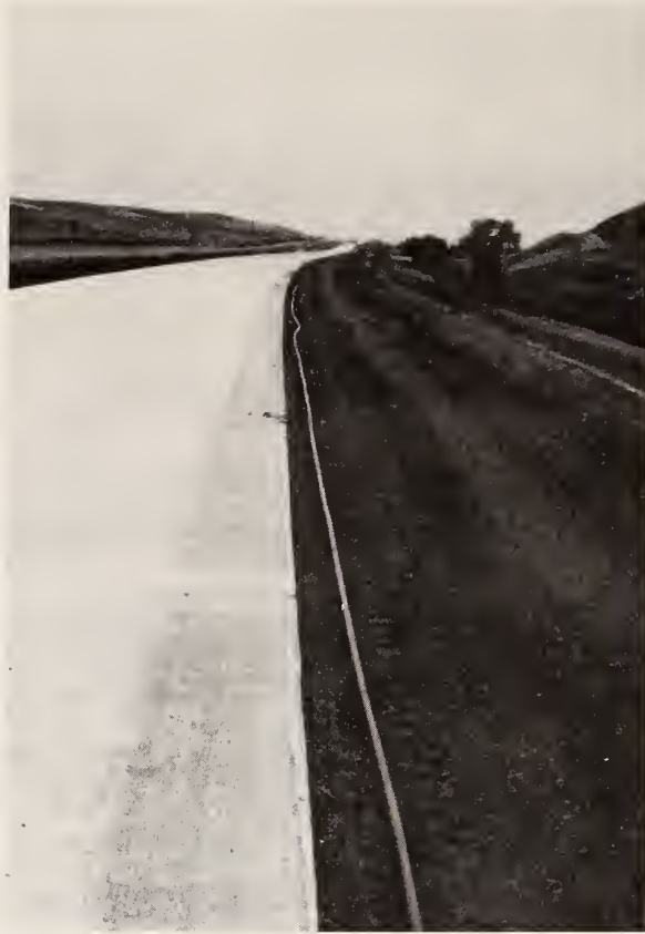
Figure 6.1. Mini-Drain System in California.
