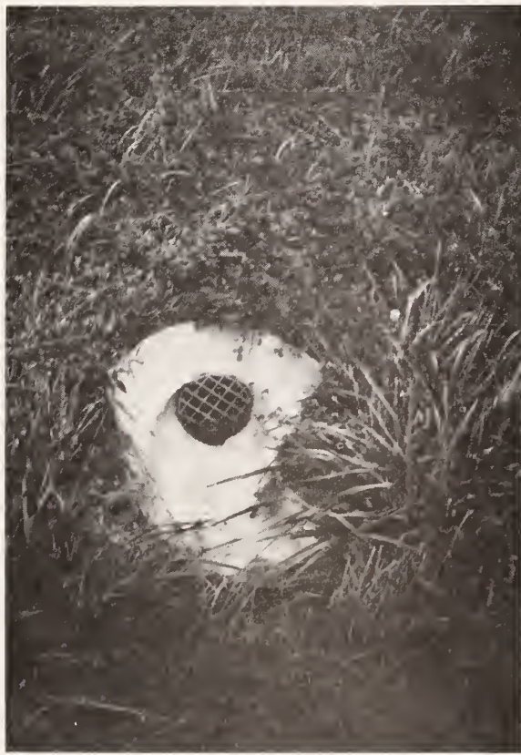
Figure 6.11. Formed In-Place Subdrain Outlet.
