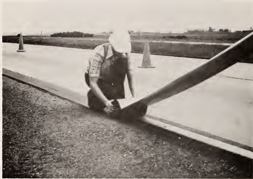
Figure 6.17. Placement of Rubberized Asphalt Strips.
