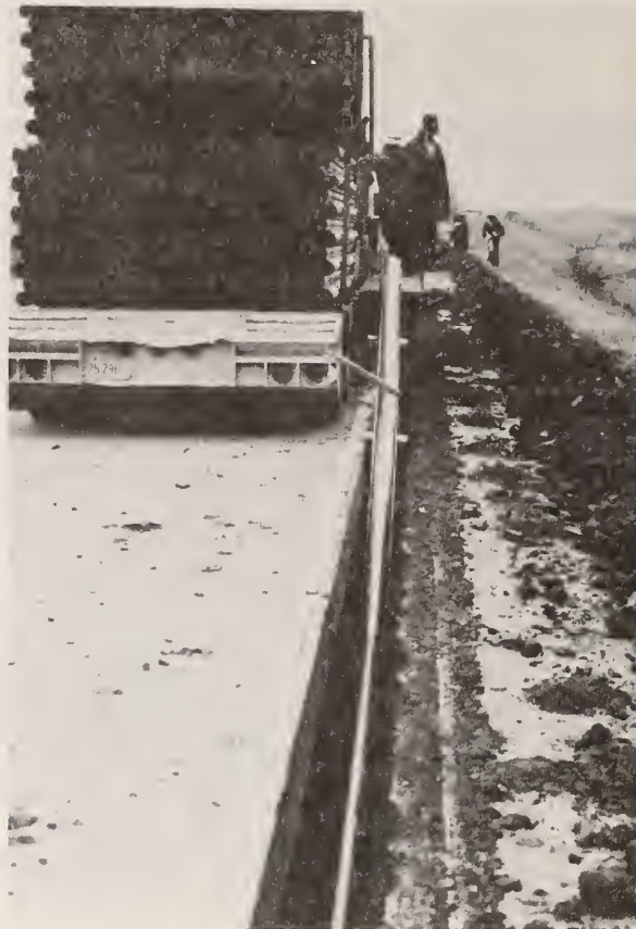
Figure 6.5. Bituminous Fiber Pipe Subdrain Installation.
