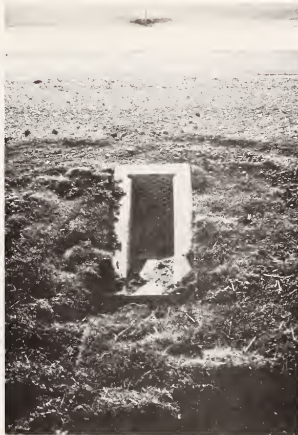
Figure 6.12. Preformed Subdrain Outlet Headwall and Splashblock used in Illinois.
