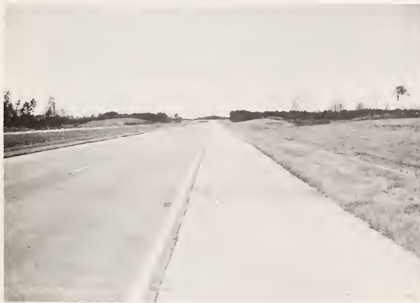
Figure 6.15. Concrete Shoulder on FAI 16 in Georgia.
