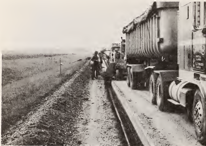
Figure 6.22. Placement of Subdrainage Envelope Material.
