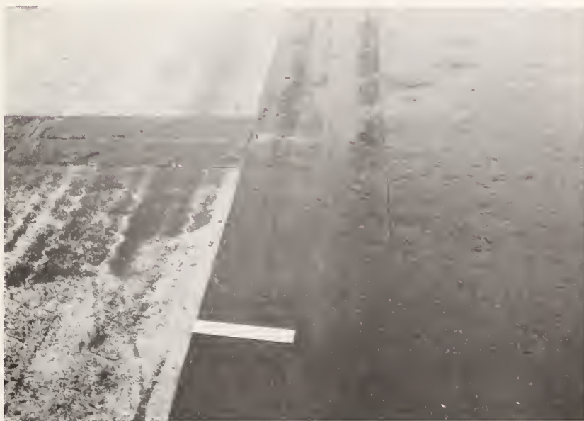
Figure 6.16. Rubberized Asphalt Strips for Pavement Rehabilitation in Georgia.
