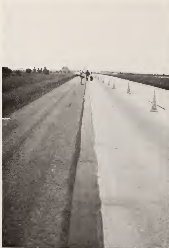
Figure 6.18. Sealing Edge Joint with Rubberized Asphalt Strips in Illinois.
