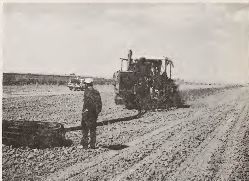
Figure 6.6. Installation of Corrugated Plastic Tubing.
