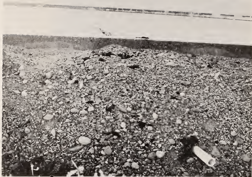
Figure 6.9. Transverse Mini-Drain Outlet.
