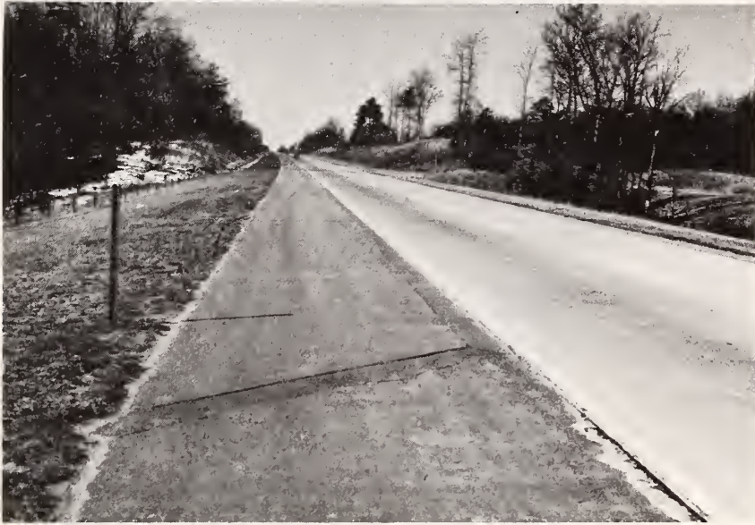
Figure 6.3. Intermittent Longitudinal Subdrain in Virginia.
