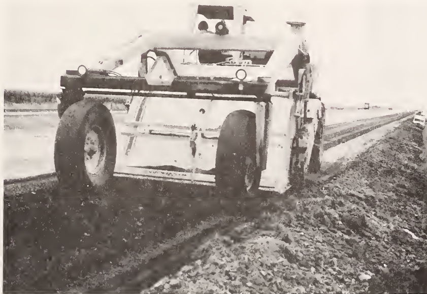
Figure 6.24. Pulverization of Asphalt Shoulder for Recycling.
