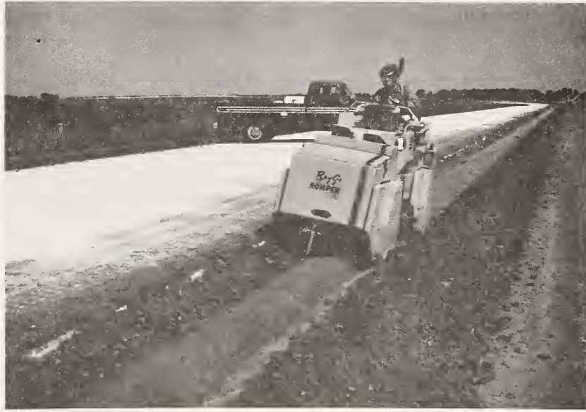
Figure 6.23. Compaction of Subdrainage Trench Backfill Material.
