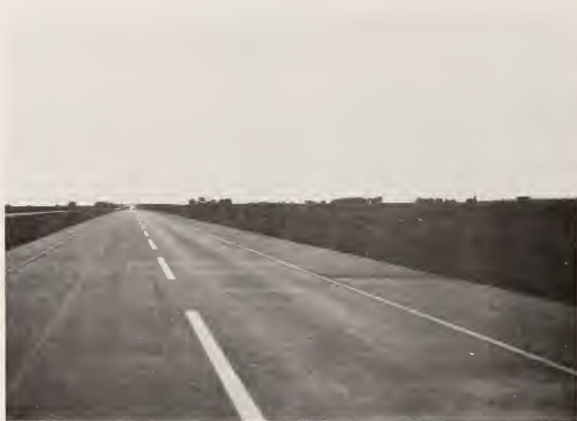
Figure 6.14. Concrete Shoulder on Illinois Toll Road.
