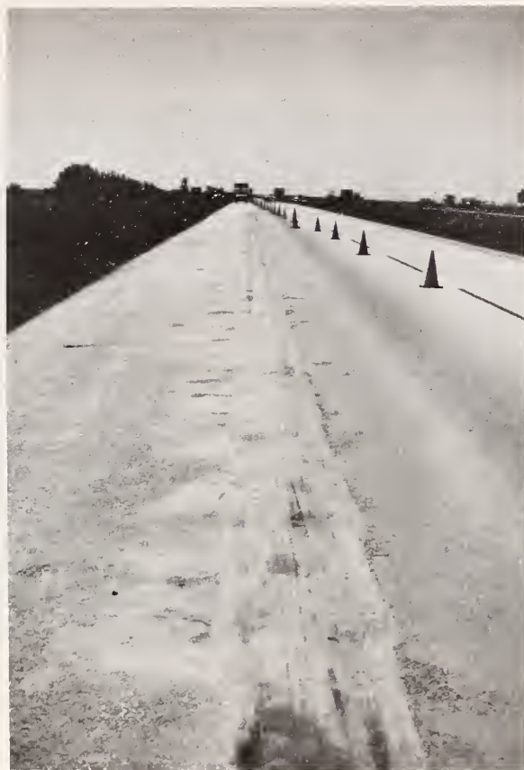
Figure 6.19. Completion of Membrane Strip in Illinois.
