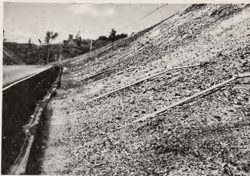
Figure 6.10. Transverse Mini-Drain System for Slope Stability.
