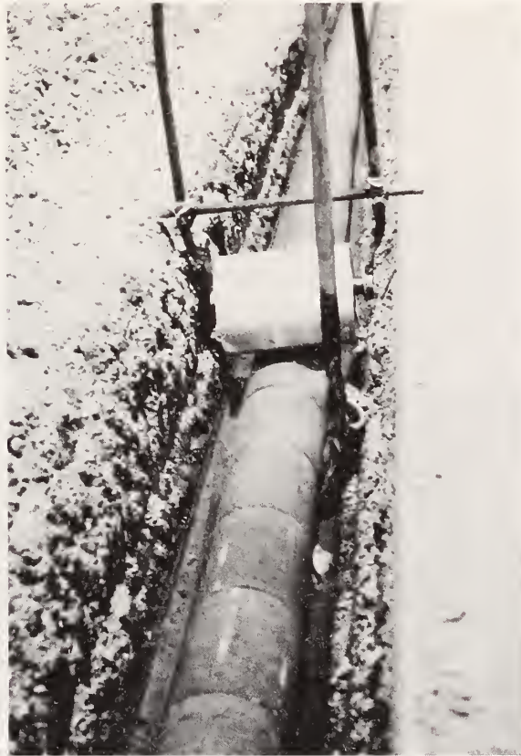
Figure 6.4. Concrete Subdrain Pipe.
