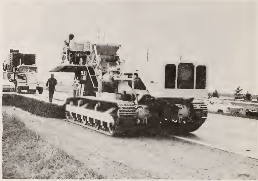
Figure 6.21. Trenching Equipment for Subdrainage Installation.
