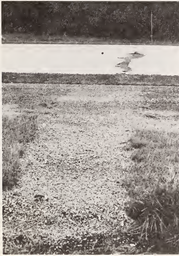
Figure 6.7. Transverse Drainage System in New York.
