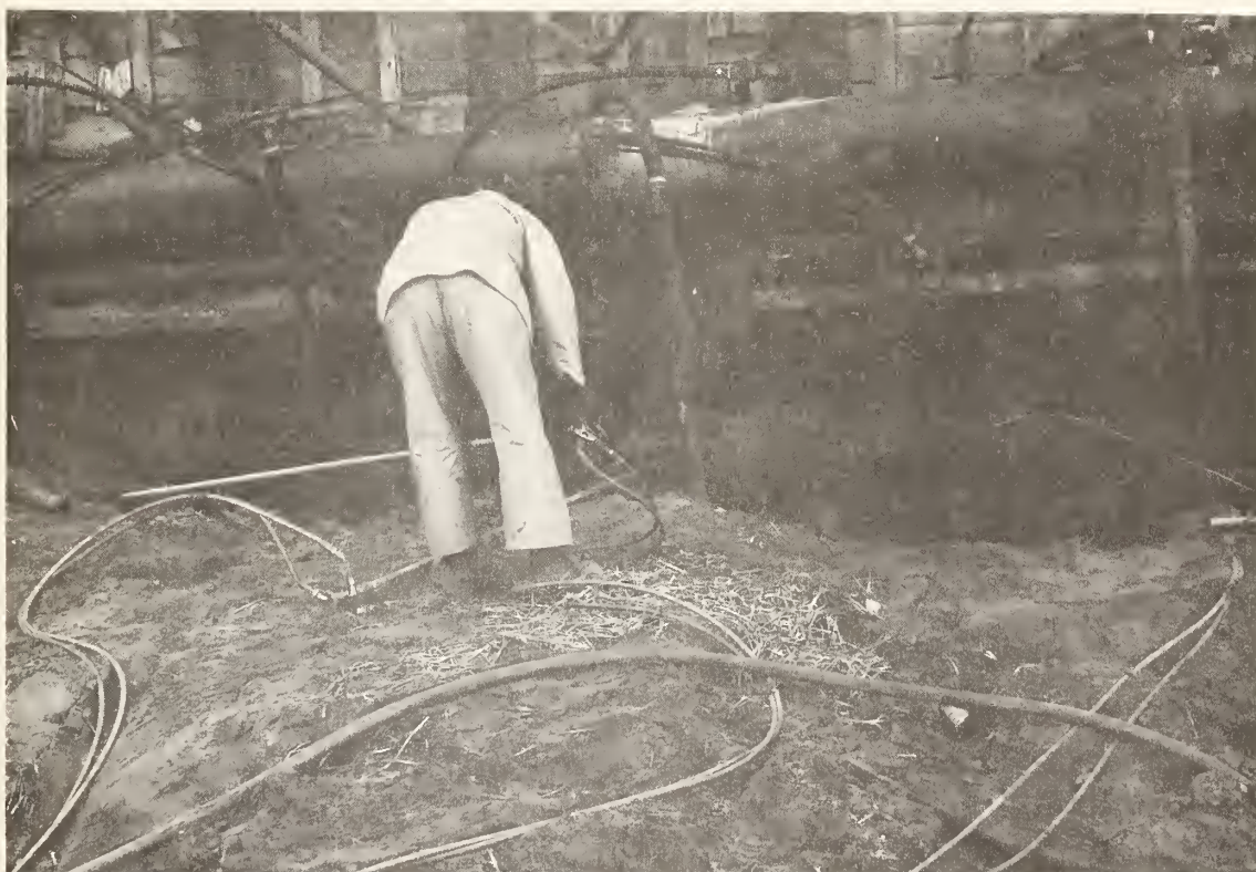
Figure 11. Grouting to consolidate sand behind wood lagging.
