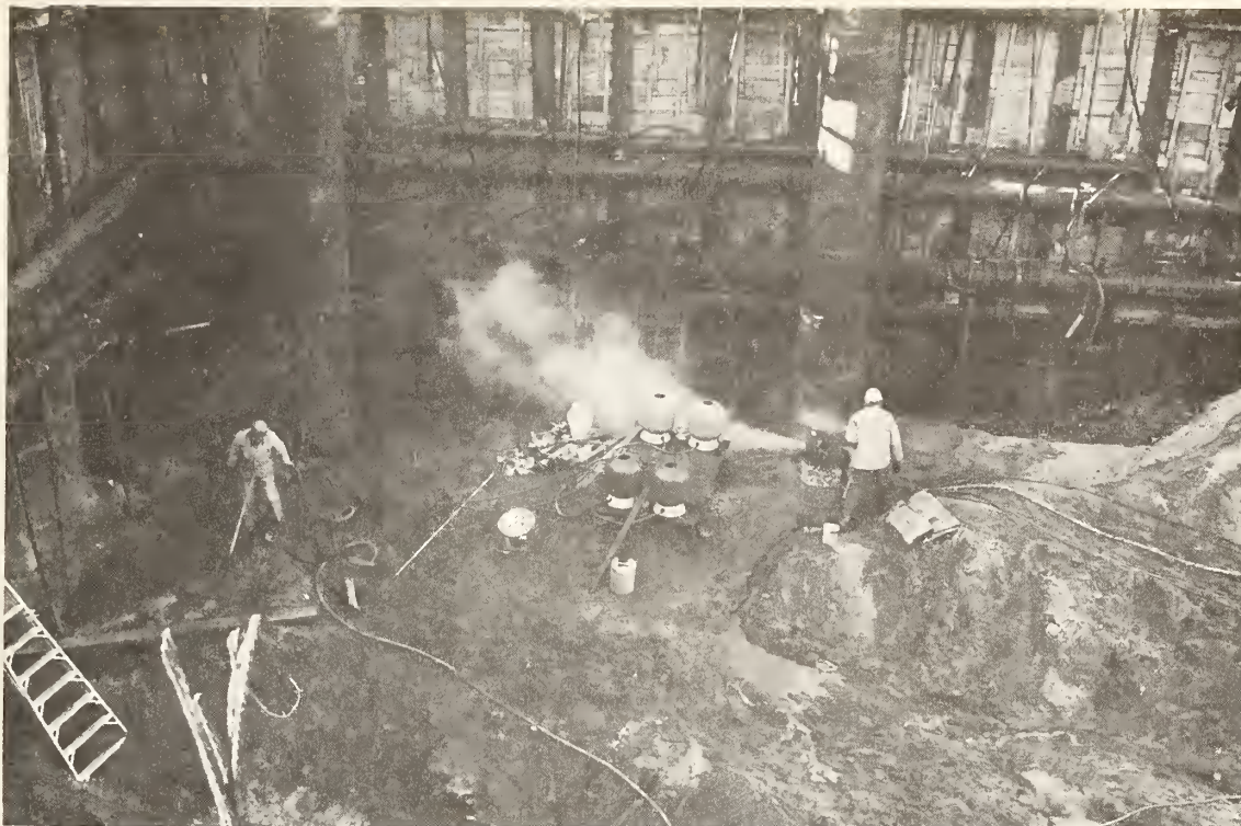
Figure 10. Small grouting job in cut-and-cover construction.
