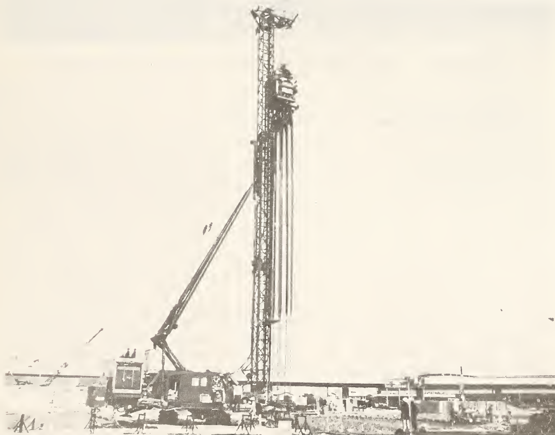
Figure 15. Machine for placing packer element and connector tubing.
