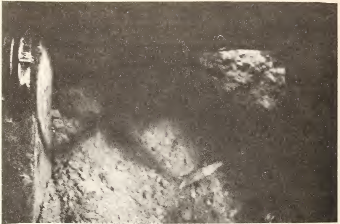
Figure C-21. Grouted soil at tunnel face.
