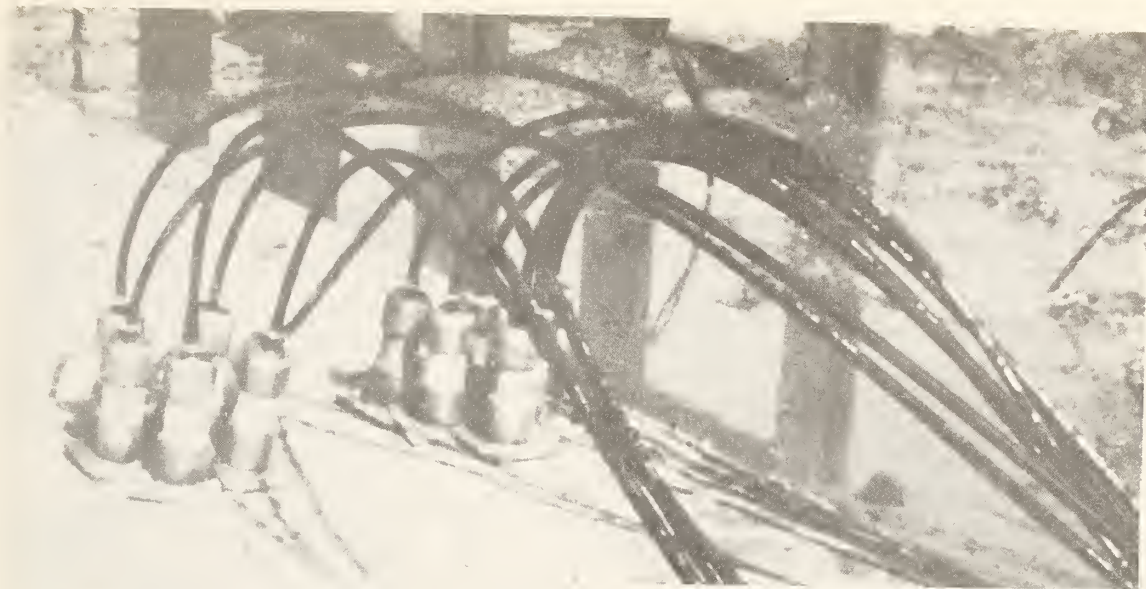
Figure 14. Packer element and connector tubing used in Europe.
