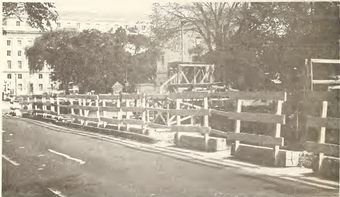
Figure C-9. Washington grouting site.
