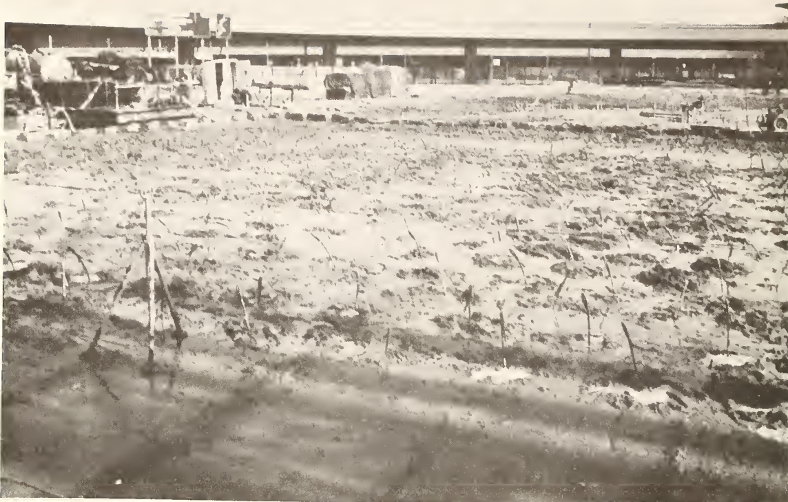
Figure 16. Grouting tubes in place for grout injection.
