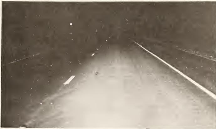
Figure 25. Centerline of 5-foot (1.52-m) stripes and a reflective RPM in alternate 35- foot (10.67-m) gaps.
