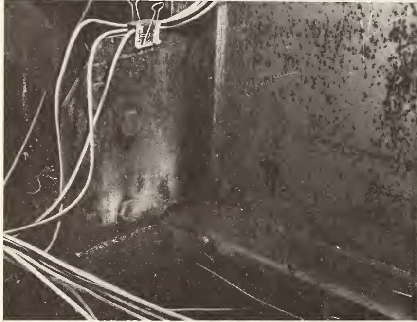
Fig. 60 Web Crack Repairs - Location ww on Girder 2 of Assembly 3
