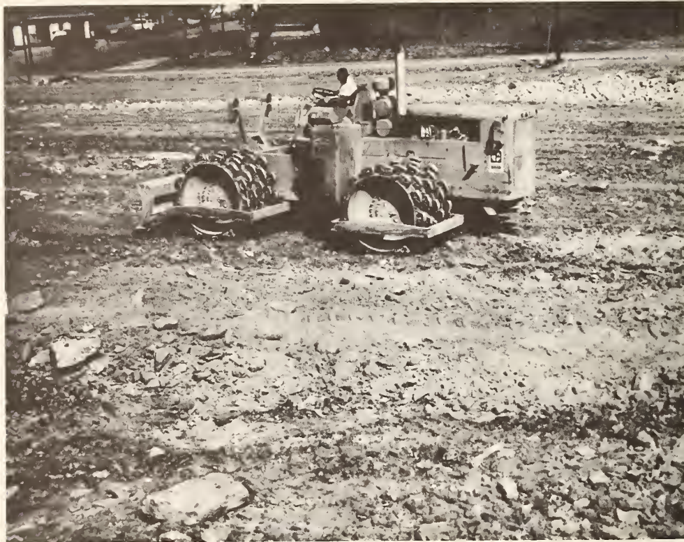
Figure 33. Four-wheel compactor dozer
