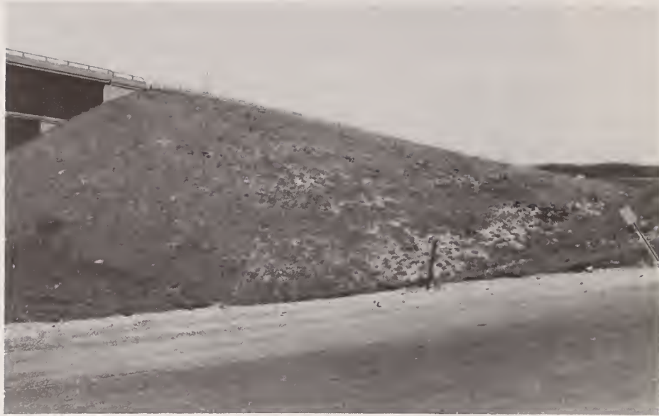
a. East approach embankment
