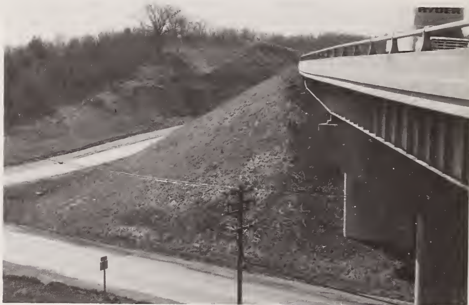
b. West approach embankment
