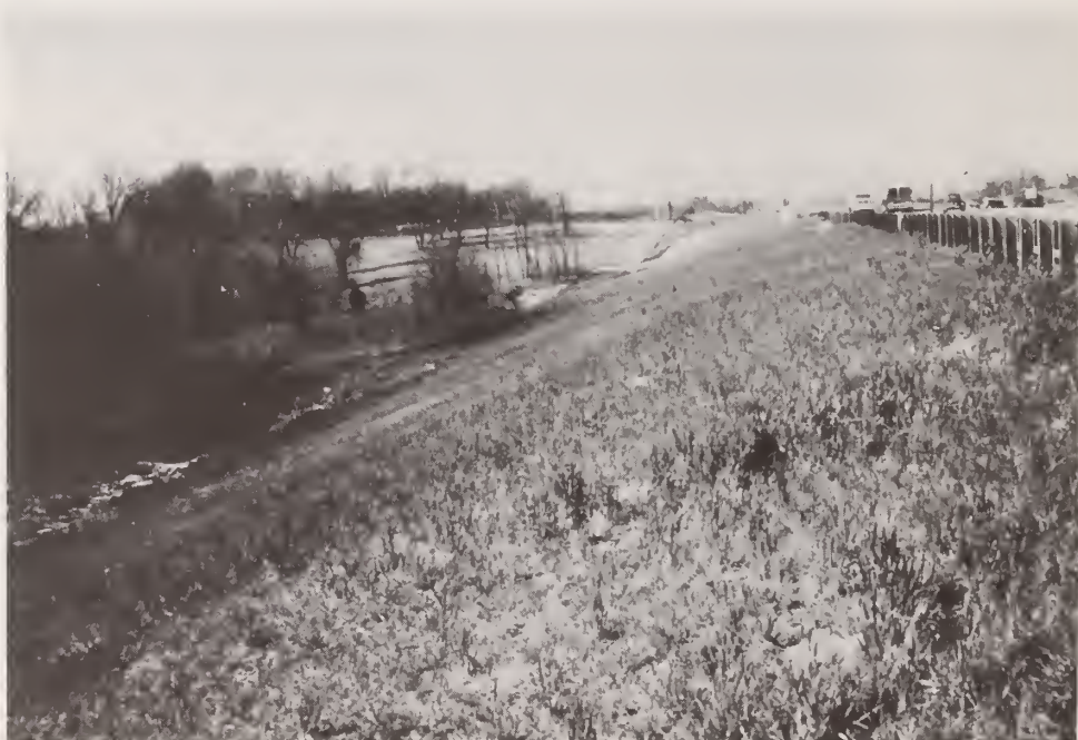
Figure 9. General view of I-75, Kentucky shale embankment after reconstruction MP 179.7 to 179.9
