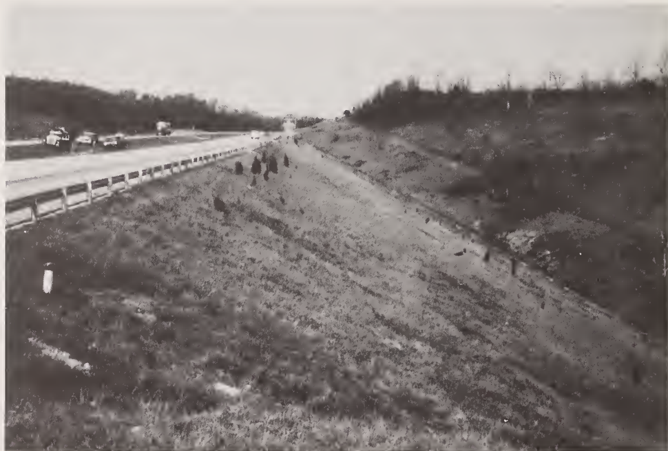
Figure 14. Indiana I-74 embankment, sta. 426+00 to 440+40 (north slope, looking west)
