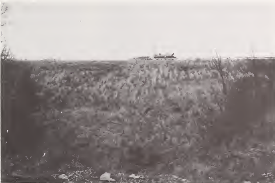
Figure 6. U. S. 460 West Virginia embankment
