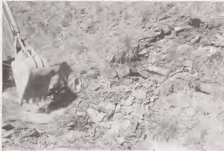
Figure 5. Excavating unweathered parent shale chunks, Tennessee I-75
