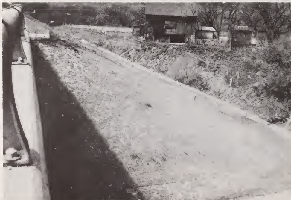
Figure 13. West approach embankment I-74, Ohio at Wesselman Road
