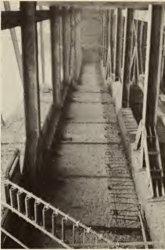
FIGURES 90-91. MULTIPLE-AUGER RIG AND EXPOSED SLURRY WALL. (By permission of Tone Boring Co.)
