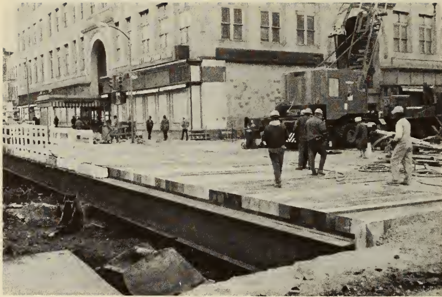
FIGURE 50. WASHINGTON, D. C. METRO, Decking 11th and G Street
