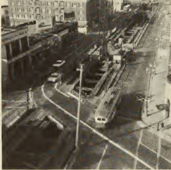
FIGURE 57. EXCAVATING FROM THE LOAD PLATFORM (Courtesy of Fruin-Colnon Contracting Company.)
