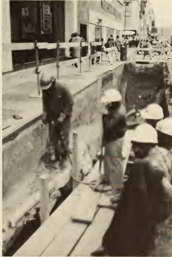
FIGURE 45. WASHINGTON, D. C. METRO, Exposing the Utilities
