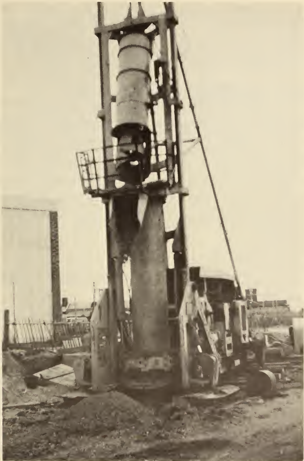
FIGURE 105. BENOTO RIG DRILLING HOLES, London, England.
