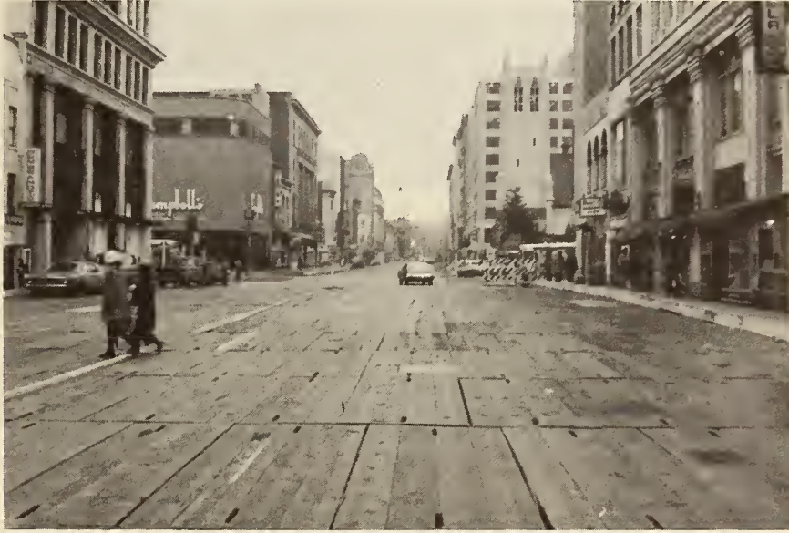
FIGURE 52. WASHINGTON, D. C. METRO, G Street Deck in Place
