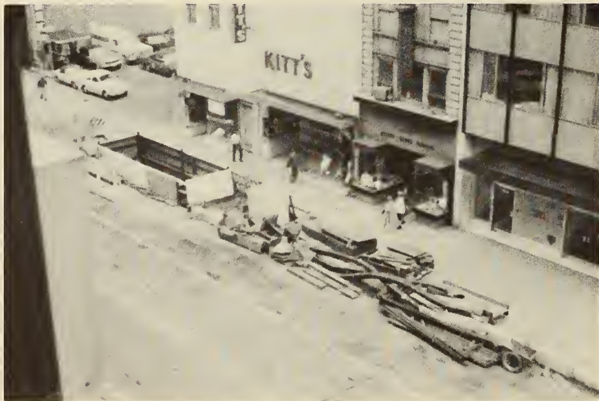
FIGURE 51. WASHINGTON, D. C. METRO, Decking and Access Opening
