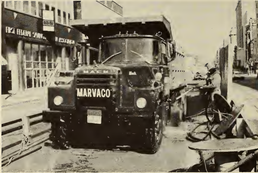
FIGURE 1. WASHINGTON, D.C. METRO, Truck Wheel-Washing Station
