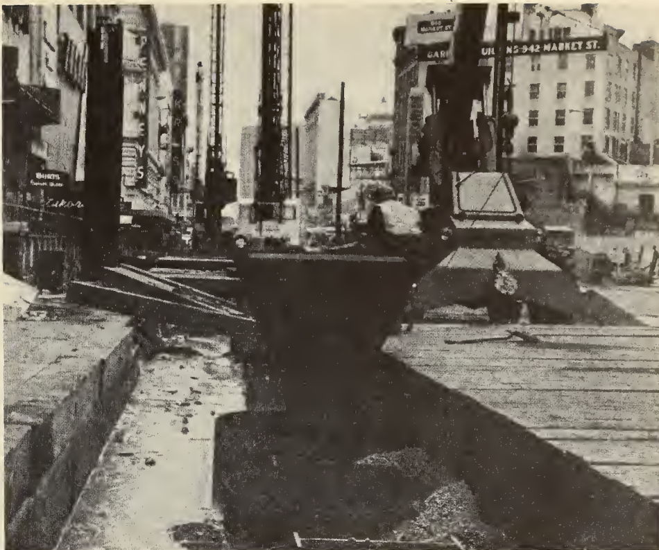
FIGURE 93. BART, SAN FRANCISCO, SPTC METHOD. Backfilling a vertical H-beam.
