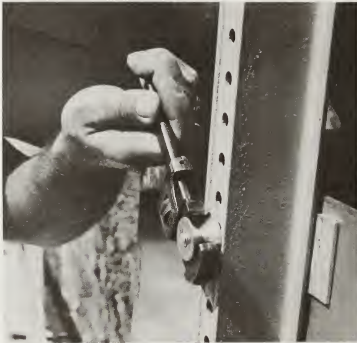
(a) TIGHTENING SECURITY FASTENER
