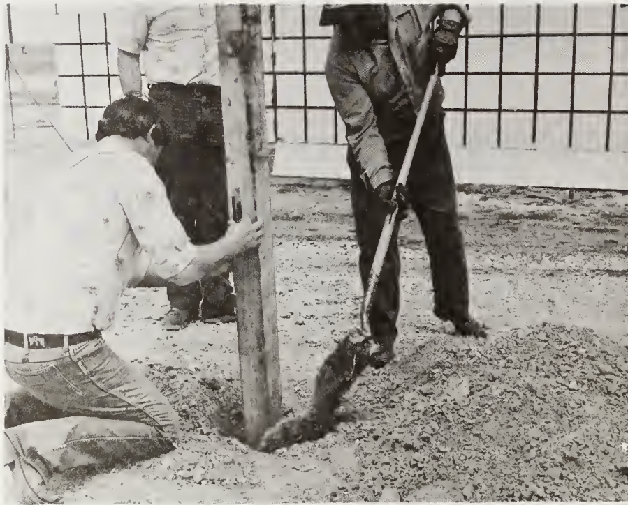
(a) BACKFILLING
