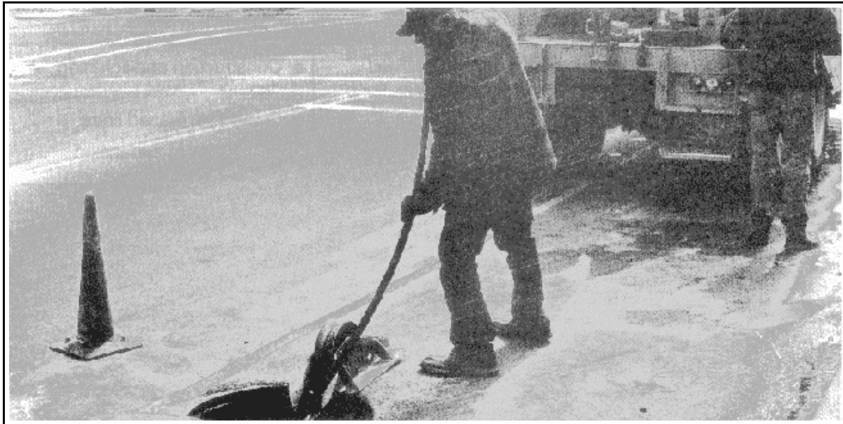
Figure 8-1 Installing Communications Cable
