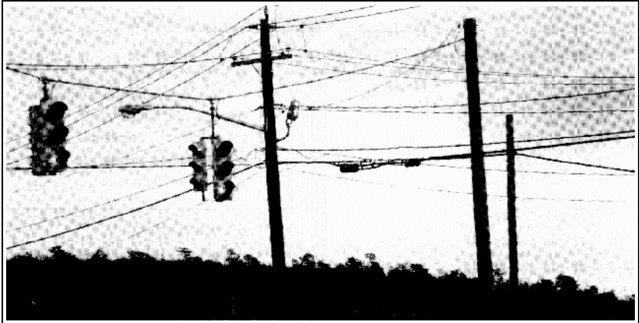
Figure 6-1 Telephone Company Lines
