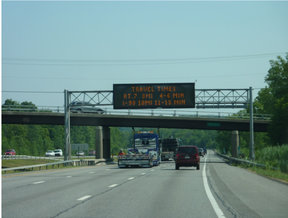
Figure 28. Variable Message Sign
