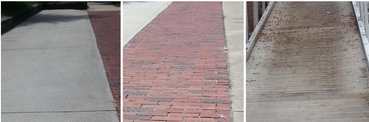
Figure 15. View of the Three Surfaces Tested
