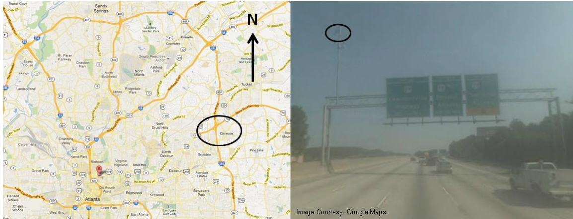
Figure 17: Gantry-mounted VDS Camera Location on I-285 near US-78
