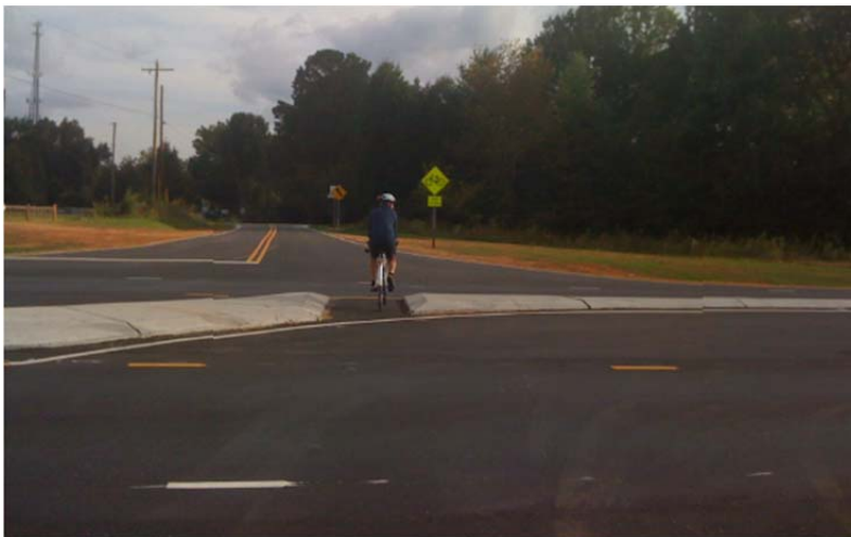
Figure 30: Bicyclist Passing Across a Channelized Island at an RCUT
