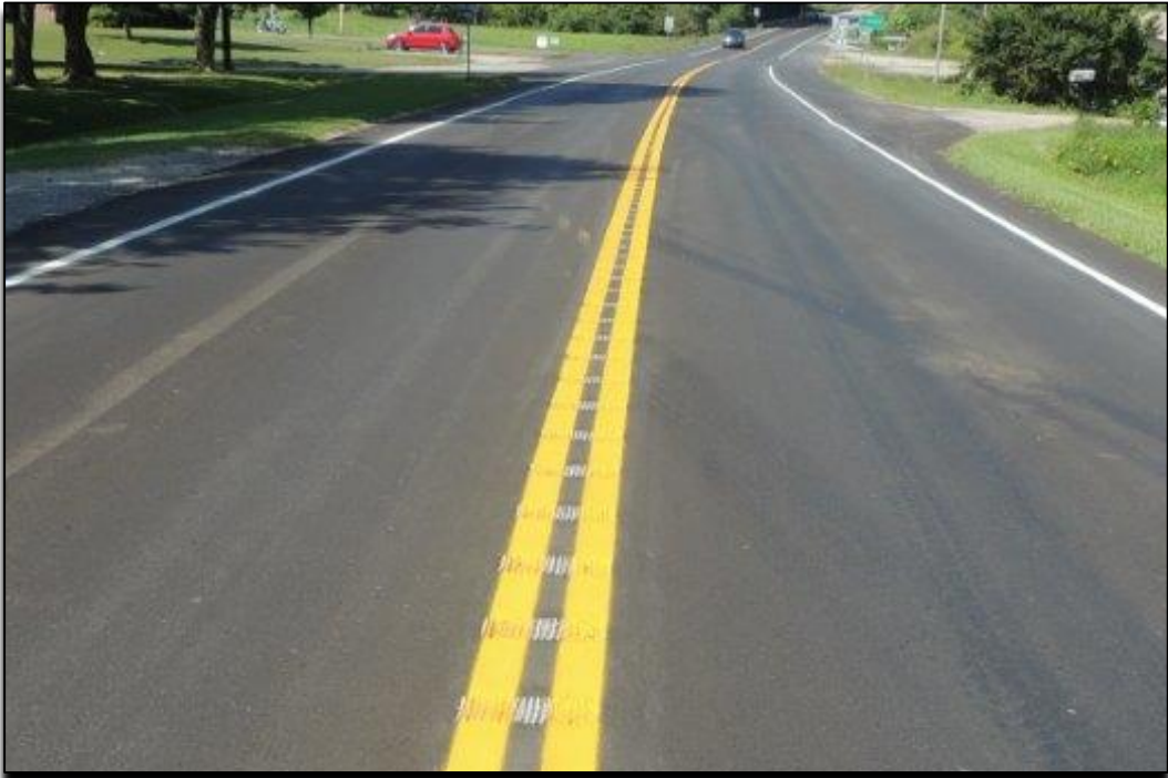
Source: U.S. Hwy 60, Franklin County, KY
