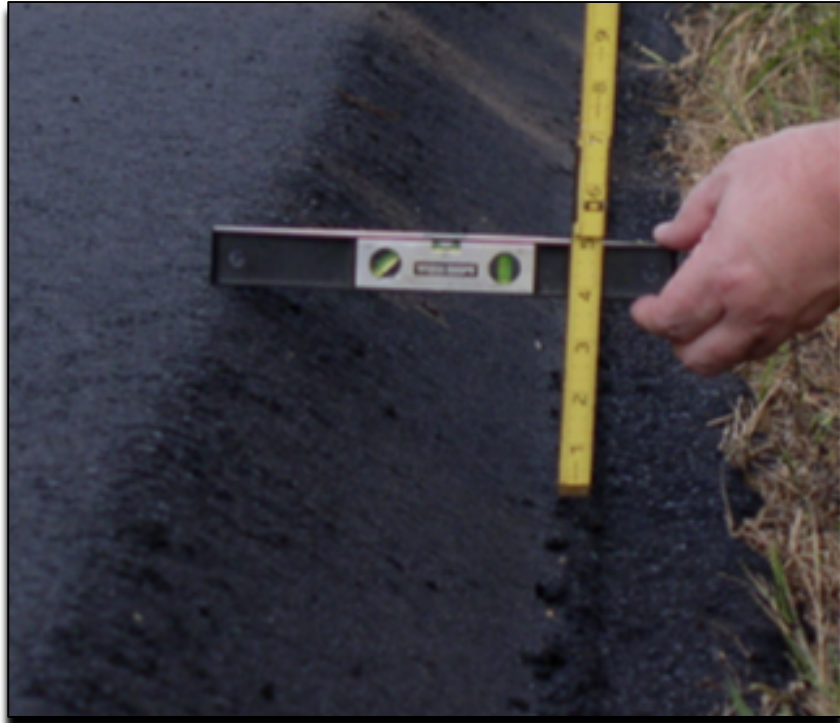
Figure 9: Pavement with Safety Edge
