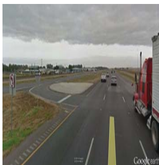
Restricted median opening on US-90
