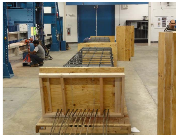
Figure 3.12: Installing edge & side Panels
