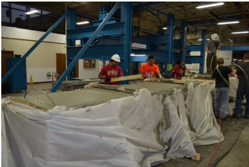
Figure 3.22: Casting of Box Beams, S1-1 and S1-2
