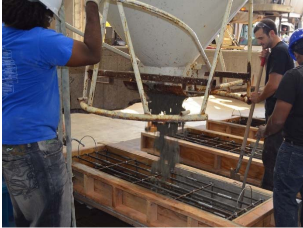
Fig. 3.40: Placing of concrete
