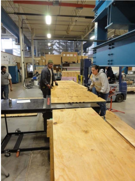
Figure 3.4: Construction of formwork.
