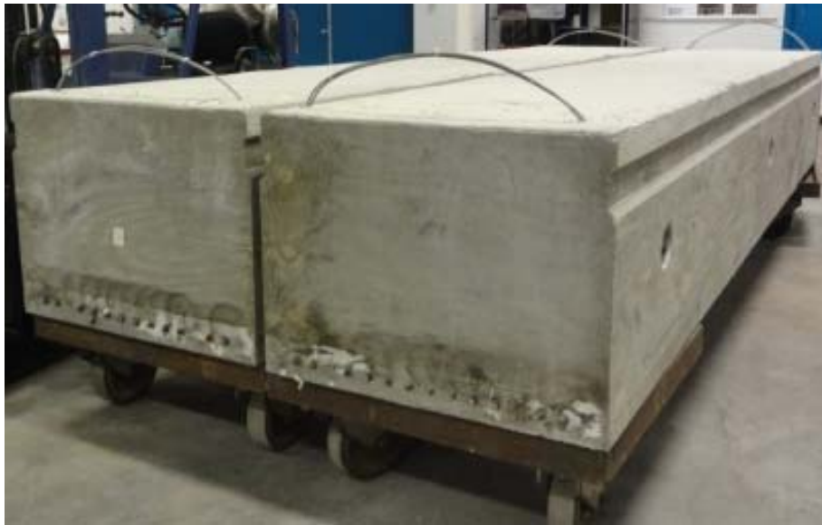
Figure 3.1: Specimen 1 Box Beams, S1-1 and S1-2.
