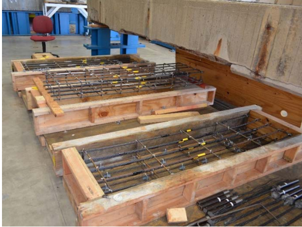
Figure 3.37: Cages of reinforcement and strands
