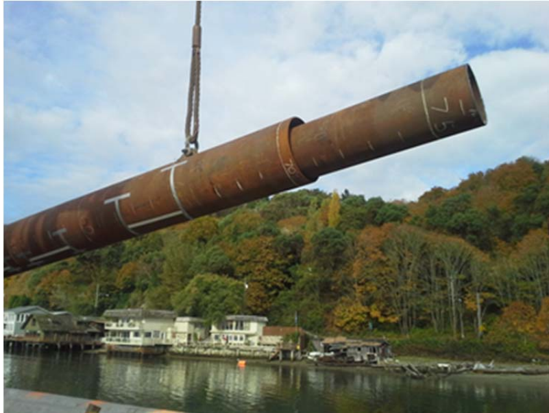
Figure 26: Lofting of the double pile
