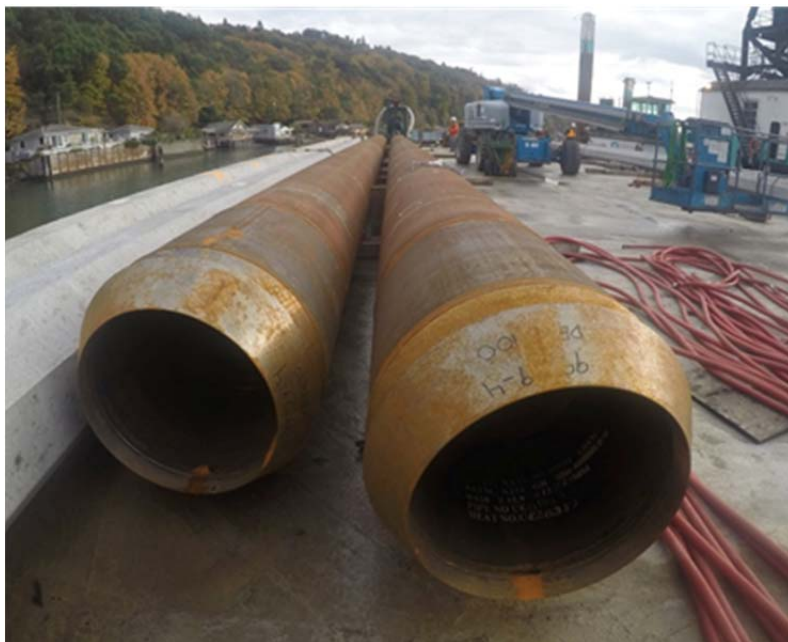
Figure 18: Full-scale double pile and mandrel double piles before installation
