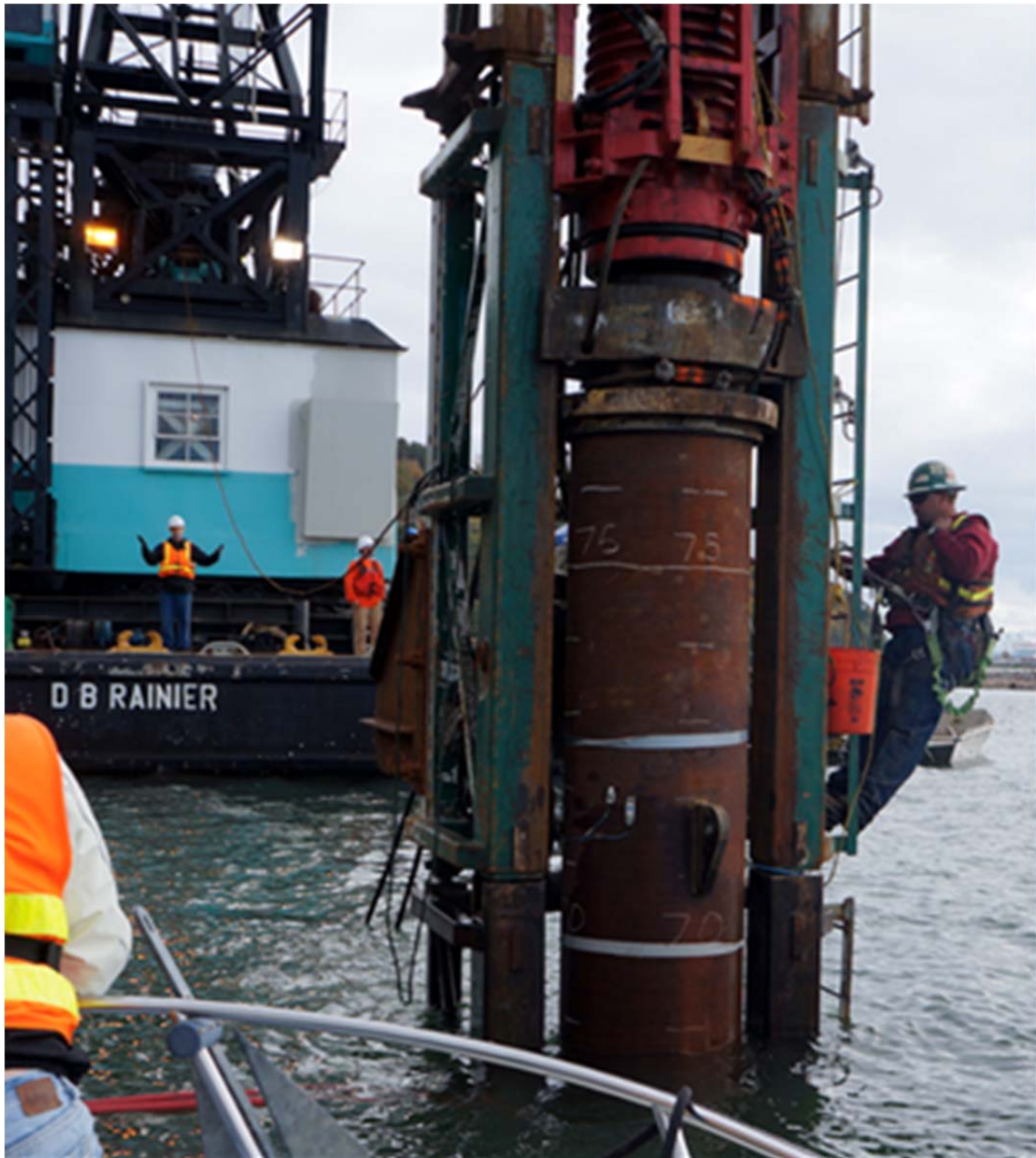
Figure 11: Delmag D46 Impact hammer being set to the control pile
