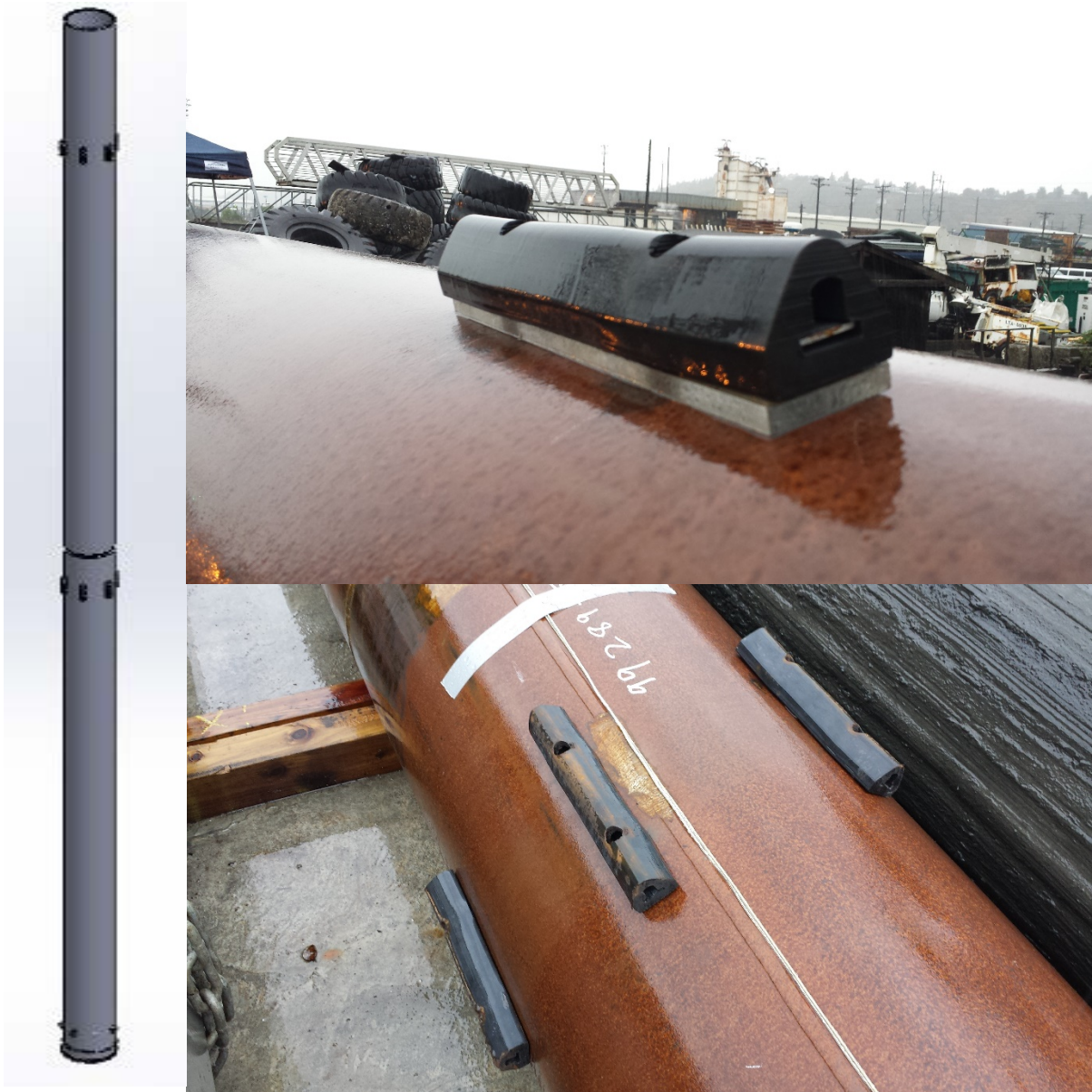
Figure 16: Installation of pile spacers
