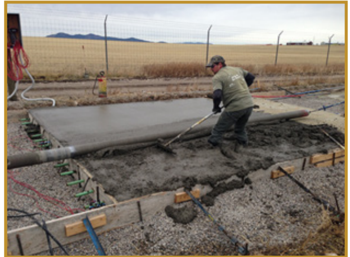
Figure 4: Casting Field Demonstration Slabs During Phase 2
