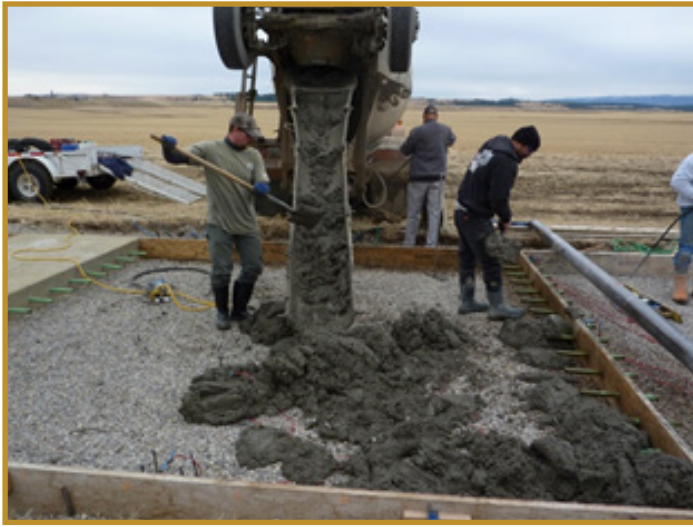
Figure 4: Casting Field Demonstration Slabs During Phase 2
