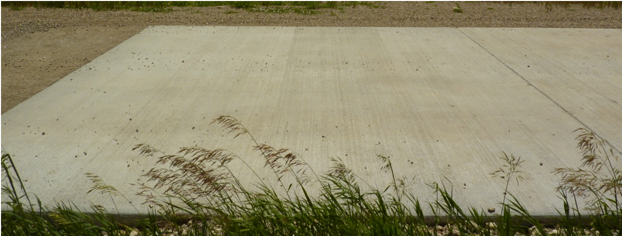
Figure 12: HR Slab at Two Years
