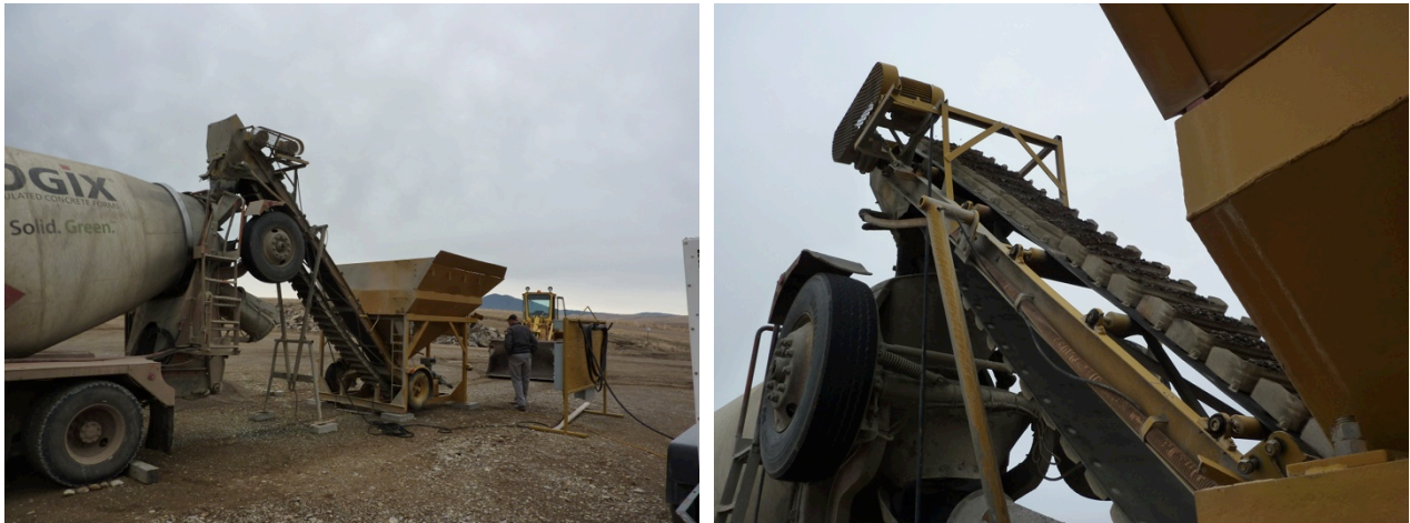
Figure 8: Charging concrete truck with RAP aggregate
