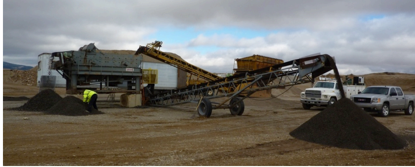
Figure 5: Overview of RAP processing
