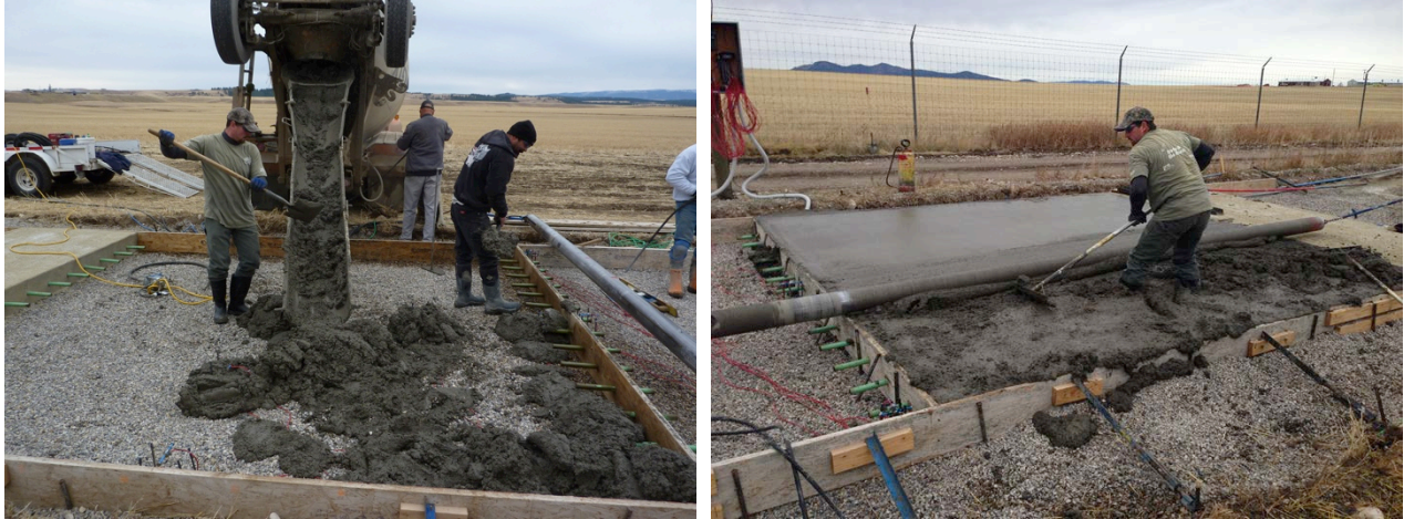
Figure 9: Placing and finishing a RAP slab
