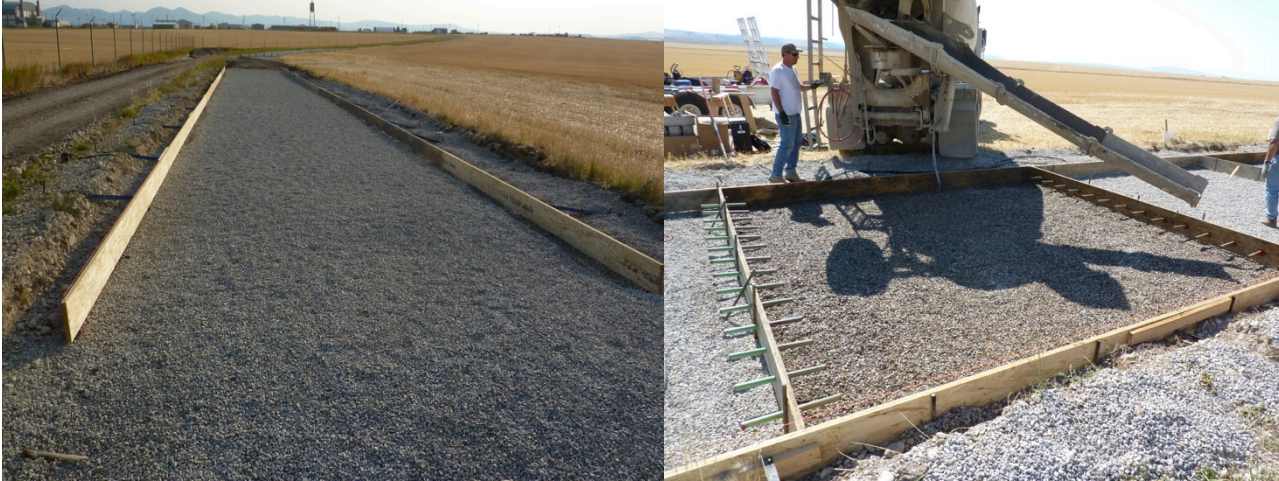
Figure 2: Base course and formwork
