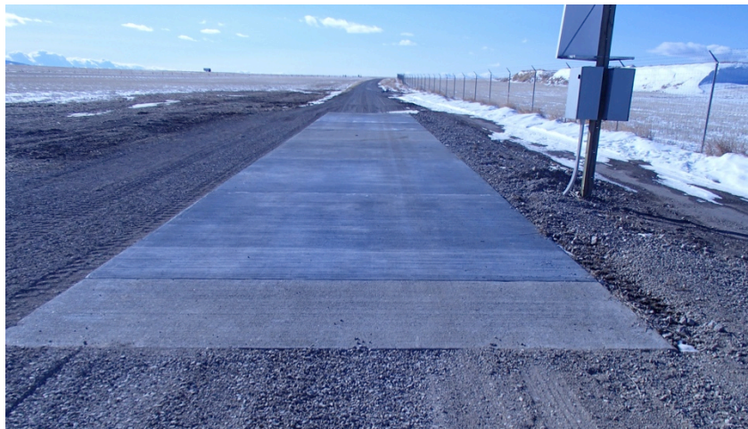
Figure 10: Finished test slabs
