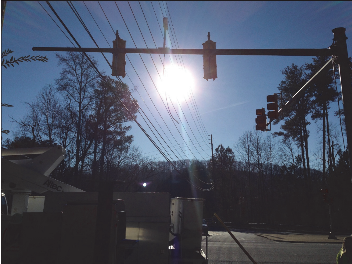
Figure 5.7 Potential glare issue in the morning of a sunny and clear day (site 2)
