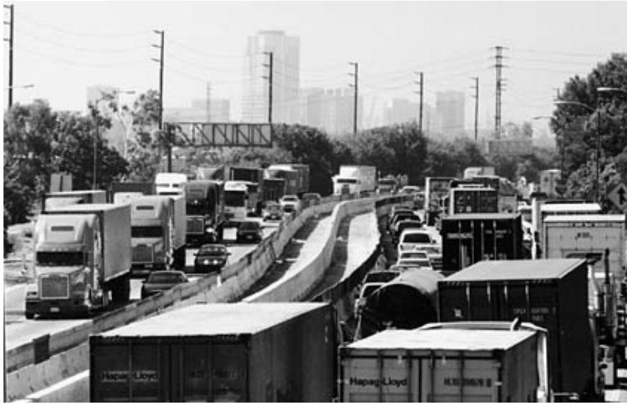
Figure 1.2: Trucks Dominate 710 Freeway on a Morning Commute
