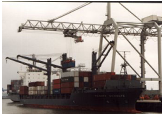
Figure 2.4: Wharf Crane at the Port of Rotterdam, the Netherlands
