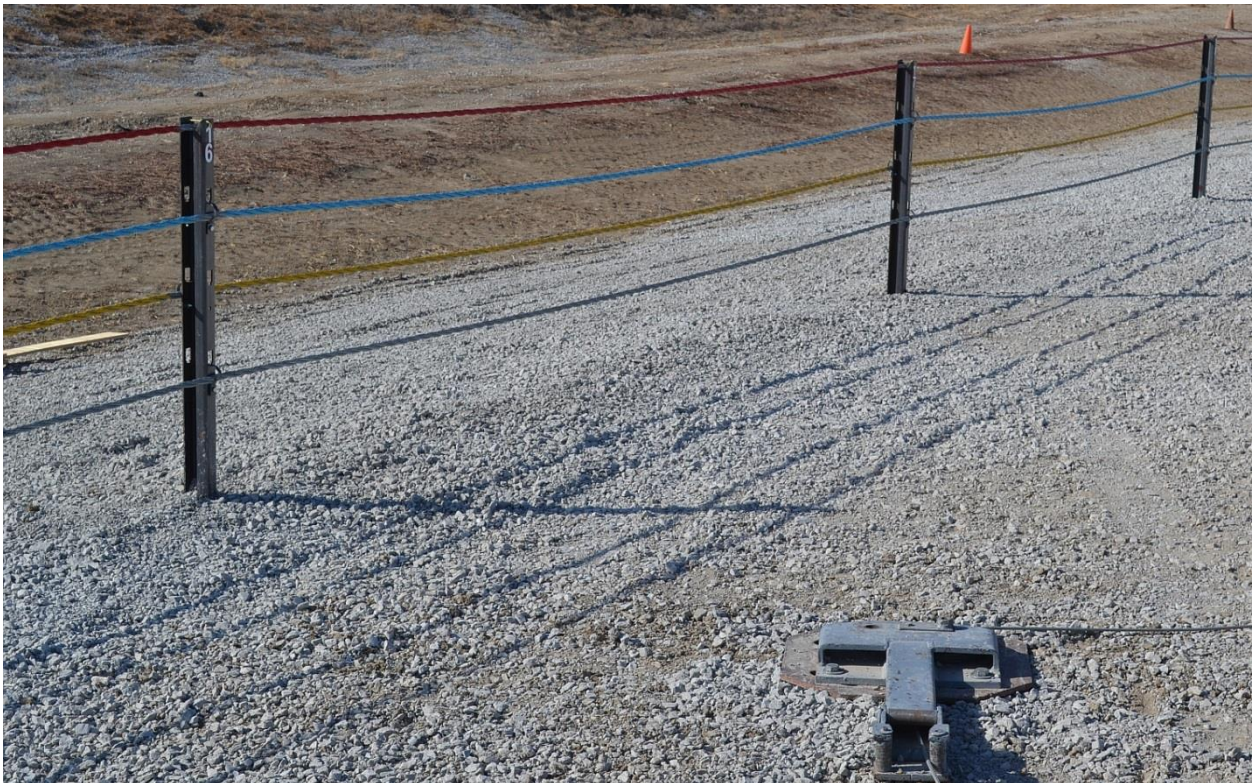
Figure 38. Test Installation Photographs, Test No. MWP-1
