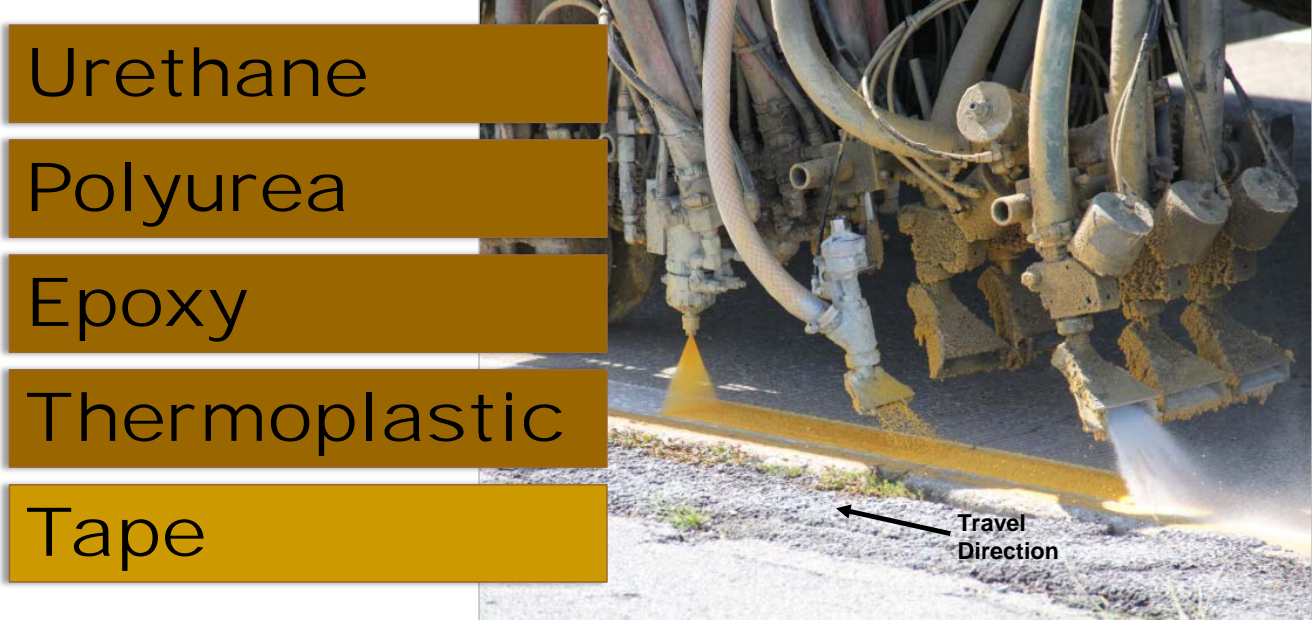
The wet reflective media were delivered to the line prior to the standard IDOT beads, as shown in the photo above. All liquid marking products were placed within a 60 mil groove with the exception of thermoplastic which was installed within a 125 mil groove. The liquid pavement marking products were placed on several types of roadway surfaces (PCC and ACC).
