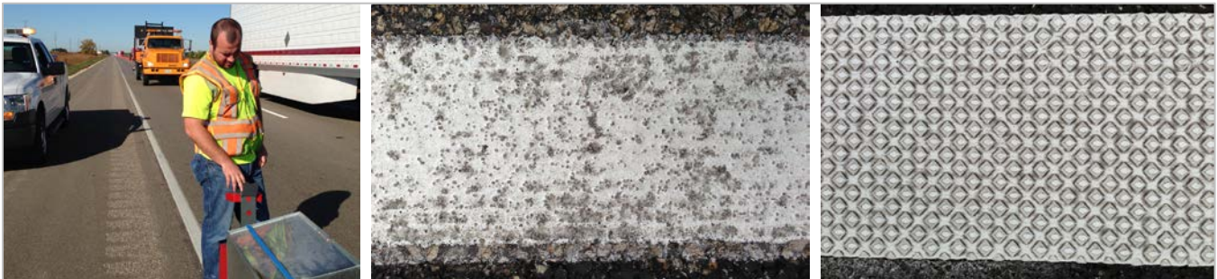
Figure 3.1 Taking a retroreflectivity (continuous wetting, left) reading on I-80 along with marking presence images for the white edge line (center) and centerline skip (right).
