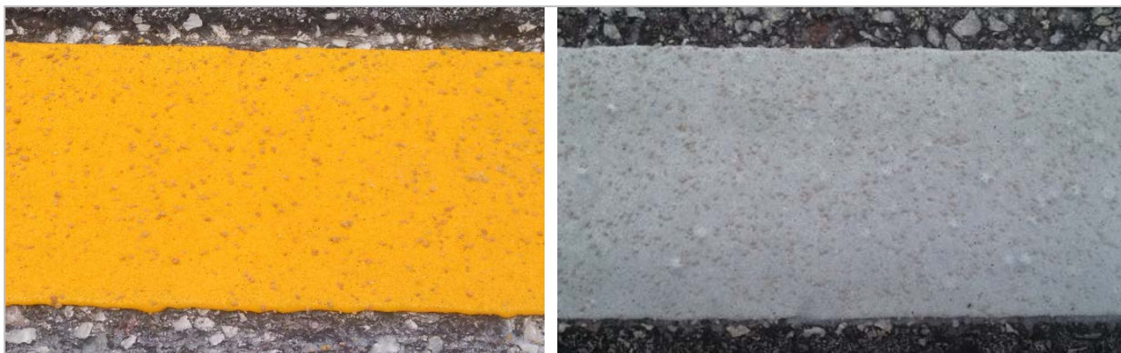
Figure 3.4 Initial installation images on I-57 for yellow edge line (left) and white edge line (right).
