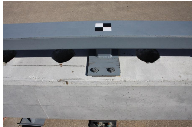
Second Connection Downstream from Joint No. 6/7
