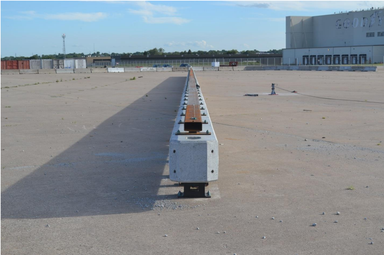
Figure 26. Test Installation Photographs, Test Nos. SFH-1 through SFH-2
