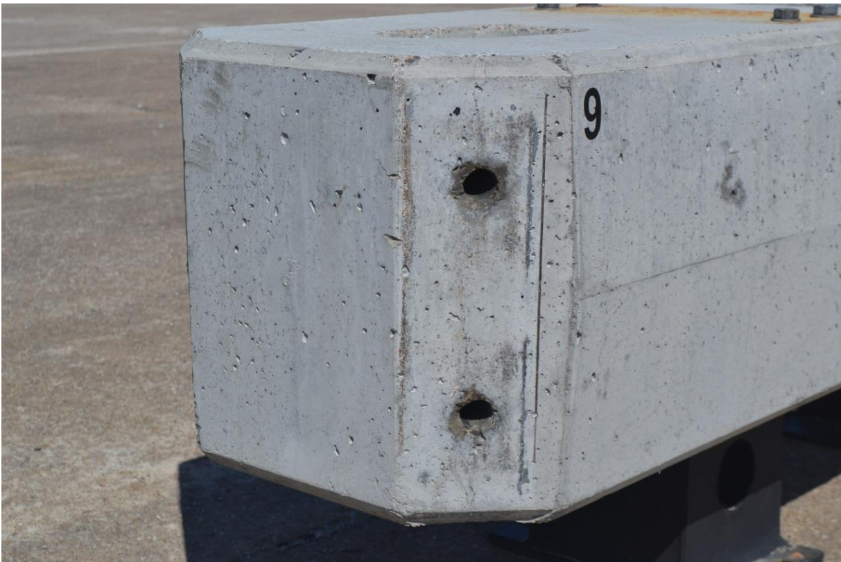
Upstream Barrier No. 9
