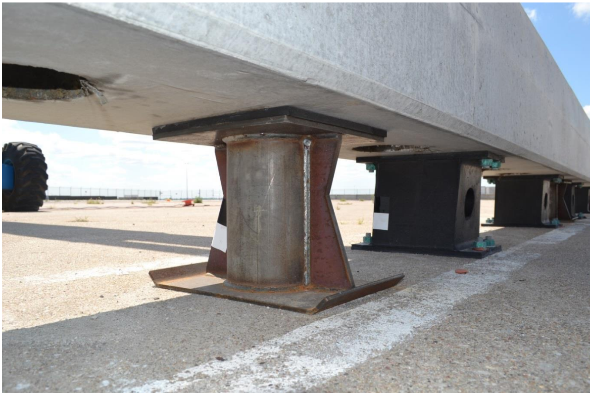
Figure 28. Test Installation Photographs, Skids and Upper Tube Assembly Splices, Test Nos. SFH-1 through SFH-2
