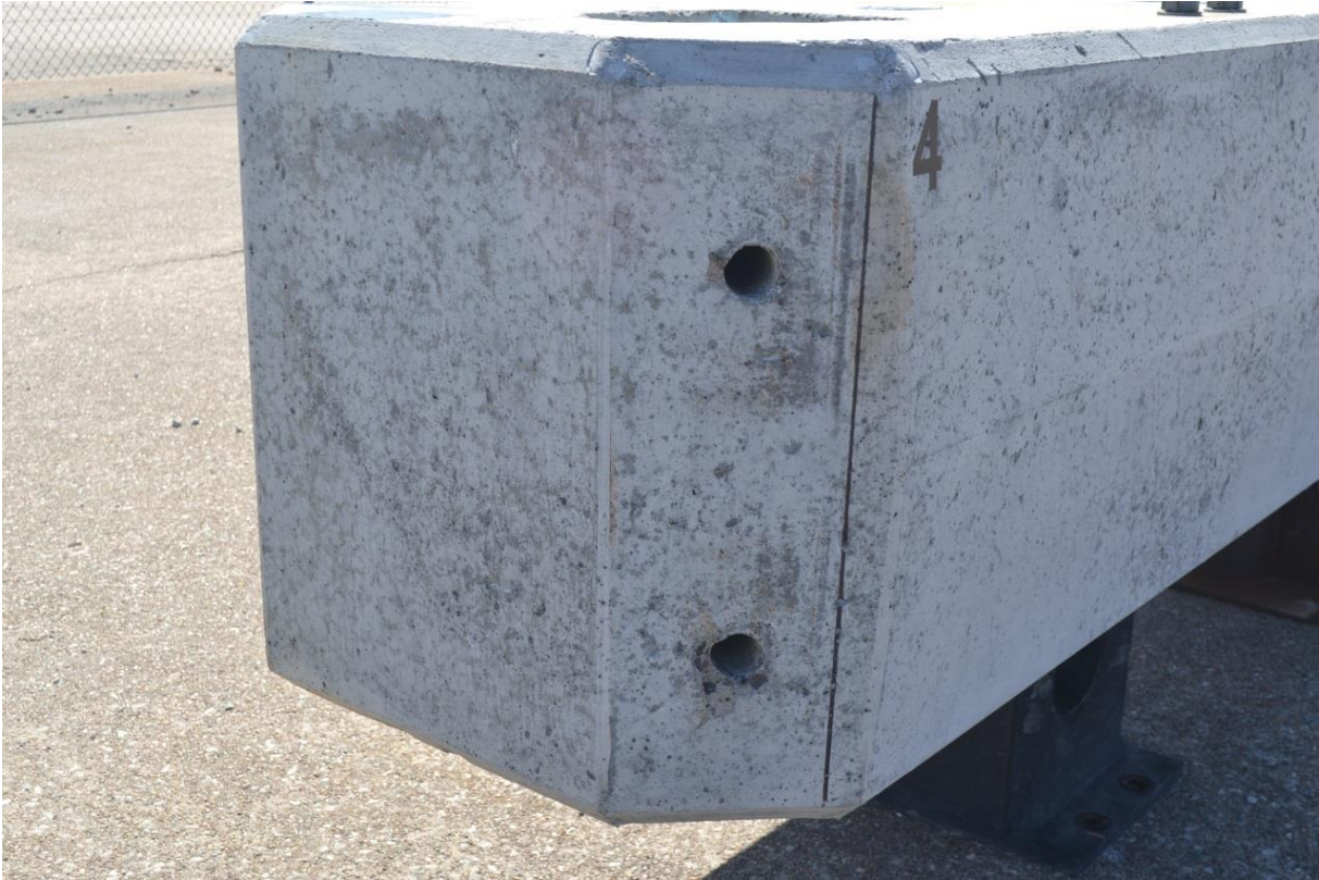
Downstream Barrier No. 4
