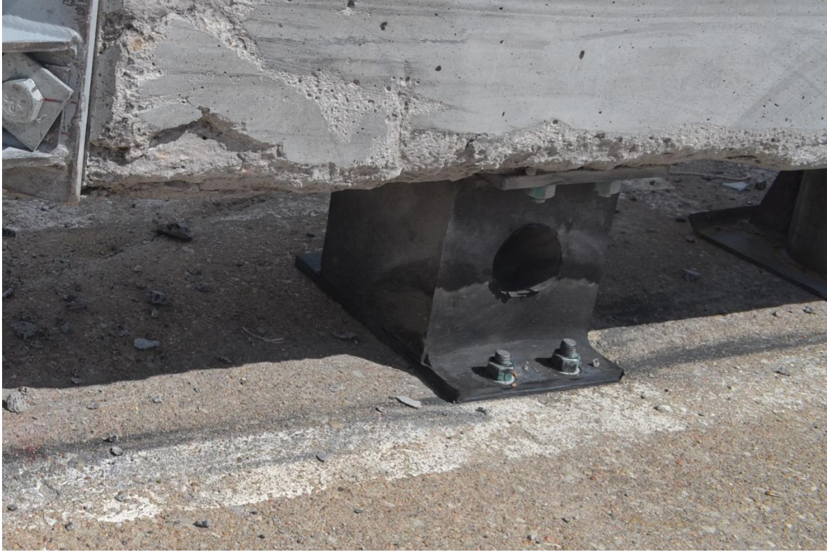
First Post Downstream from Barrier Nos. 5 and 6 Joint
