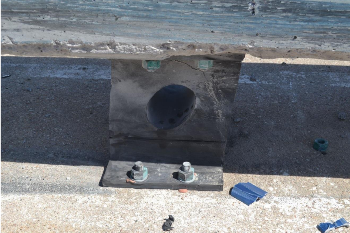
a) First Post Downstream from Joint between Barrier Nos. 7 and 8
