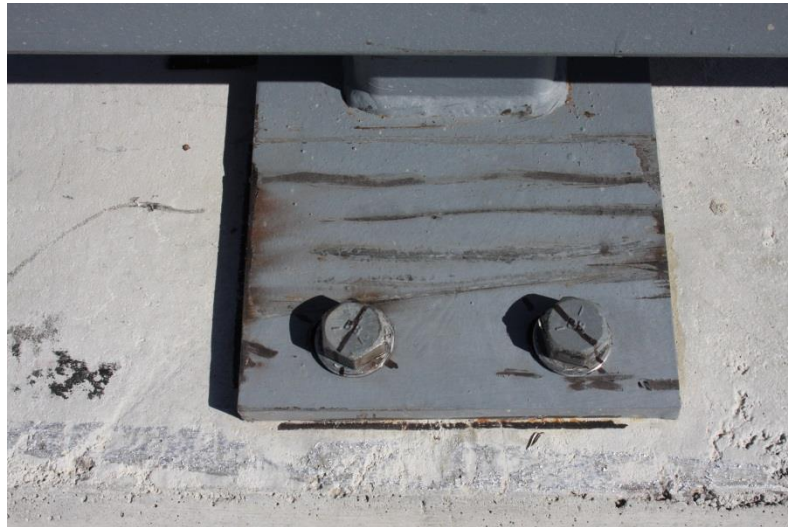
First Connection Downstream from Joint No. 6/7
