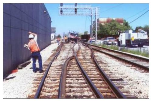
Figure 5. Switch Where the Derailment Initiated
