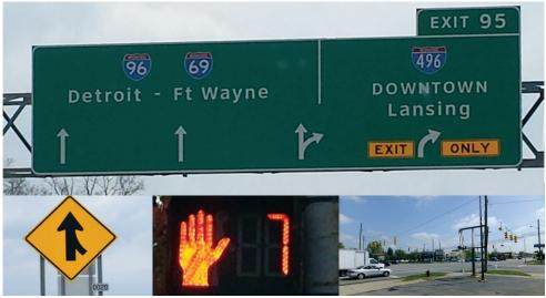
Improvements intended to improve safety for older drivers include (top) signage with the Clearview font and arrow-per-lane signing and (from bottom left) fluorescent yellow sheeting, pedestrian count-down signals and box-span signal configuration.
