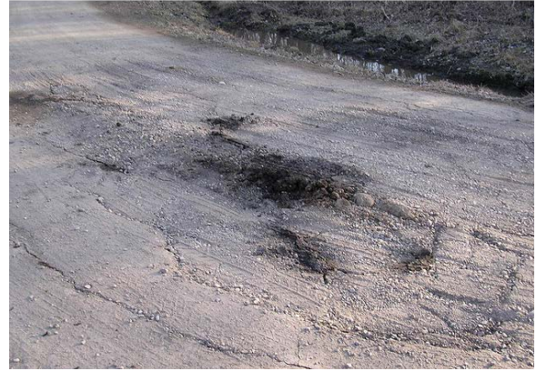
Figure 2. Boils in a gravel road.
