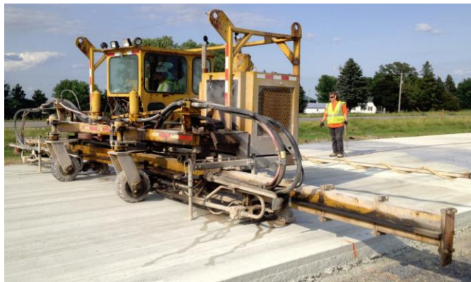
Figure 9. A non-typical conventional saw machine used at Site B
