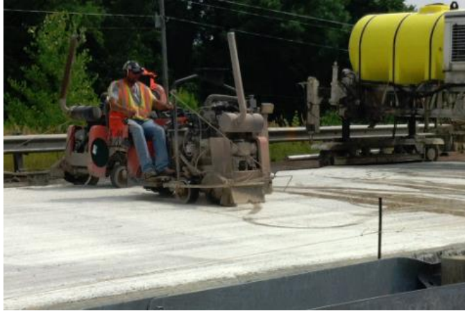
Figure 8. A typical conventional saw-cutting process
