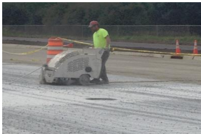
Figure 7. A typical early entry saw-cutting process
