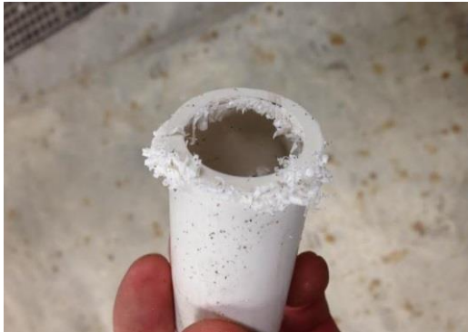
Figure 31: Bur on PVC pipe
