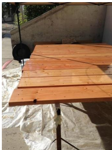
Figure 33: Planks drying after sealing
