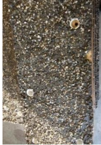
Figure 37: Chip in plank. Figure 38: Chip patched. Figure 39: Additional chip patched.
