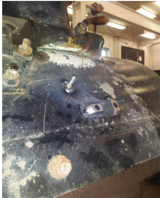
Figure 24. Strain gauges installed on the back of the underbody scraper.
