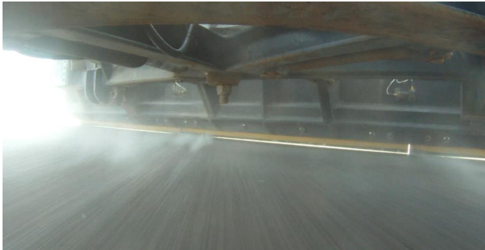
Figure 36. Carbide insert blade on asphalt pavement.
