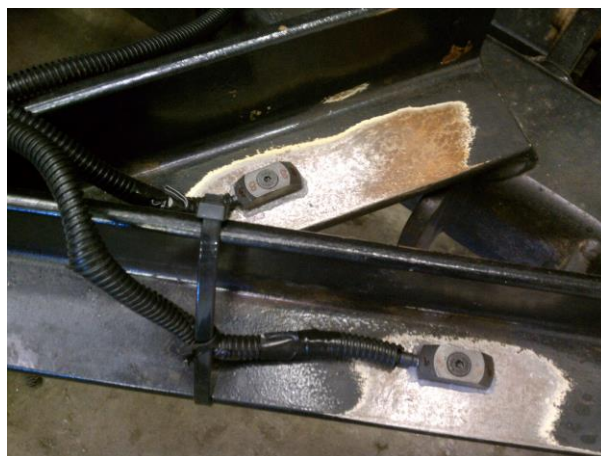
Figure 18. Member preparation and strain gauge installation.
