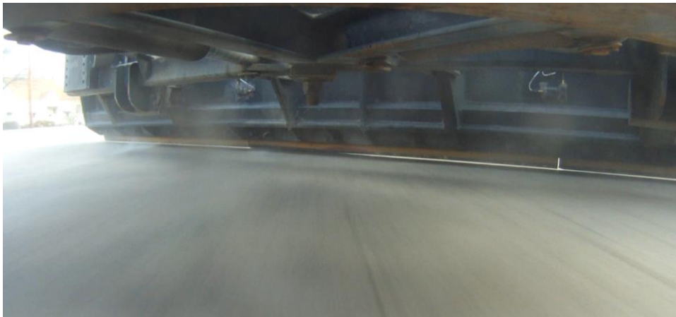
Figure 37. Carbide insert blade on concrete pavement.
