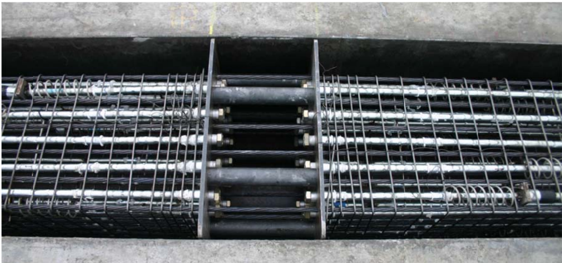
Figure 5.9. Splicing system in place.
