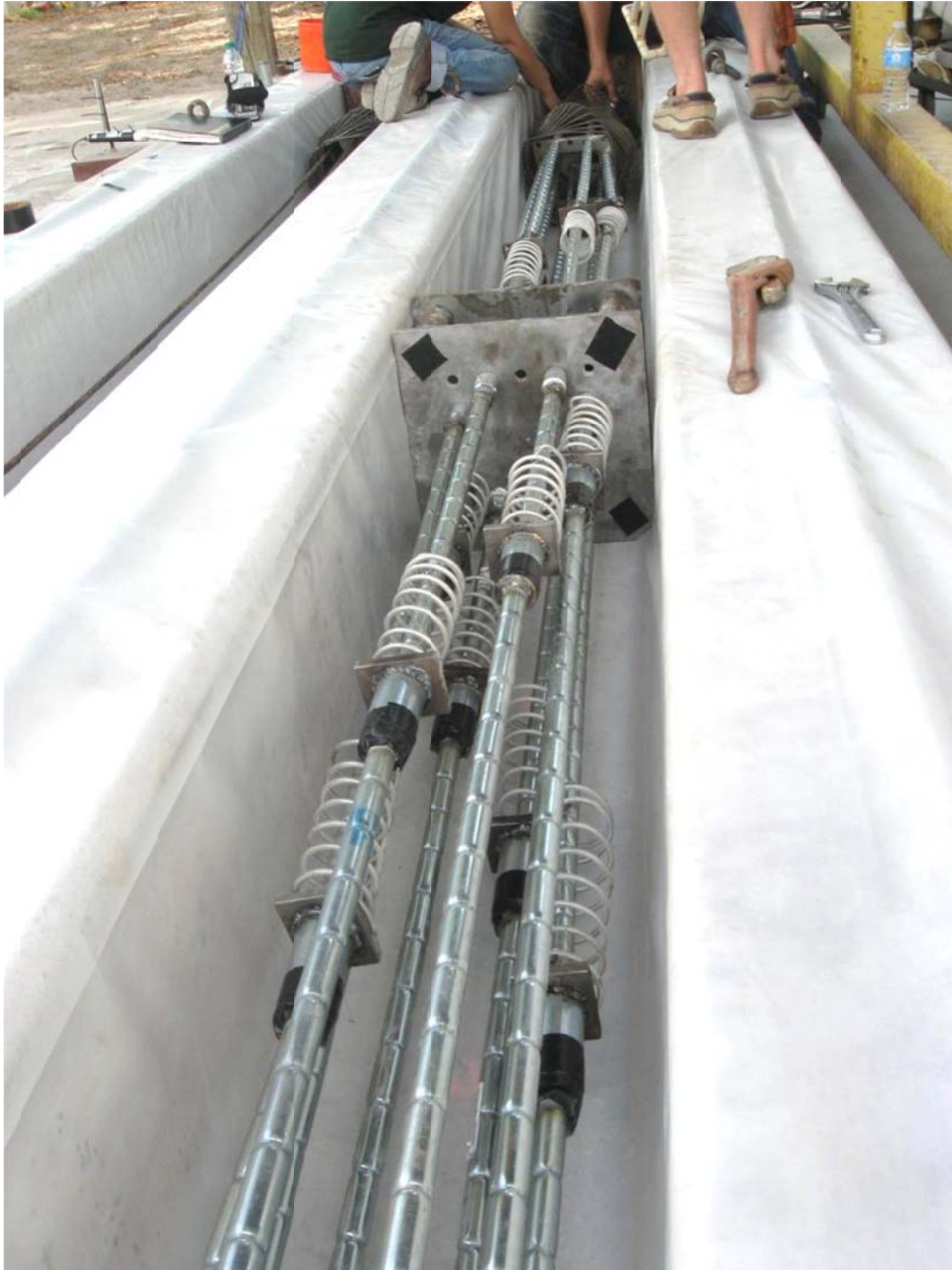
Figure 4.67 Assembly prior to pulling strand and spirals (looking toward lower segment).
