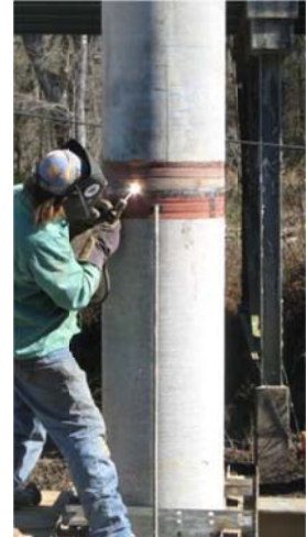
Figure 2.2. Welded pile splice
