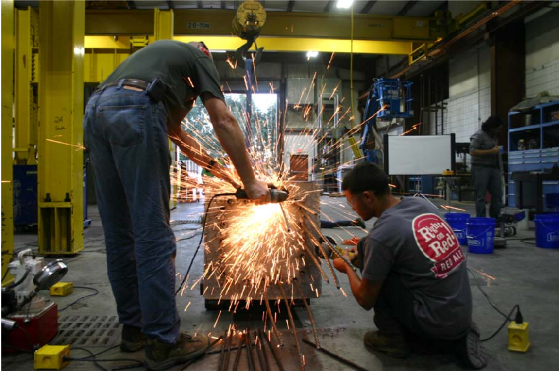
Figure 5.22. Cutting excess strand length before attaching grout fittings.
