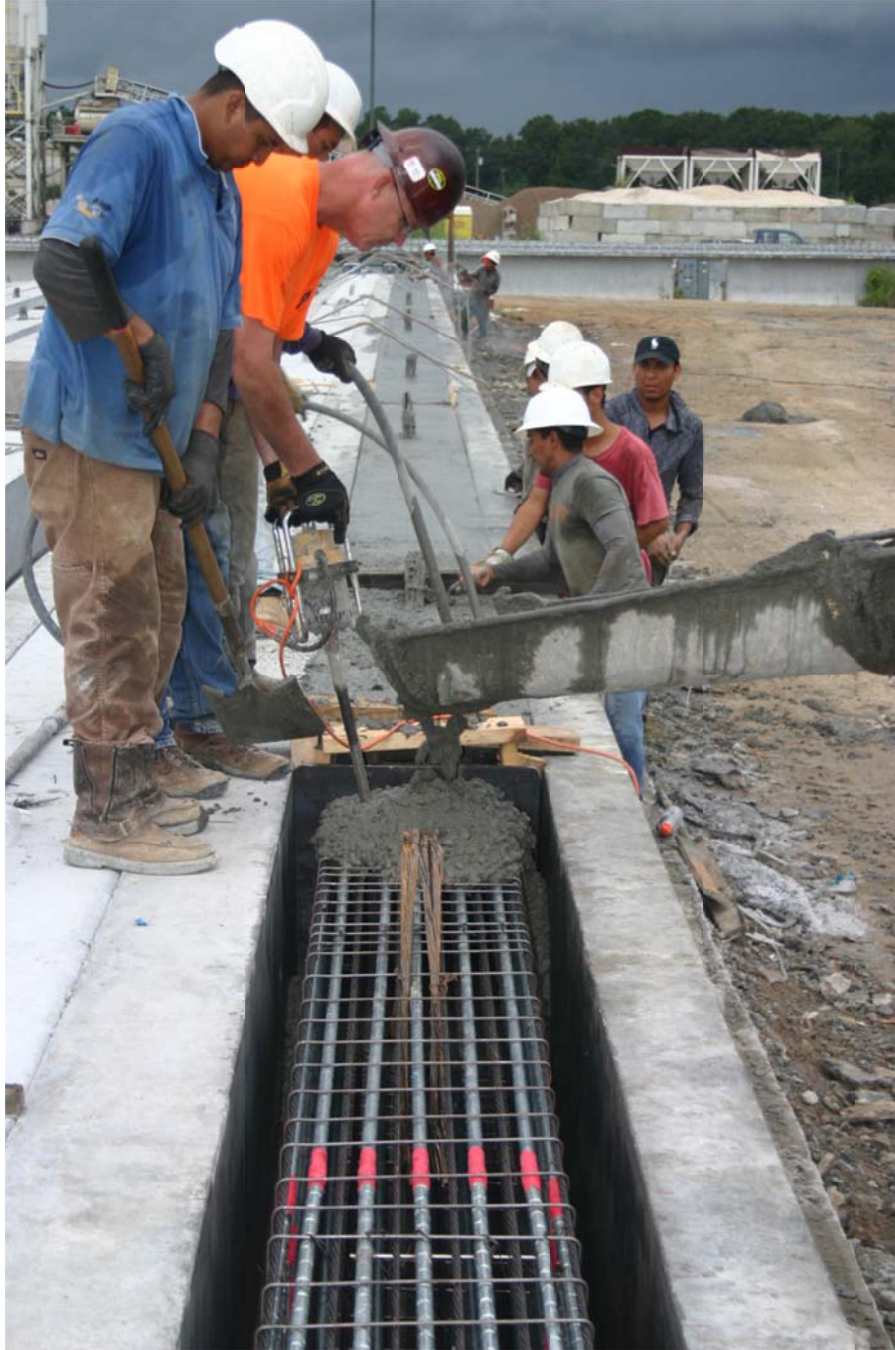
Figure 5.13. Concrete placement.
