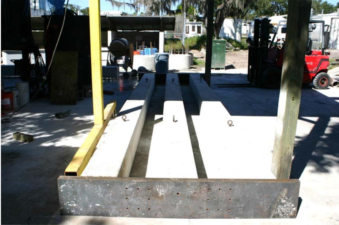
Figure 4.12. Drilled header plates in place.
