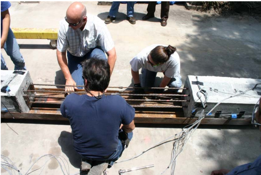
Figure 4.97. All strands inserted. Flexibility of the 8 ft strands allows additional options to insert strands at will even if all strands were encountered at the same time. However, staggering also meant that no two anchorages were encountered at the same time.
