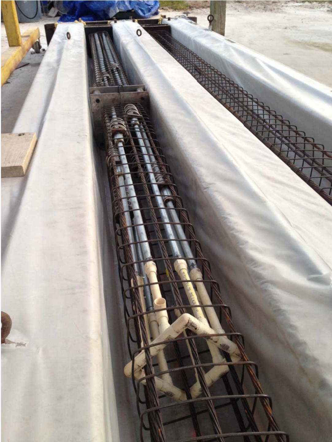
Figure 4.27. Grouting manifold beneath lower pile embedded anchorages.
