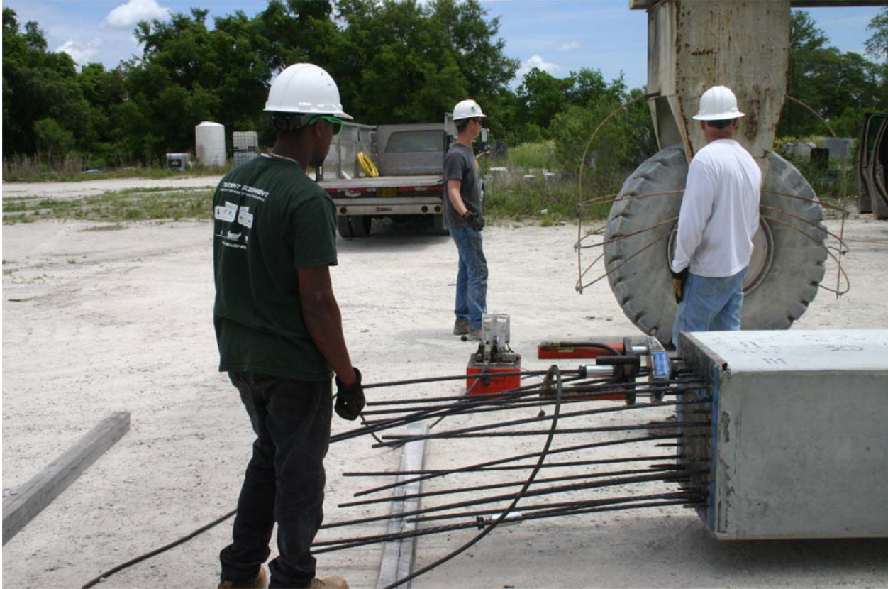
Figure 6.24. Post-tensioning of splicing strands.
