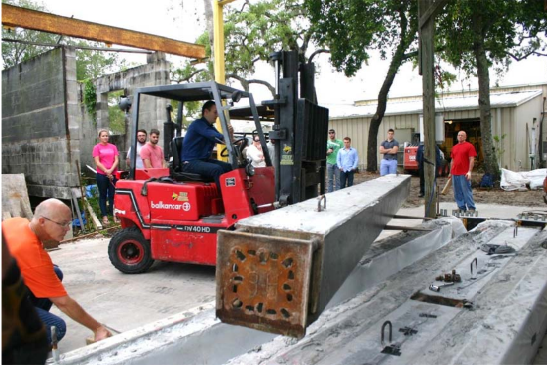
Figure 4.78. Control pile extracted from casting bed.
