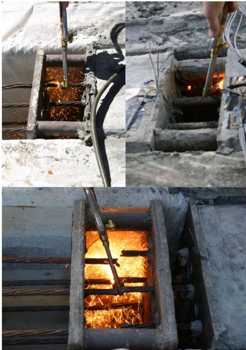
Figure 4.34. Strand cutting live end (TL), middle splice header (TR), and dead end (bot).
