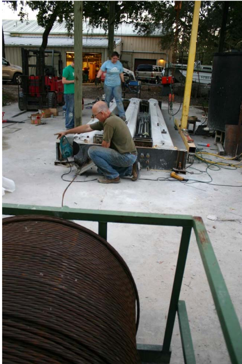
Figure 4.21. Threading strand into casting bed.
