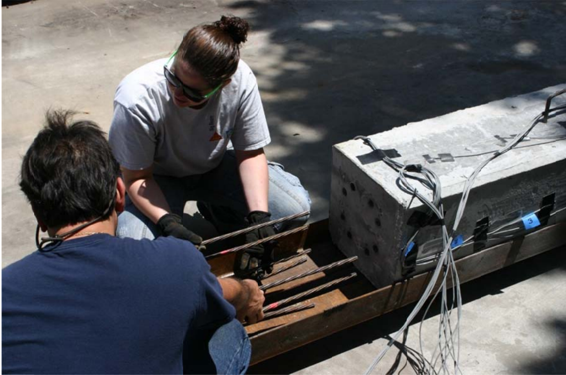
Figure 4.94. Aligning first of 8 strands as pile segments are pushed together.
