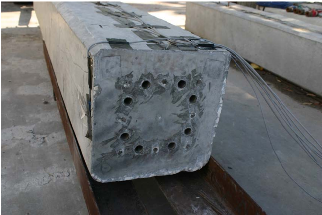
Figure 4.50. Lower pile segment aligned with upper segment on splicing rail.
