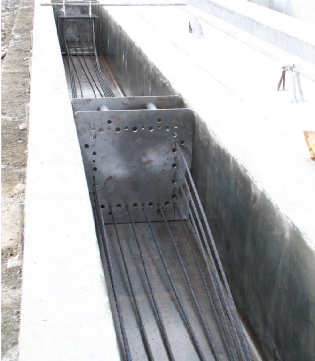
Figure 5.8. Strands threaded through header plates in casting bed.
