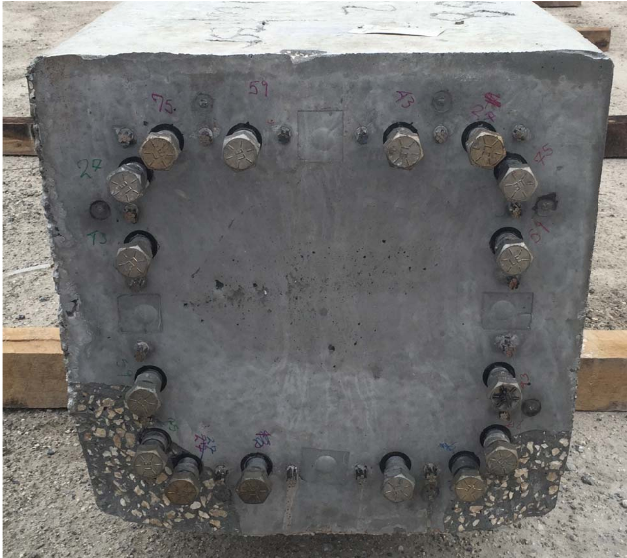
Figure 6.14. Upper pile splicing was face was chipped along bottom side during removal from bed (duct bolts retained to keep ducts clean and free from debris).
