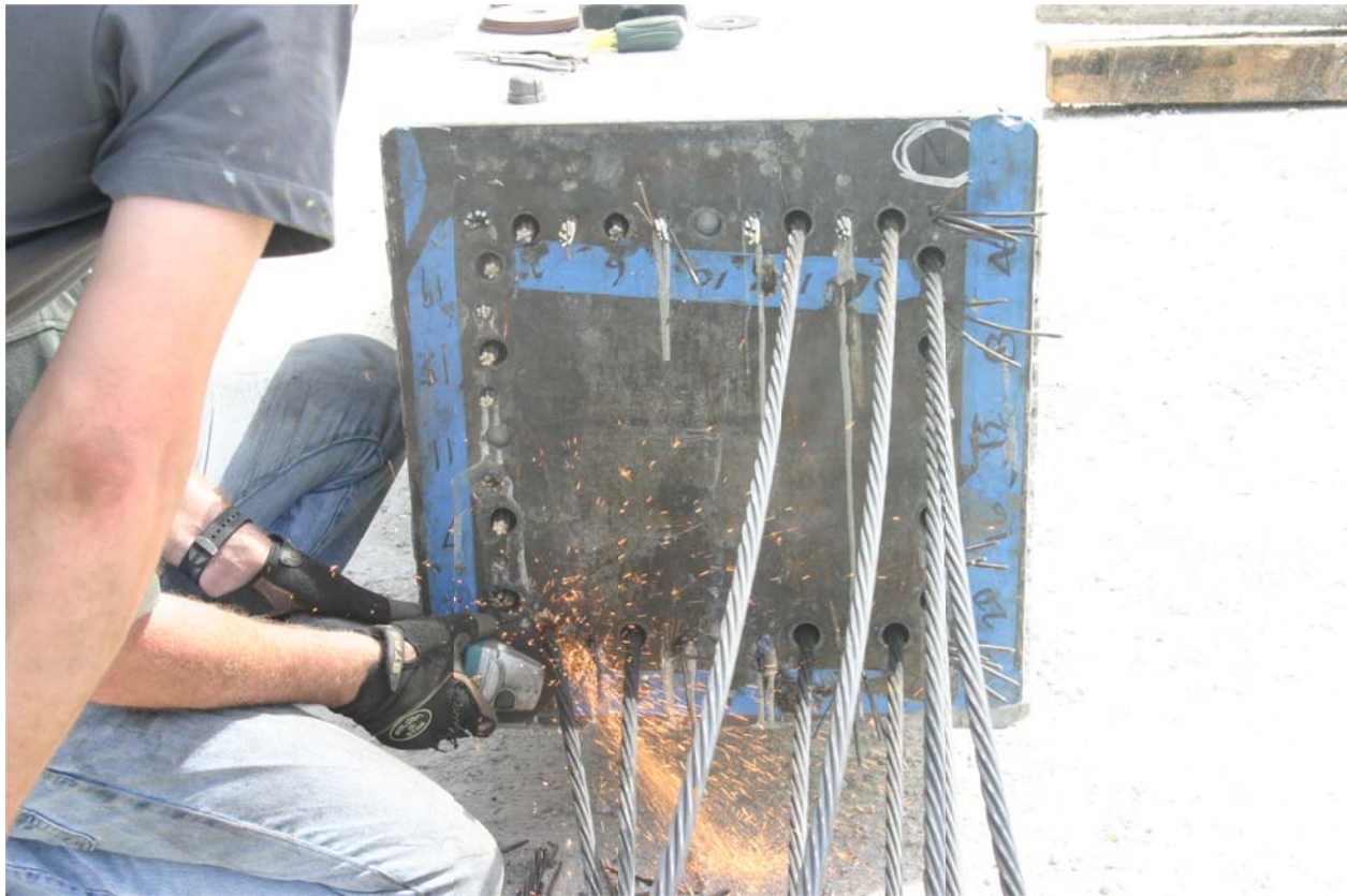
Figure 6.30. Cutting excess strand length before attaching grout fittings.
