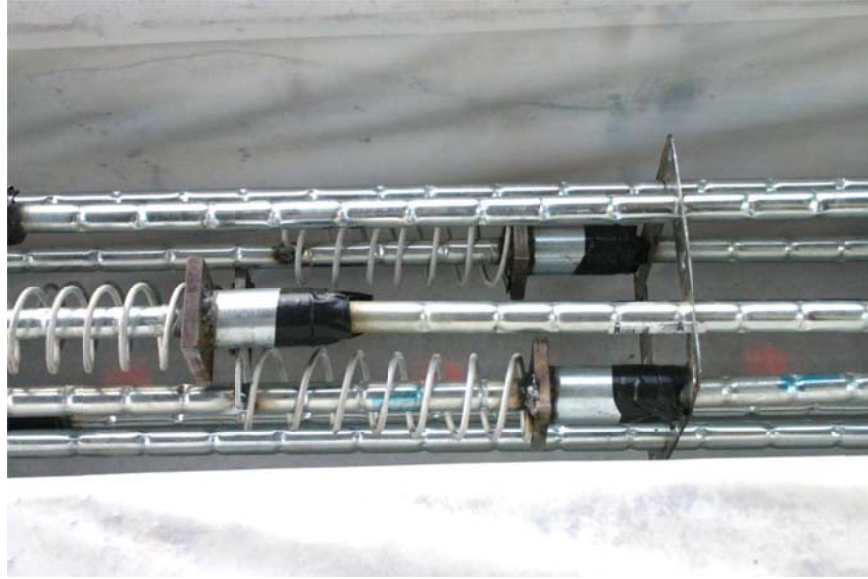
Figure 4.69. Alignment plate inserted into the lower and upper segment of the splice pile to better locate ducts.
