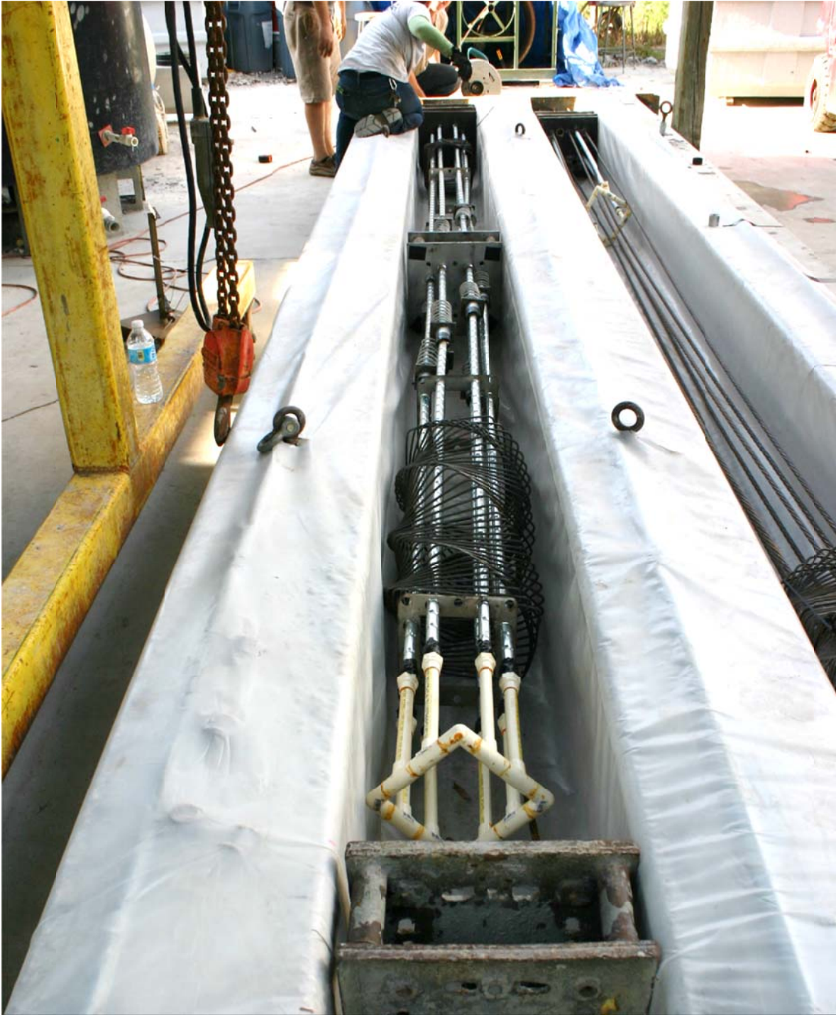
Figure 4.68. Assembly prior to pulling strand and spirals (looking toward upper segment).
