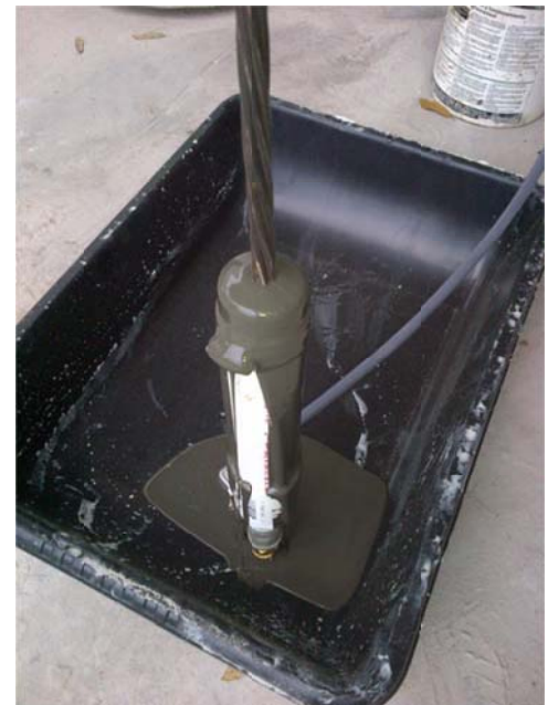
Figure 4.20. QPL approved grout pumped through chuck assembly.
