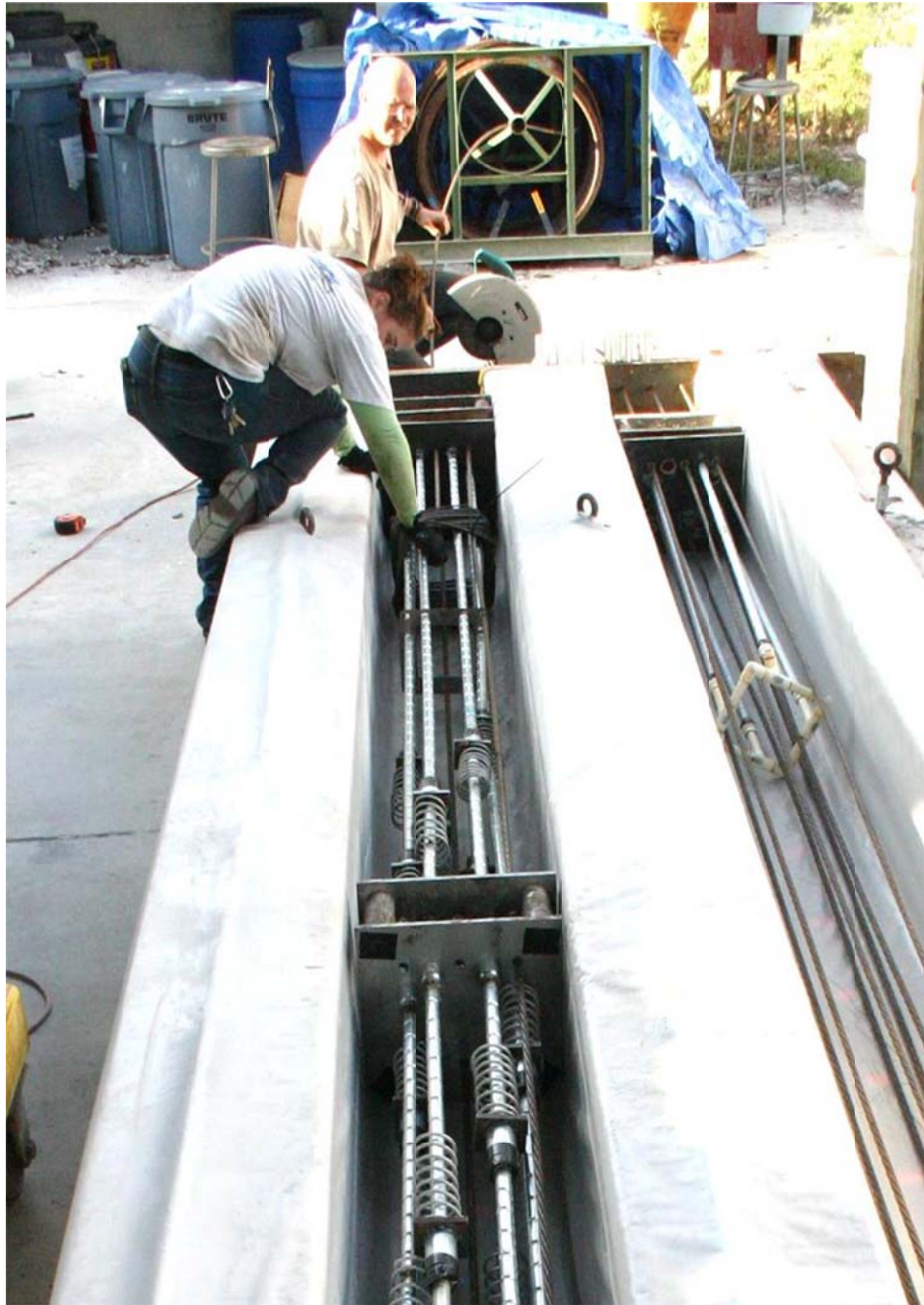
Figure 4.71. Threading strand into casting bed.
