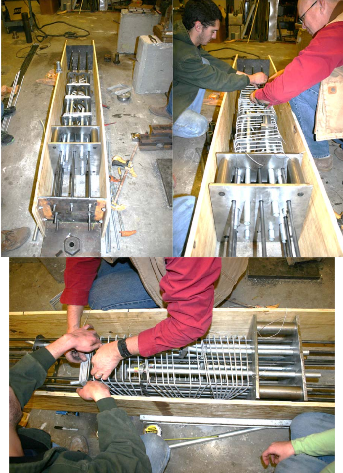
Figure 3.24. Mock assembly – components in place (left) and stirrups being tied (right & bottom).
