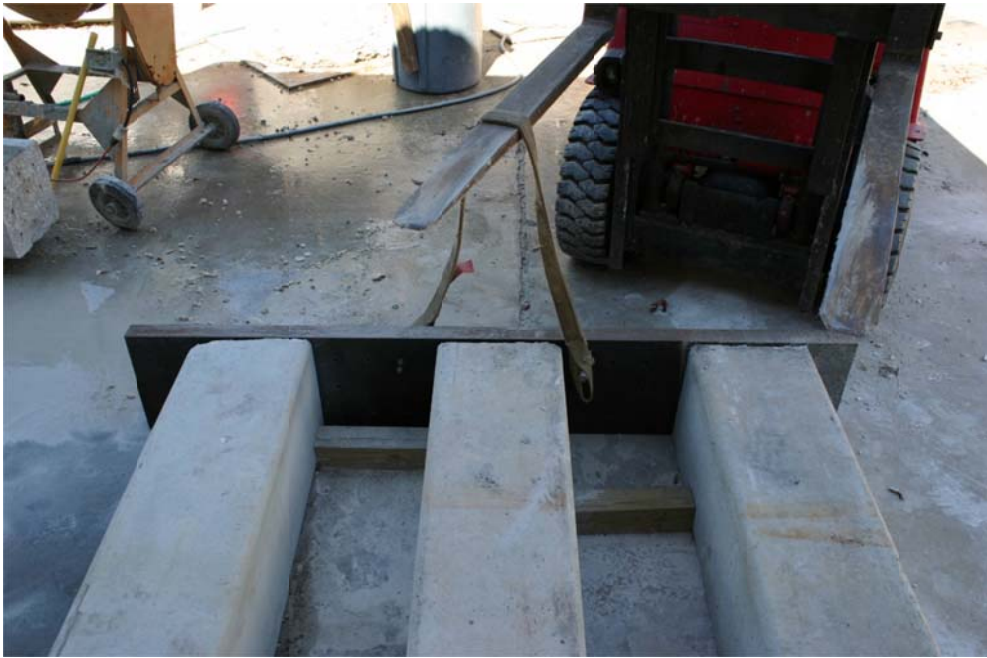
Figure 4.11. Placement of header plates at the ends of the casting beds.
