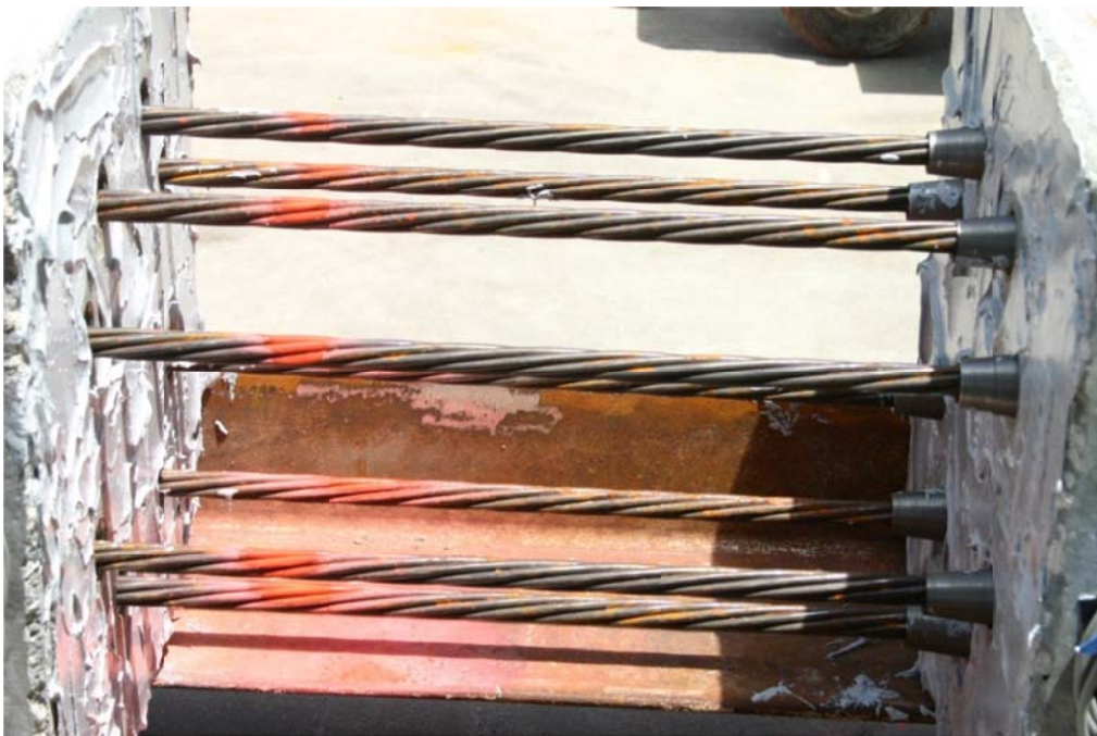
Figure 4.102. Strand clamps removed from upper segment (left), epoxy applied to both sides, ready for final assembly. Note no movement of strands into upper segment during assembly. The more restrictive wedge assemblies in upper segment (from double washer inserts) provide more resistance to sliding and therefore all movement from this point forward is into the lower pile segment (to the right).
