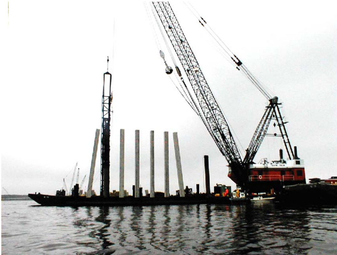
Figure 1.1. Thirty inch square solid prestressed piles driven into a bridge bent layout.
