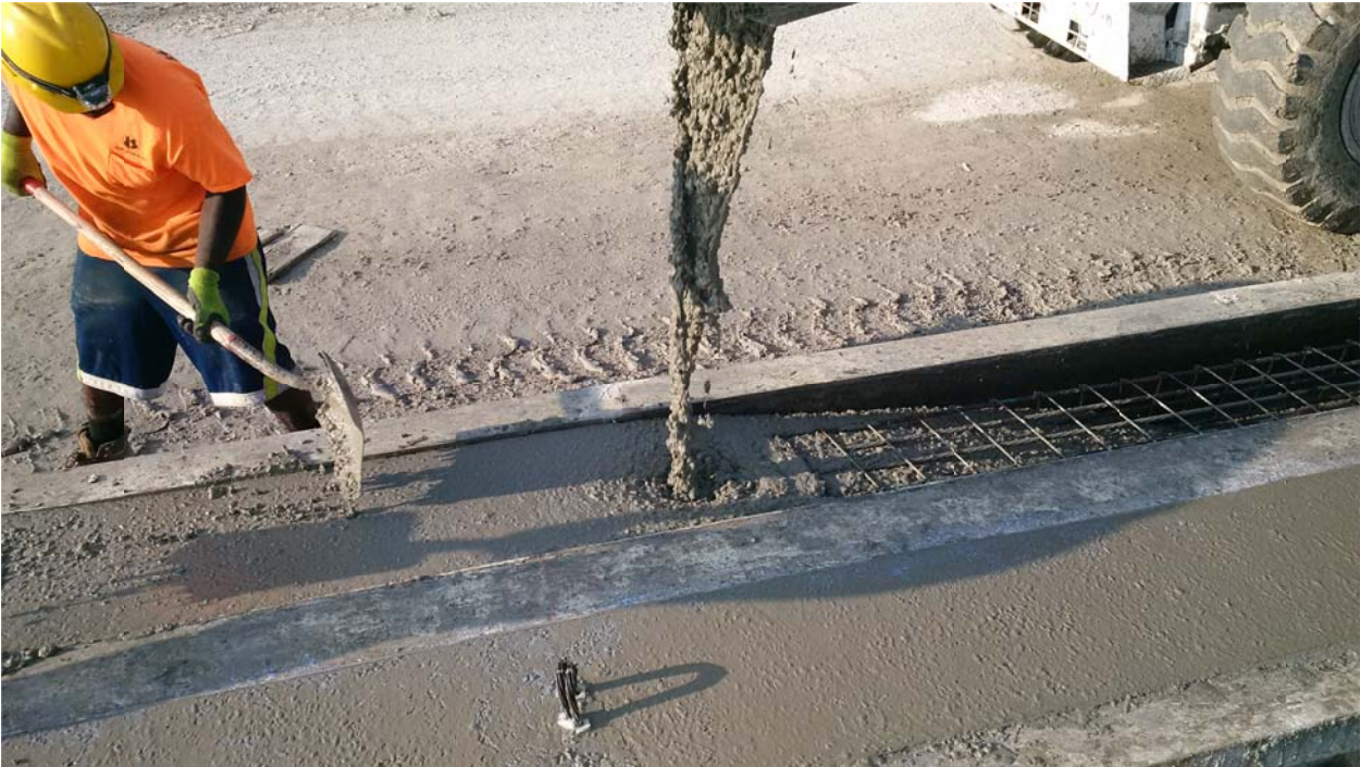
Figure 6.13. Concrete placement.
