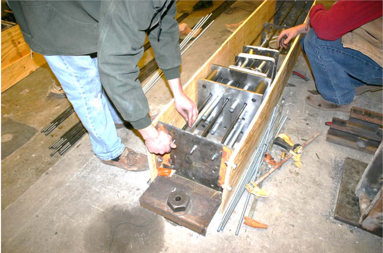
Figure 3.23. Mock casting bed assembly – placement of components.
