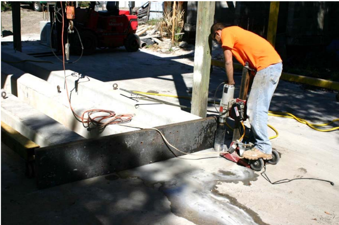
Figure 4.13. Coring slab to install ground anchors for header plates.
