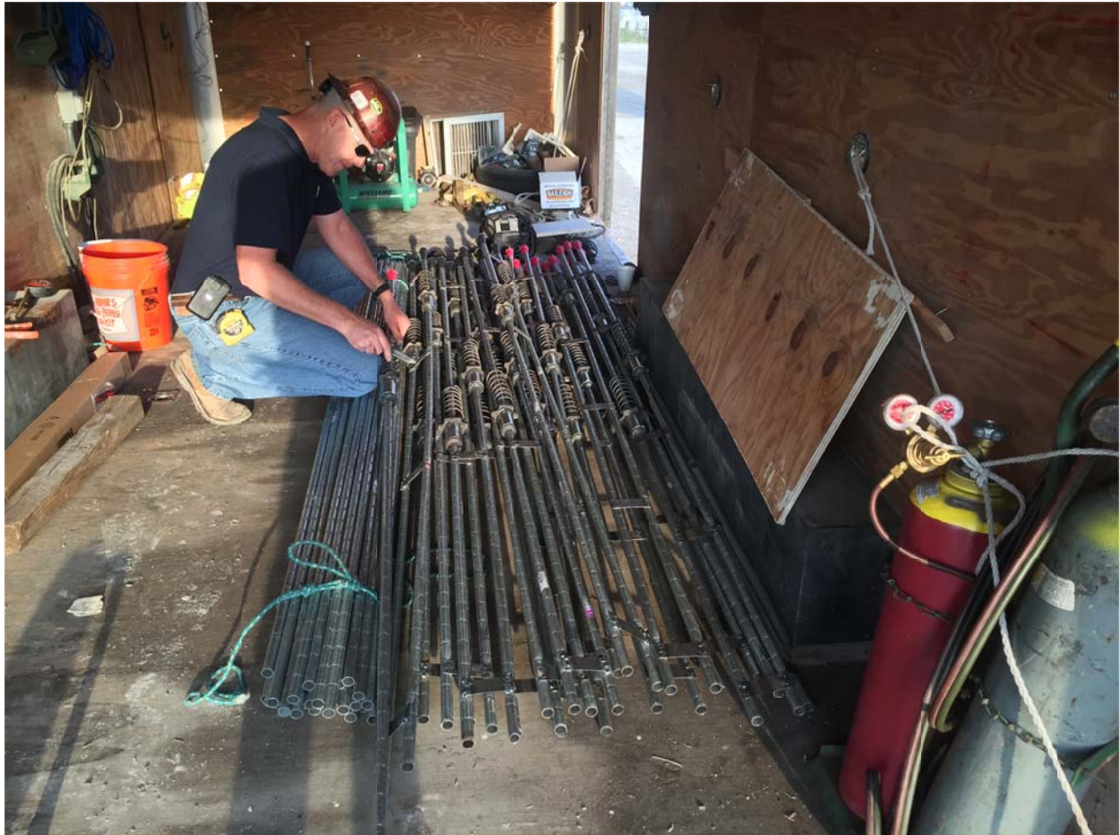
Figure 6.6. Internal components of splicing system as delivered to casting yard; extension ducts (left), paired anchorages (right).
