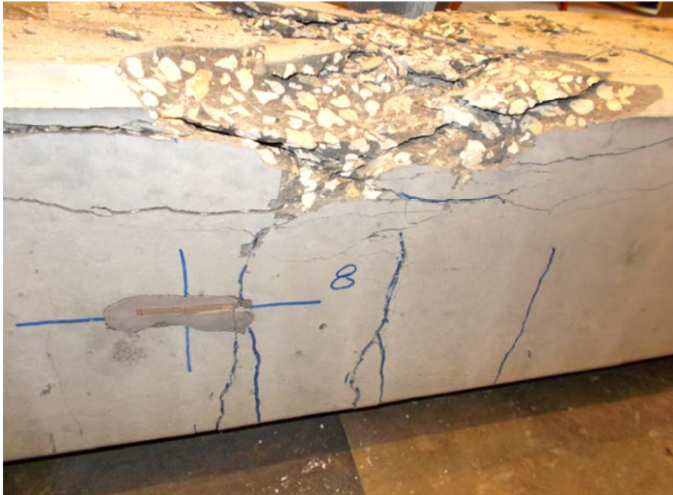
Figure 4.118. Specimen failure pattern (Control Pile 1 also shown in Figure 4.114)
