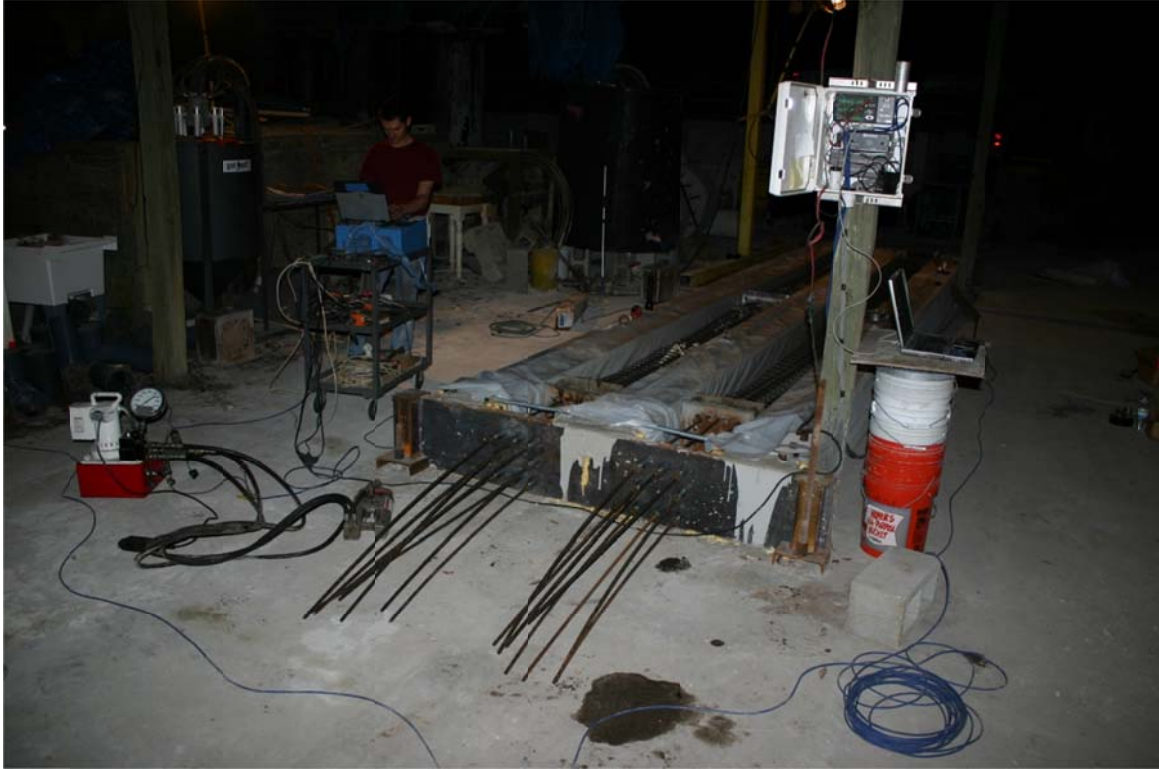
Figure 4.23. Live end prior to jacking.
