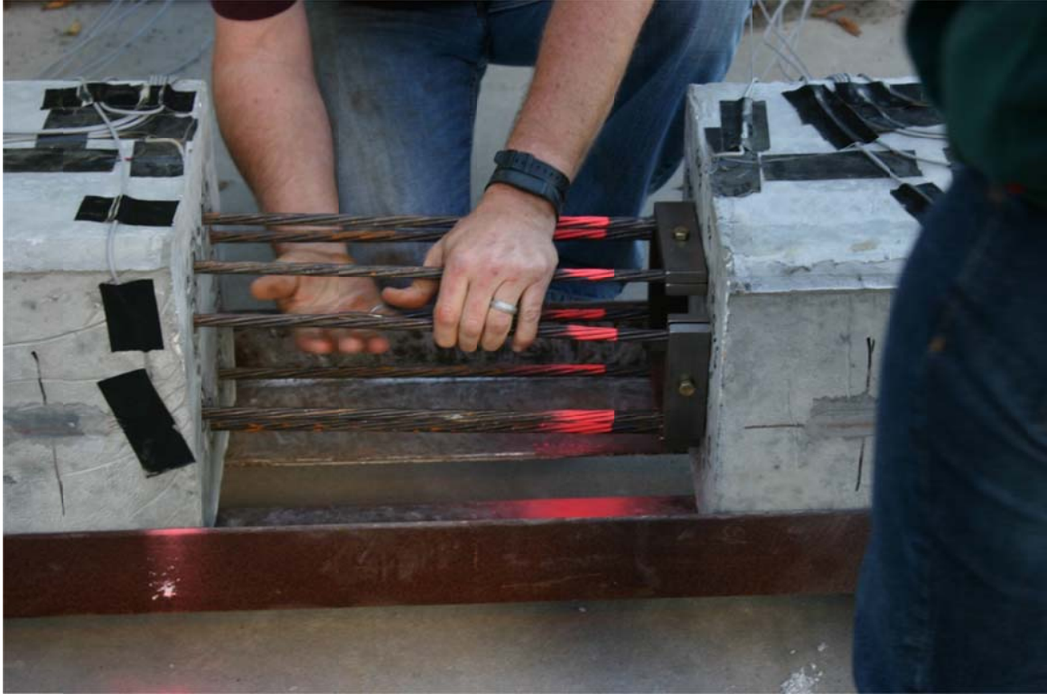
Figure 4.56. With all strands in, strand clamps need to be removed (upper segment right).
