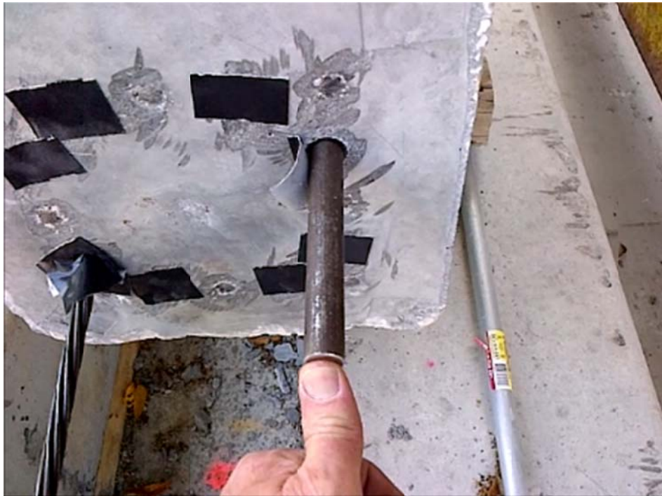
Figure 4.44. 48in long \frac{3}{4} in diameter rod used to check anchorages by compressing wedge assembly spring.
