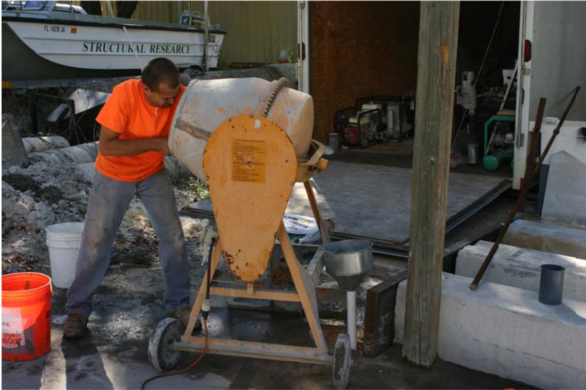
Figure 4.14. Mixing mortar for ground anchors.
