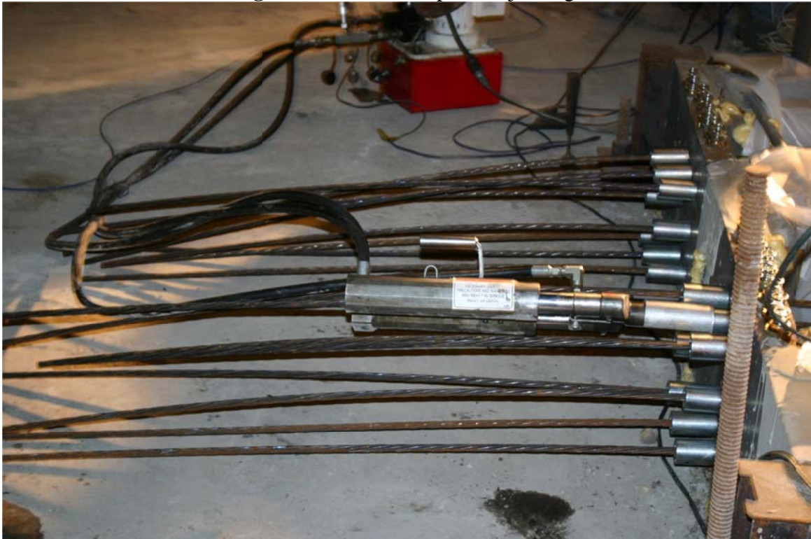
Figure 4.24. Stressing jack engaged.
