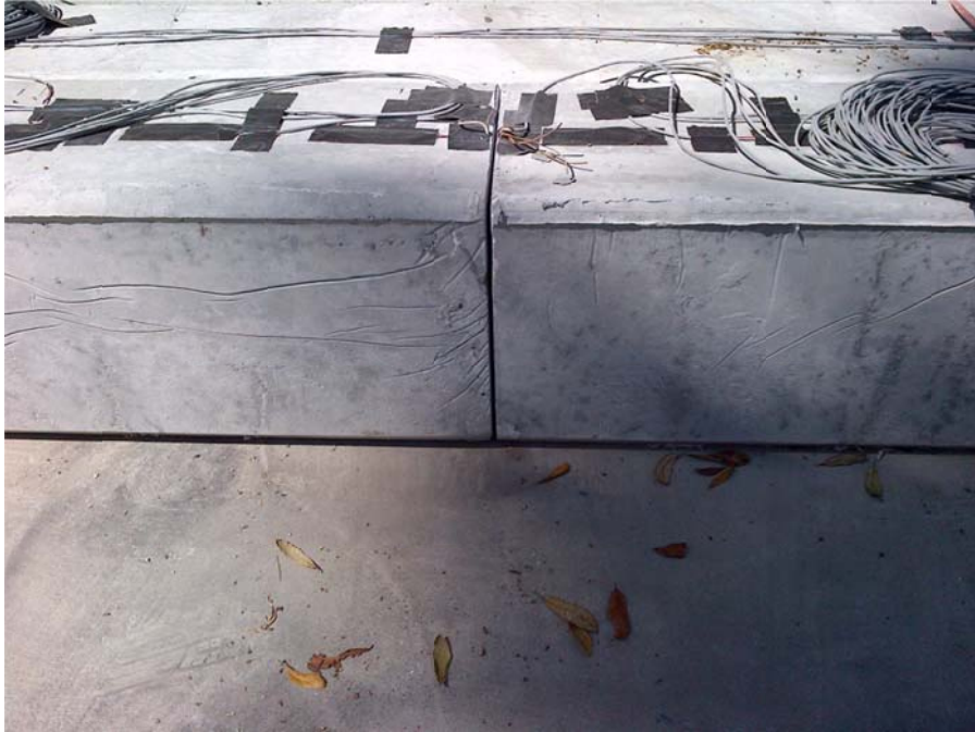
Figure 4.43. Mated ends of splice after grinding off strand and duct stubs.
