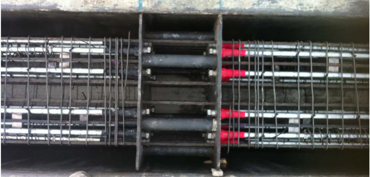
Figure 6.10. Splicing system in place
