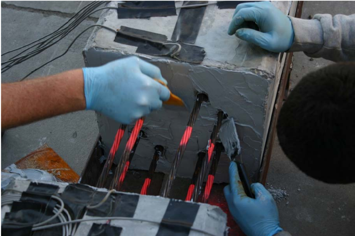
Figure 4.57. QPL-approved epoxy applied to both sides per manufacturer's recommendations.
