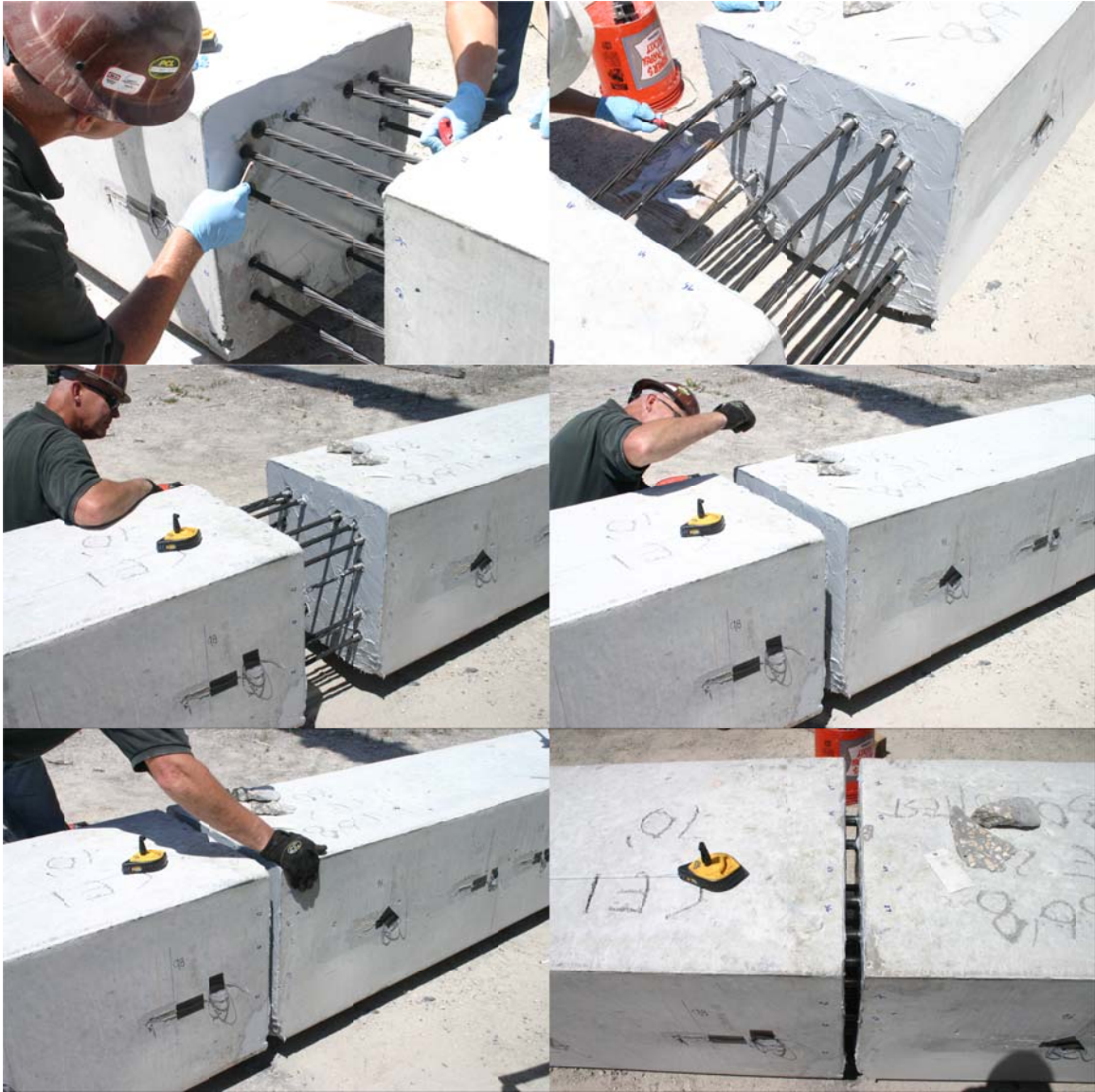
Figure 6.22. Final steps in aligning the splice.
