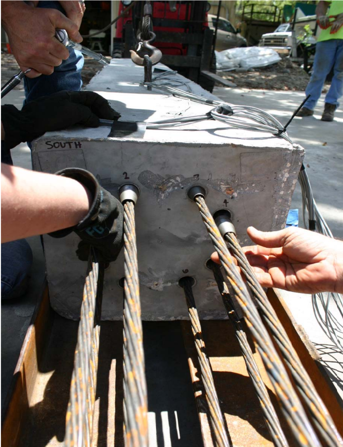
Figure 4.98. Installation of isolation sleeves into bottom pile segment duct ends
