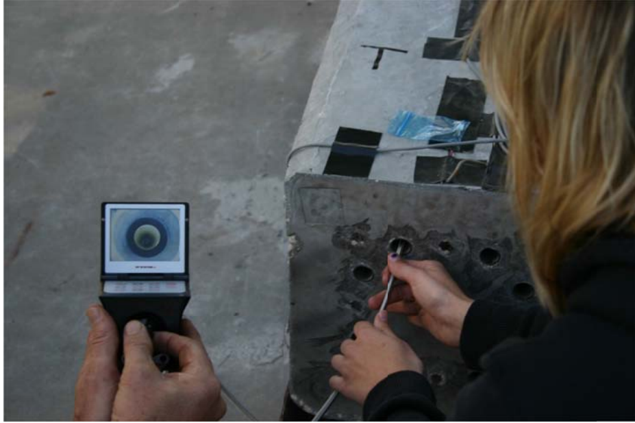
Figure 4.46. Real-time imaging of duct cleanliness.
