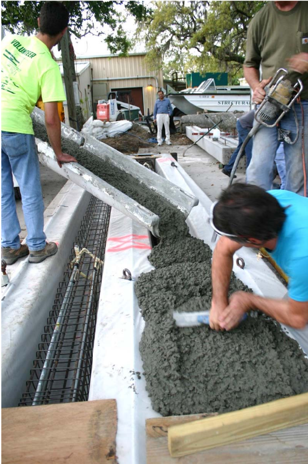
Figure 4.76. Concrete placement with 5.5in slump; control pile 2 left, splice pile 2 right.
