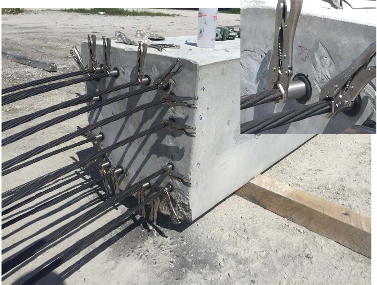
Figure 6.19. Upper pile segment with all splicing strands inserted and clamped complete with alignment dowels and neoprene gaskets.
