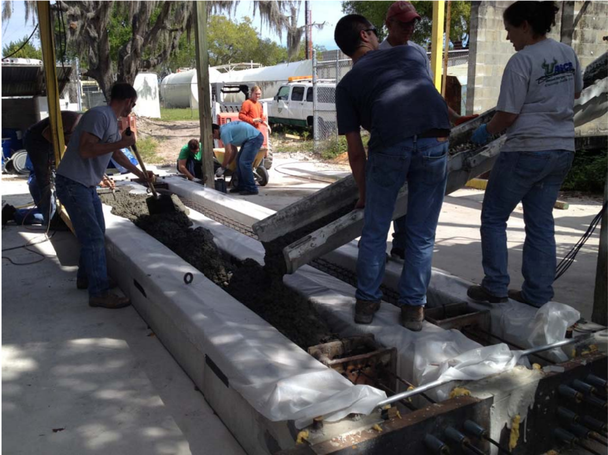
Figure 4.29. Concrete placement with 4.5in slump; east pile (control) to the right.
