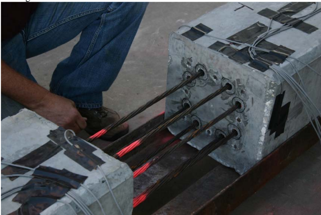
Figure 4.55. All strands embedded past anchorage wedges (lower pile right).
