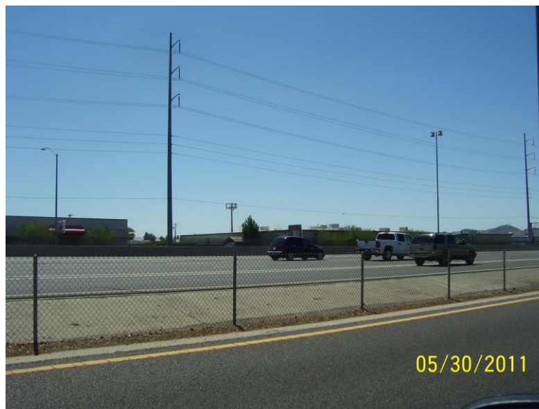
Figure 5. Example of Chain Link Fence Barrier along Main Lanes (Source: Will Bozeman).
