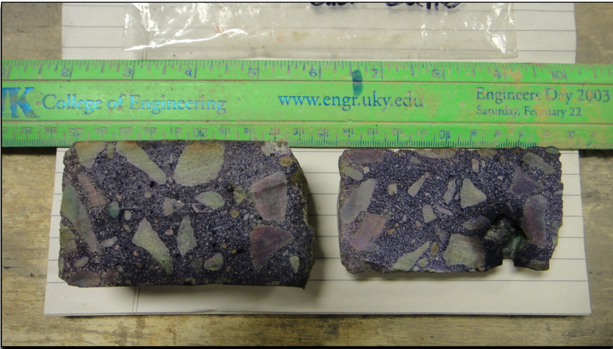
Figure 105. Bridge #047B00116N Core Sample, Post-Spray
