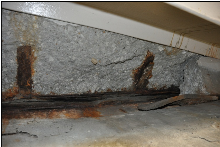
Figure 18. I-65 over Fairgrounds entrance from Bradley Ave., Joint seal area
