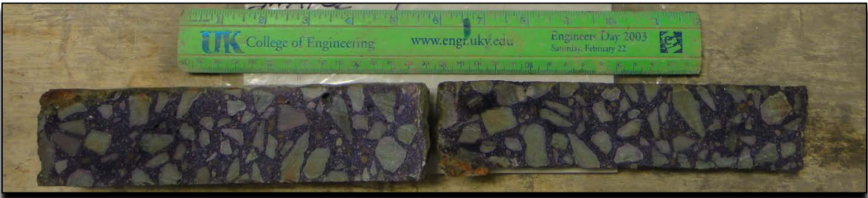
Figure 117. Bridge #043B00026R Core Sample, Post-Spray
