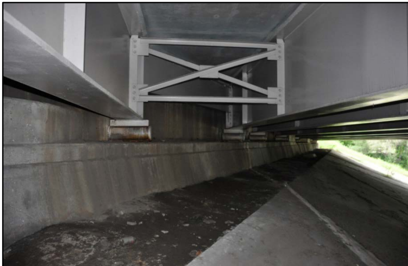
Figure 366. I-65 over S. Floyd St., Staining on back wall and abutment
