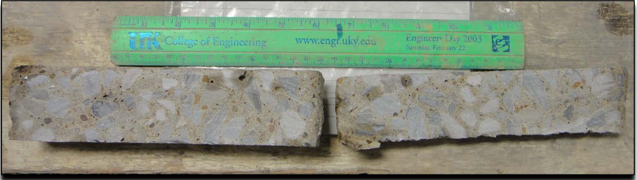
Figure 116. Bridge #043B00026R Core Sample, Pre-Spray
