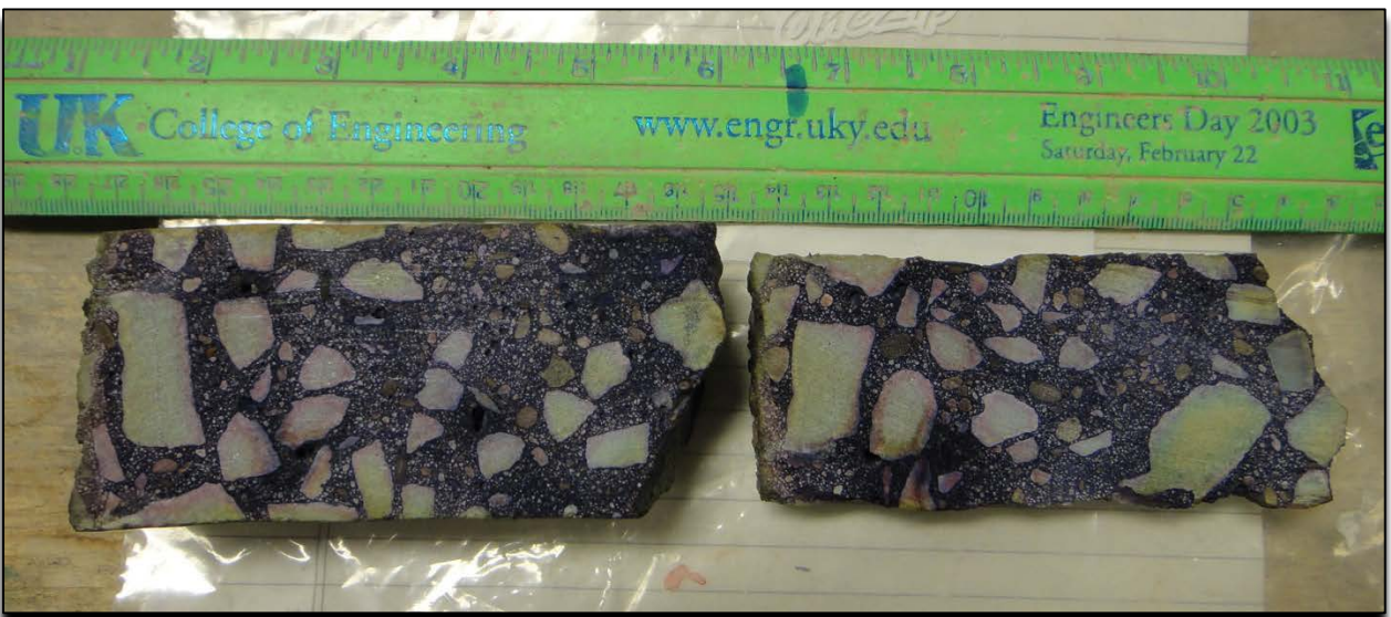
Figure 113. Bridge #103B00029N Core Sample, Post-Spray
