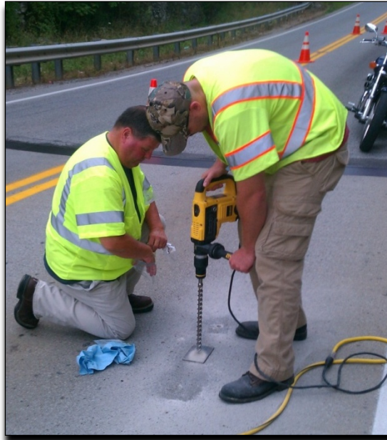
Figure 4. Drilling for Powder Sample
