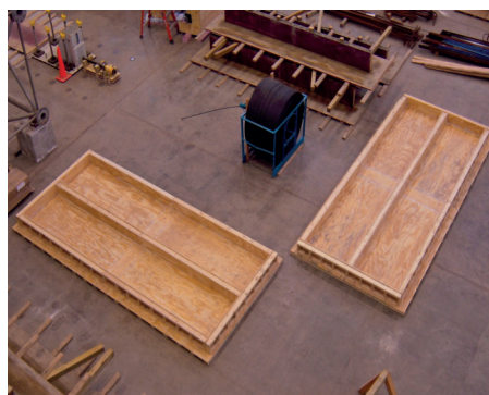
(a) Slab Formwork
