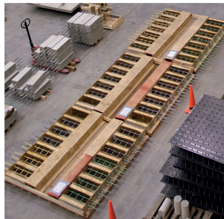
(b) Formwork and reinforcement
