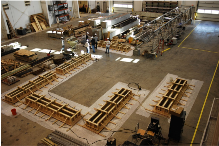
Figure B.13 Assembled formwork (series II).
