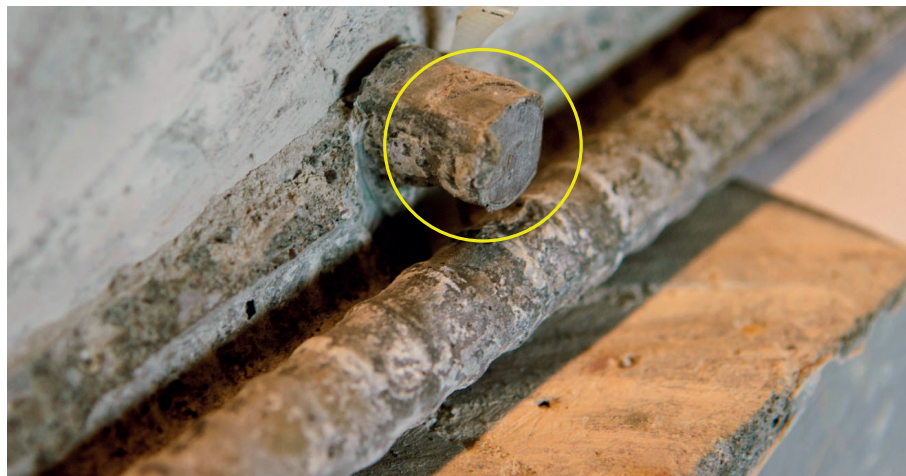
(b) White Corrosion and Consumption of Zinc-clad on Transverse Steel
