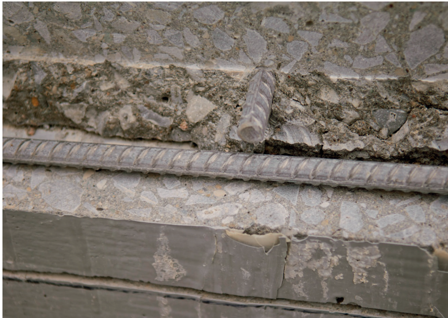
(b) No Corrosion Observed
