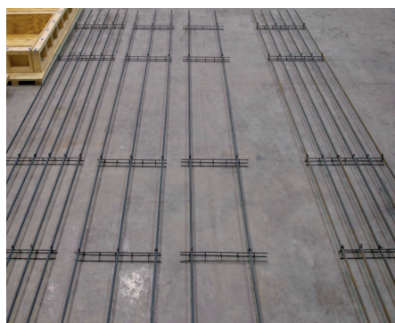
(b) Reinforcing Steel Layout
