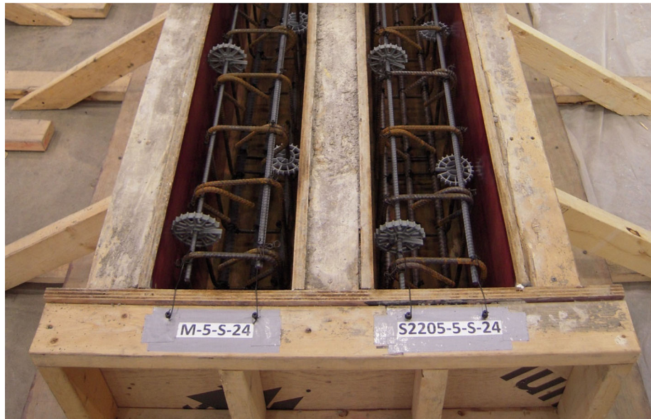
Figure B.17 Plastic spacer wheels (series IV).
