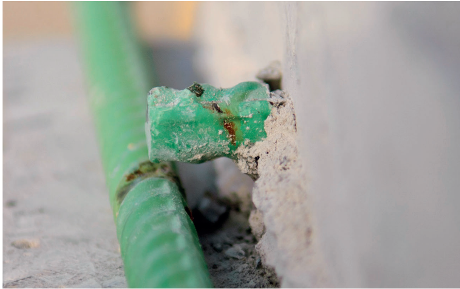
(a) Corrosion on Transverse Bar with Black Tie
