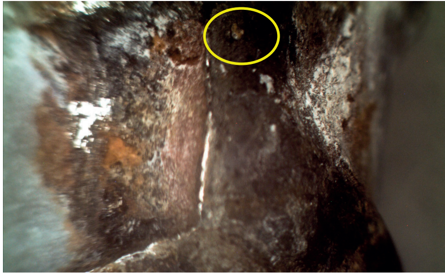
(a) Pitting Corrosion on Transverse Steel
