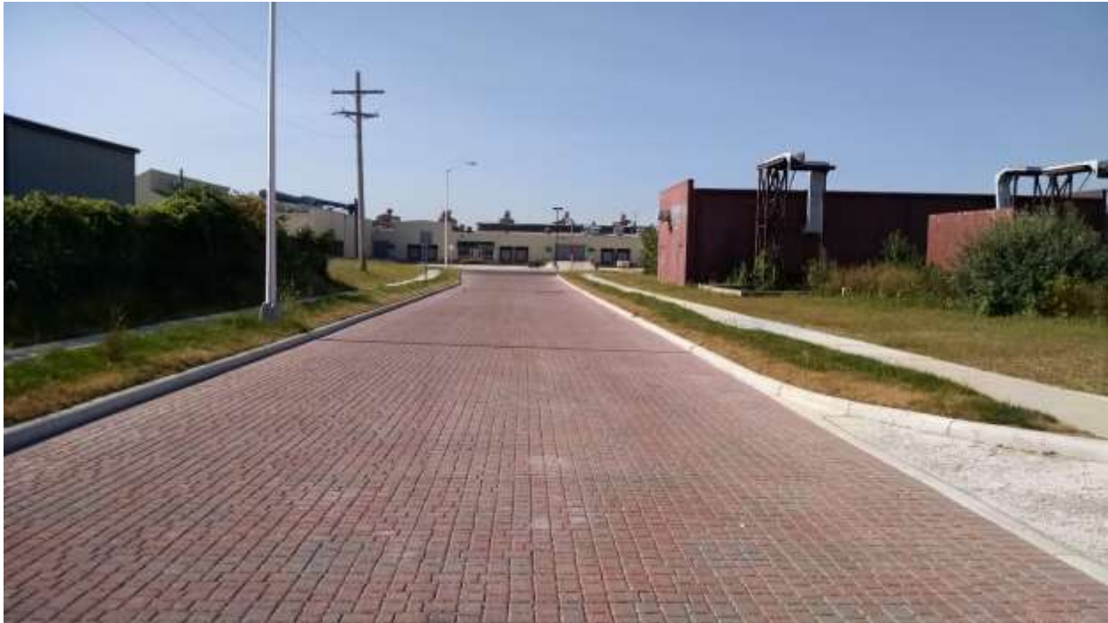
FigureD-7. Tech South permeable pavement project after construction completed
