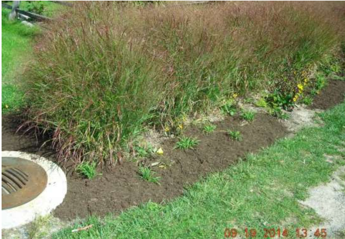
Figure D-2. Detail of plantings and outlet for the bioretention area for Angola Road
