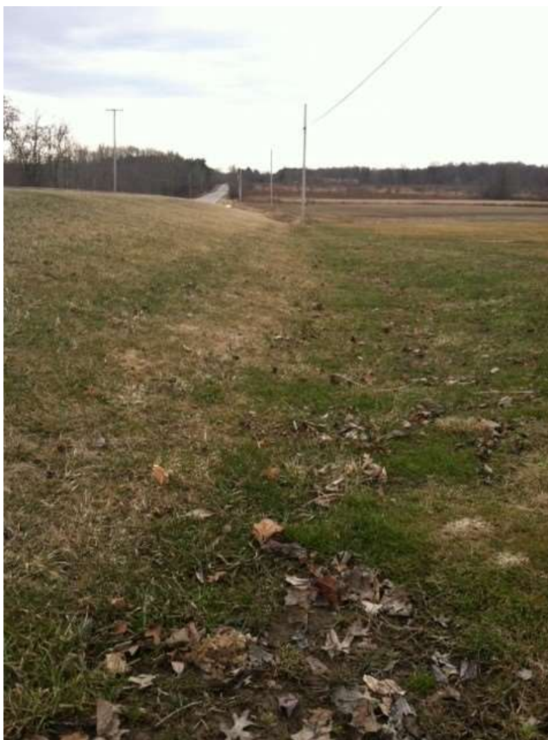
Figure D-11. The established vegetated swale after construction of the MAH-45 Project
