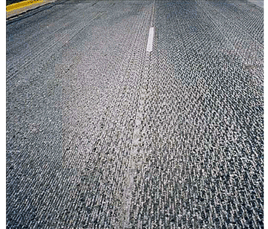
Asphalt removed by milling can be recycled and reused to pave again.
