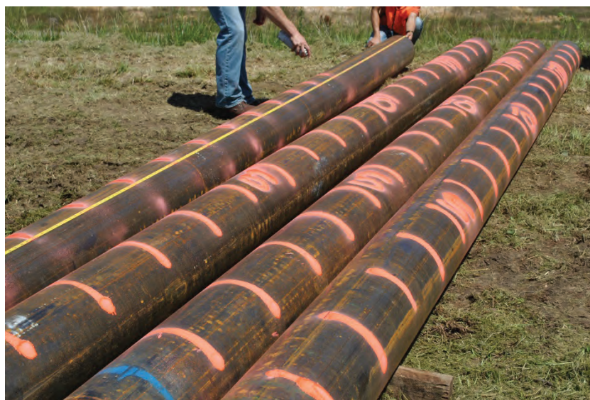
Figure 3.12. 1-ft intervals marked on piles.
