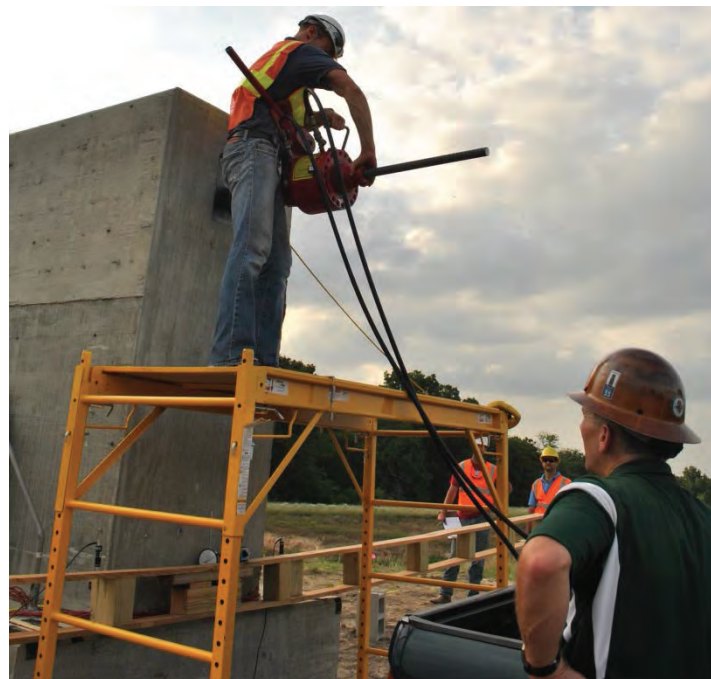
Figure 3.53. Resetting stroke of the hydraulic jack during the load test.
