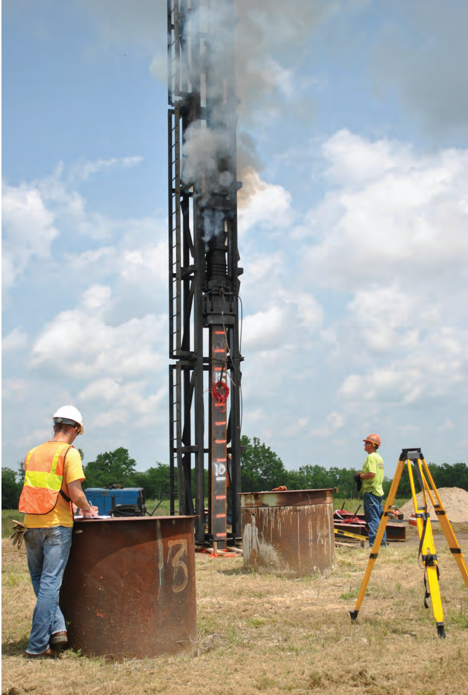
Figure 3.10. Crew monitoring pile driving.
