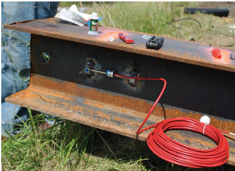
Figure 3.35. Installed Geokon 4000 gage at pile tip.
