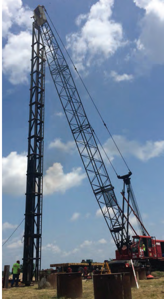
Figure 3.9. Crane and hammer leads used for pile driving.
