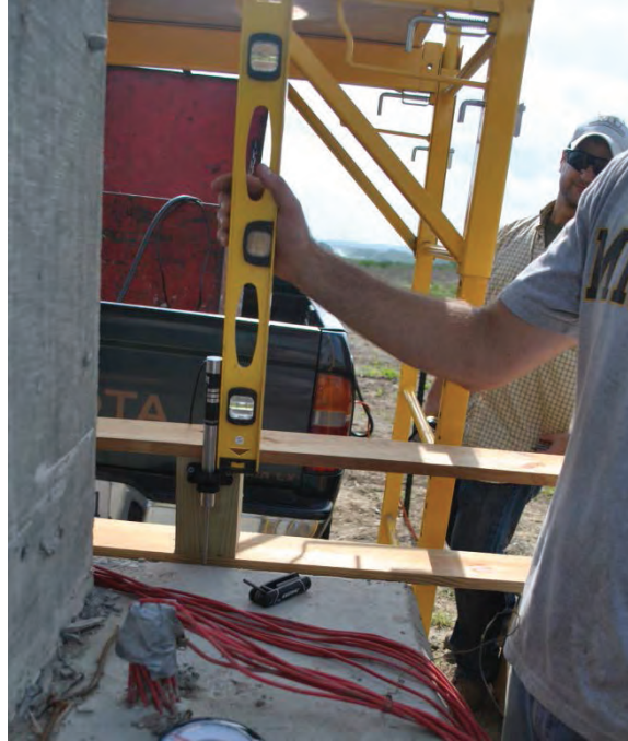
Figure 3.45. Installation of uplift LVDT.
