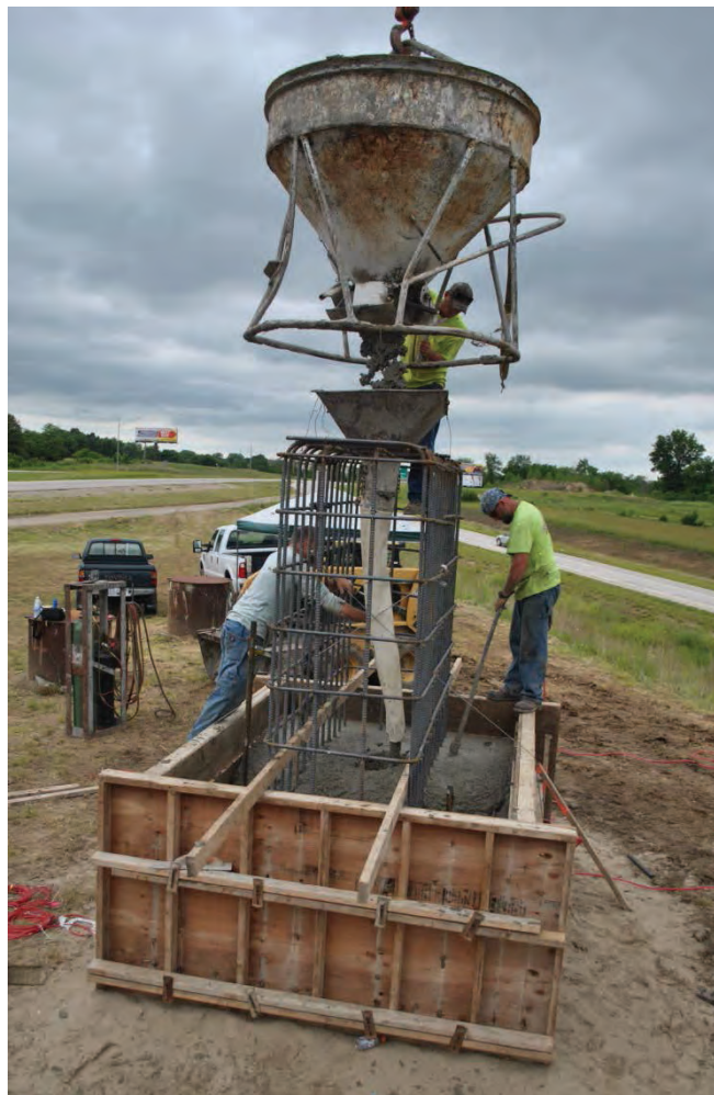
Figure 3.26. Placing concrete for H-pile cap.
