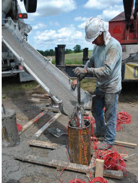
Figure 3.18. Placing concrete in CIP-2.
