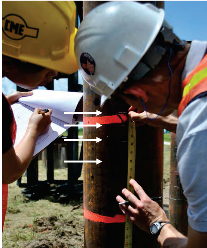
Figure 3.14. Measured final pile penetration after driving.
