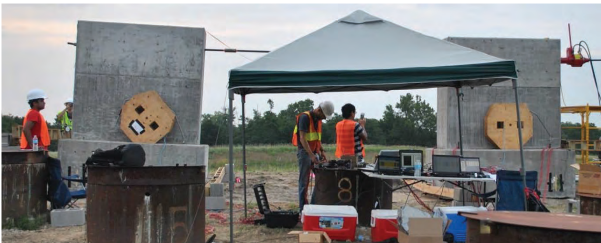
Figure 3.55. Pile structures during final load step. H-pile cap is at left and CIP pile cap is at right.
