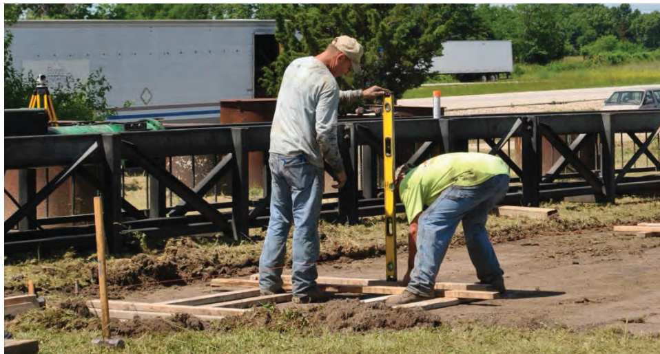
Figure 3.8. Crew places template for piles on level work surface.
