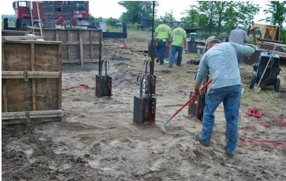
Figure 3.22. Crew levels sand prior to placing forms for pile cap.
