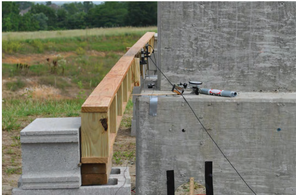
Figure 3.42. LVDTs positioned above rear of pile caps to measure uplift.
