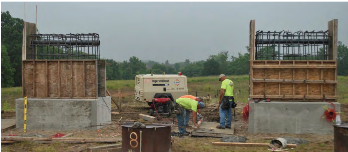
Figure 3.30. Forming stems. Pipes for threadbar load application are in place.
