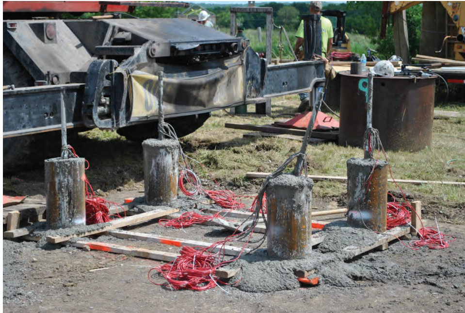
Figure 3.20. CIP Pile group after driving, prior to placement of sand.
