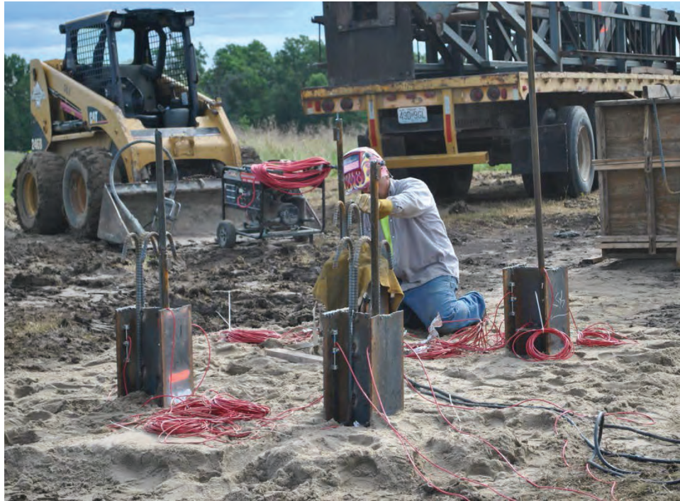
Figure 3.34. Welding Geokon 4000 gages to pile head after driving.
