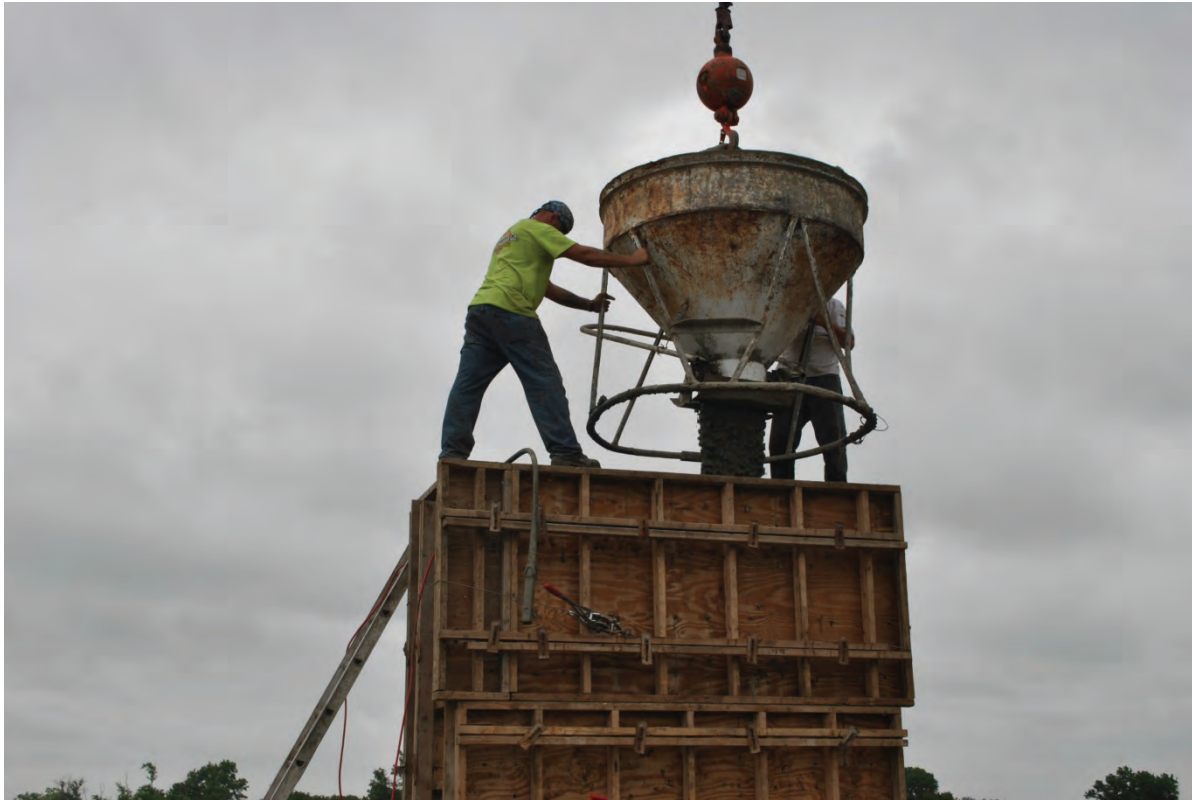
Figure 3.31. Placing concrete for stems.
