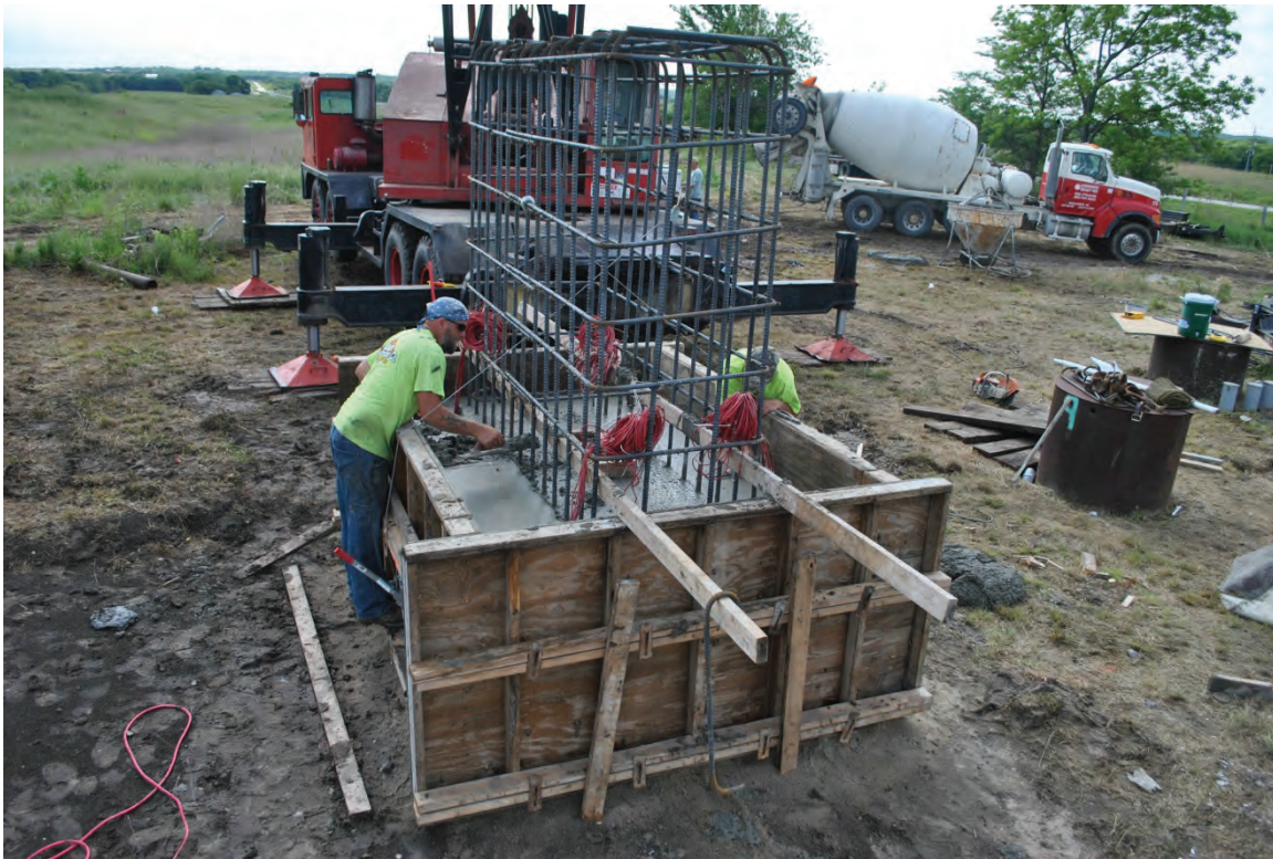
Figure 3.28. Finishing concrete for pile cap.
