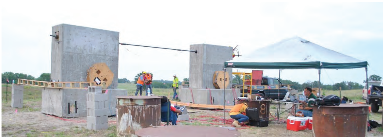
Figure 3.52. View of load test with H-pile group on left and CIP pile group on right.
