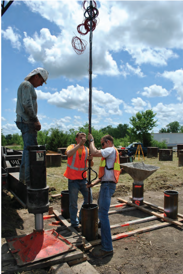
Figure 3.17. Placing instrumented pipe into CIP pile.
