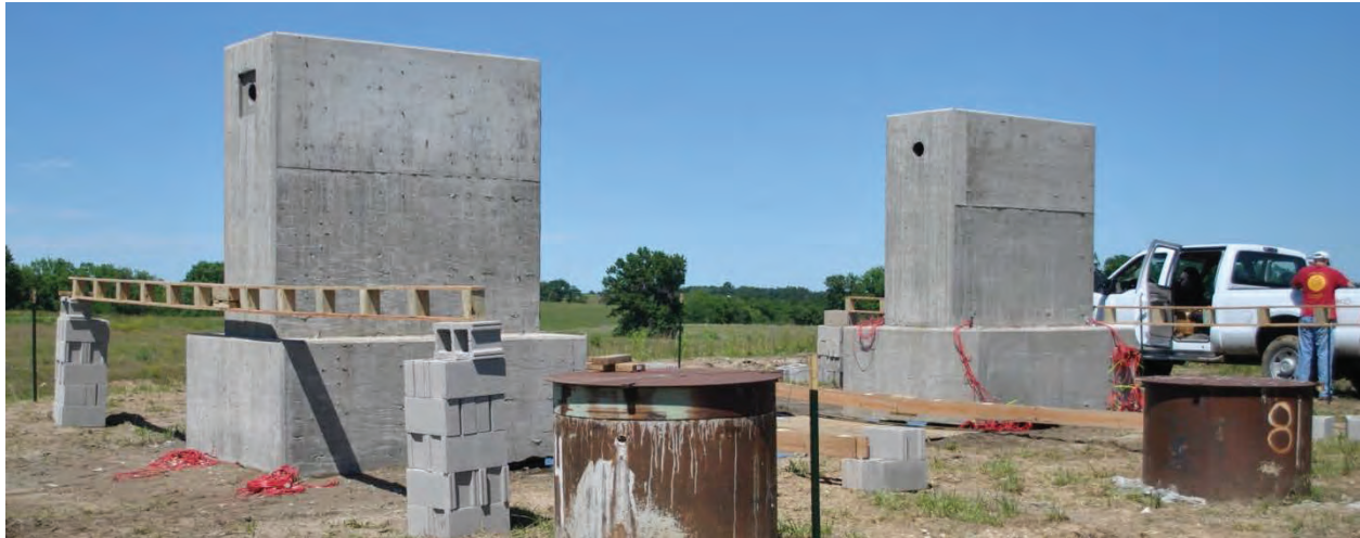
Figure 3.33. Completed pile cap-stem structures.
