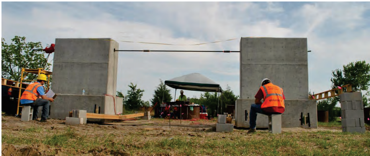
Figure 3.51. View of load test with CIP pile group on left and H-pile group on right. Canopy housing computers and DAQs is in background.
