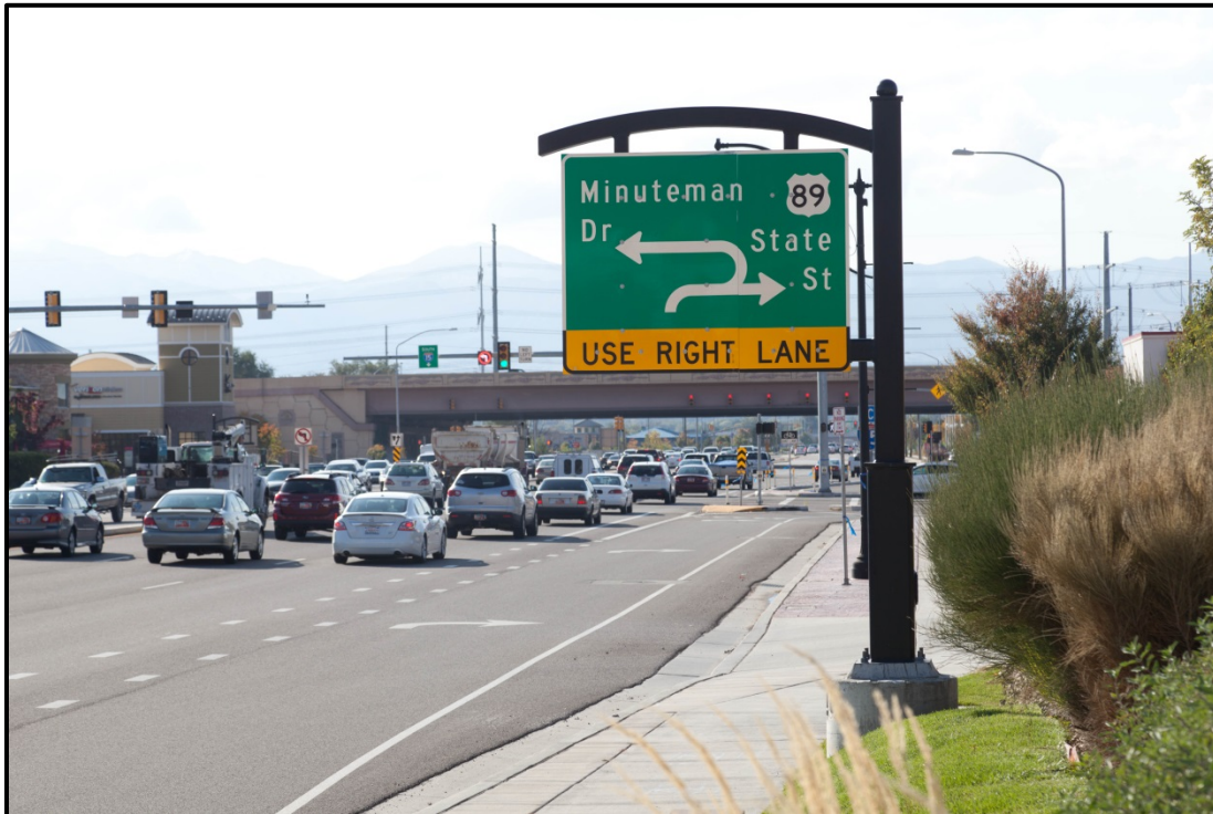
Exhibit 1-10. Advance signing at a MUT intersection in Draper, Utah. (3)
