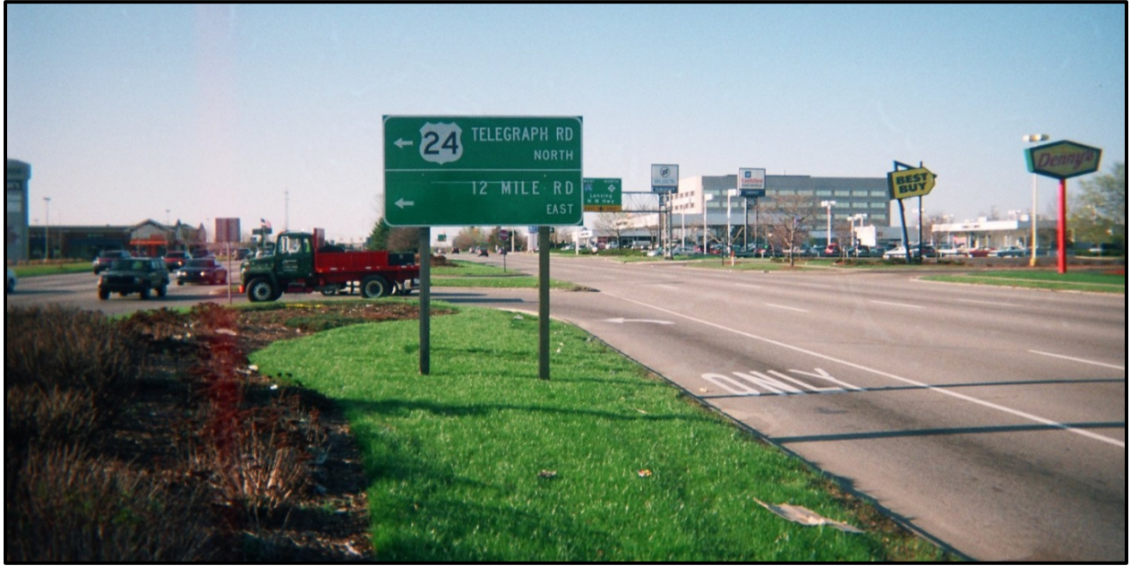
Exhibit 1-13. MUT crossover intersection in Southfield, Michigan. (4)
