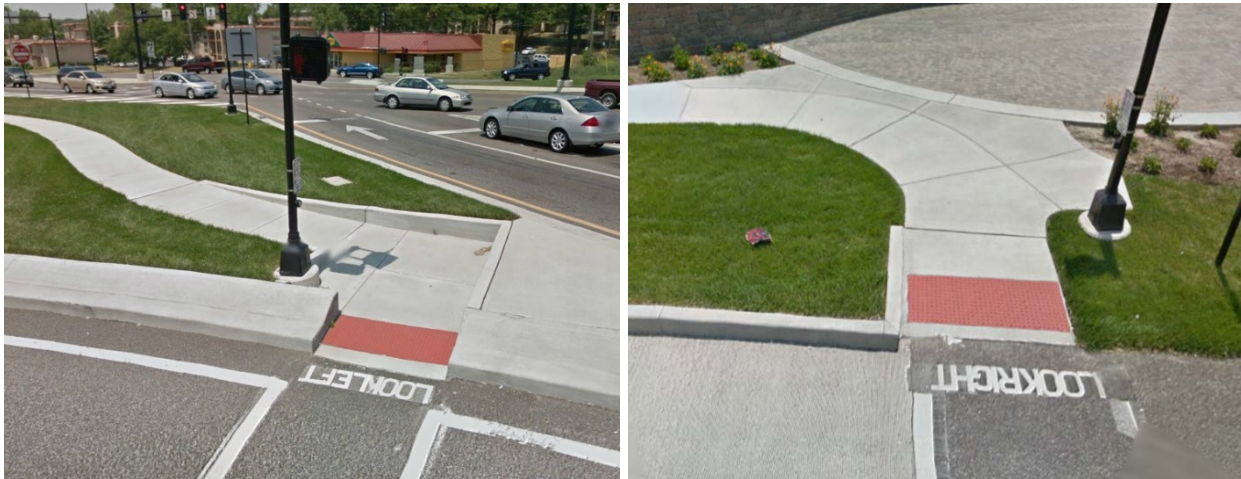
Exhibit 3-17. Pedestrian markings to indicate directionality of traffic (Maryland Heights, MO). (14)
