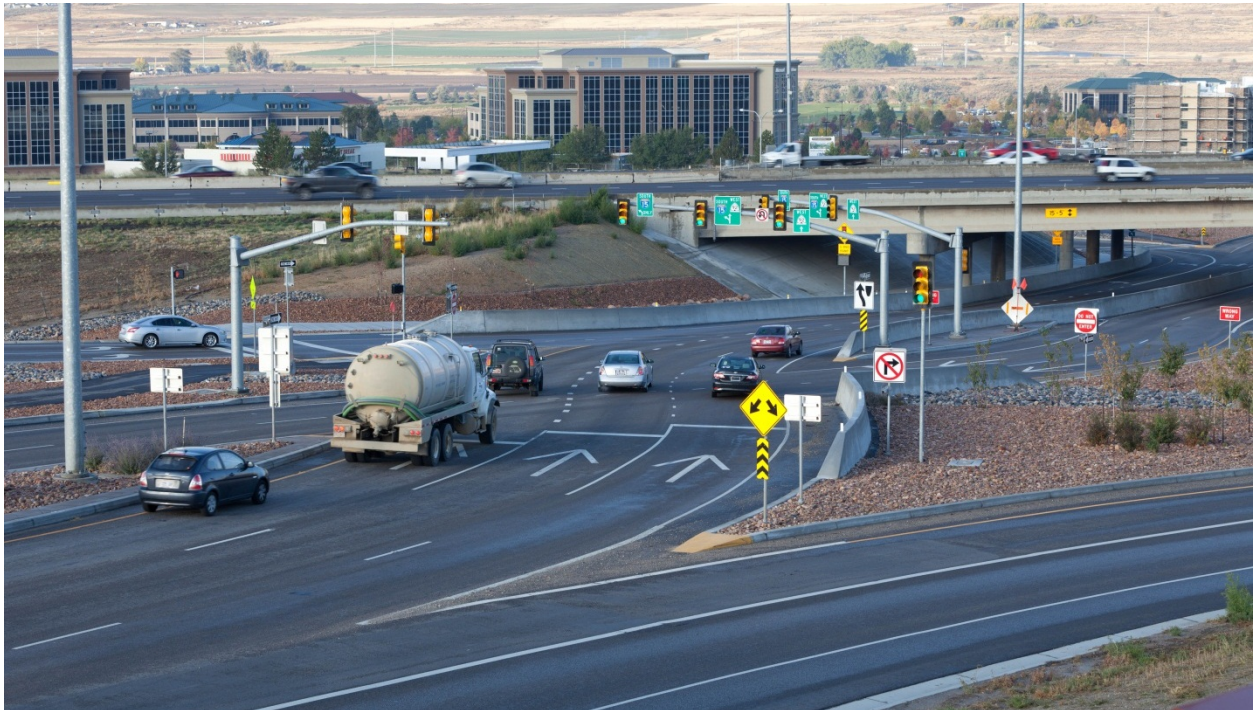
Exhibit 1-7. Crossover location at the DDI located at SR 92 and Interstate 15 (Utah County, UT). (5)
