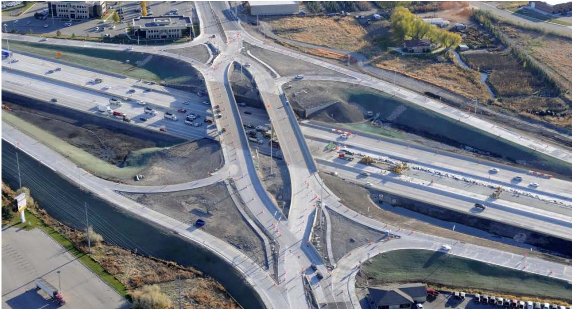
Exhibit 1-11. DDI (overpass) at 500 East American Fork (American Fork, UT). (1)
