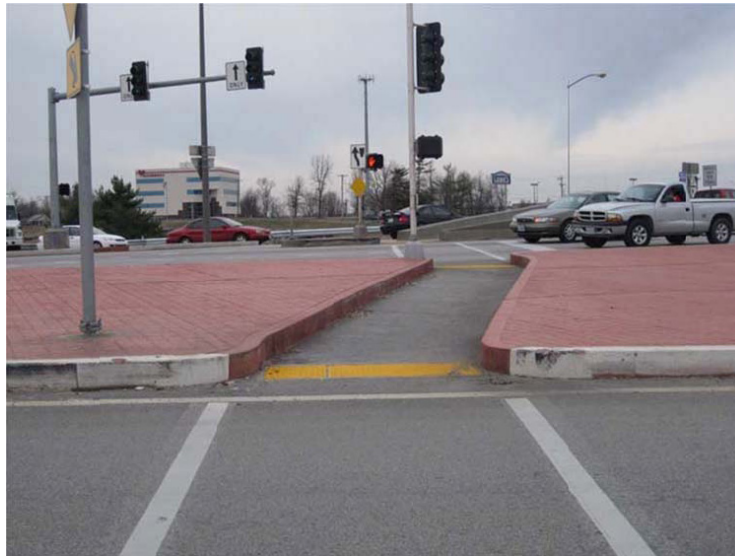
Exhibit 3-20. Example of pedestrian wayfinding provision at DDI via curbing. (26)
