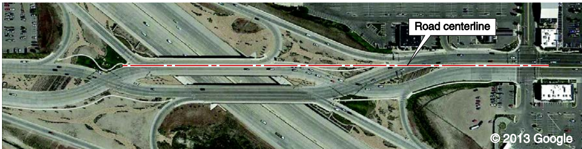
Exhibit 7-12. Shifted alignment south of centerline (red) with no reverse curves between crossovers (Pioneer Crossing, American Fork, UT). (26)
