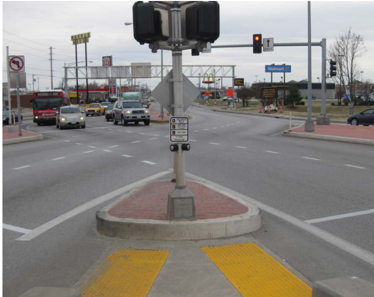
Exhibit 8-10. Undesirable use of single pole with two pedestrian push-buttons, no APS, and insufficient separation of the two detectable warning surfaces. (26)
