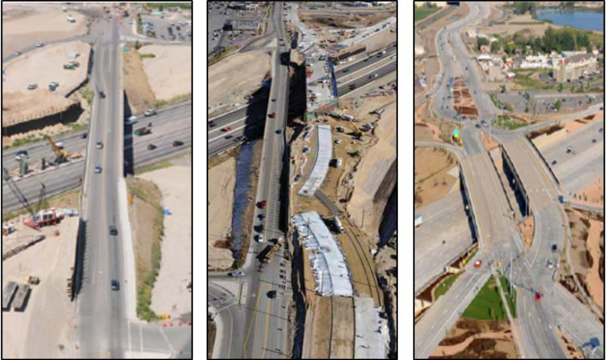
Exhibit 9-3. Construction staging using pre-cast construction methods. (48)
