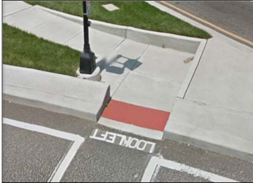
Exhibit 8-30. Engraved pedestrian pavement marking – “Look Left.” (26)
