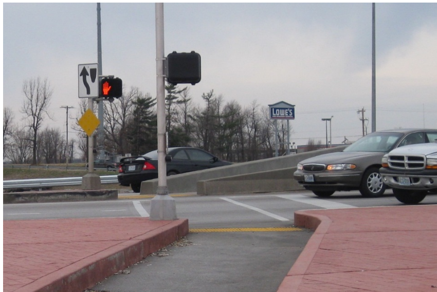
Exhibit 8-13. Pedestrian signal and push-button on outside of crossover (pedestrian facilities in center). (14)
