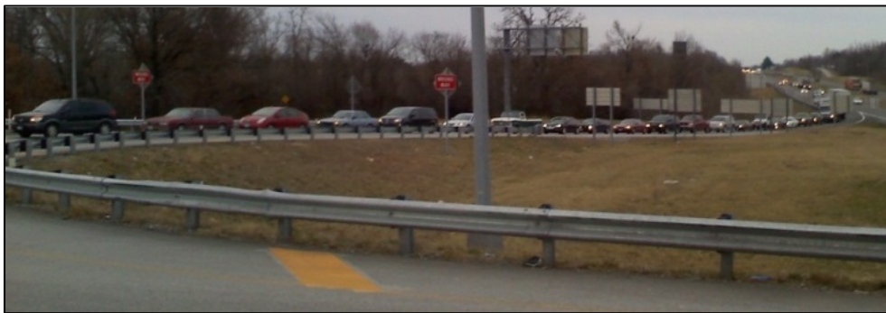
Exhibit 5-9. Queue spillback caused by heavy traffic volumes and a no RTOR condition. (14)
