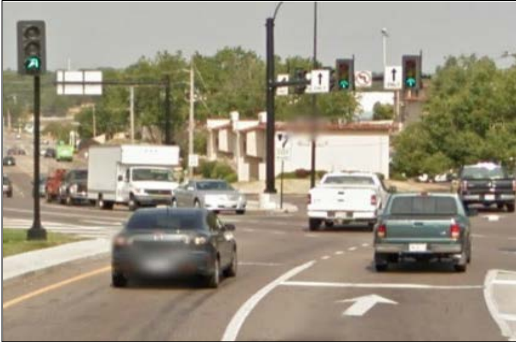
Exhibit 7-27. Supplemental advanced signal at crossover. (26)
