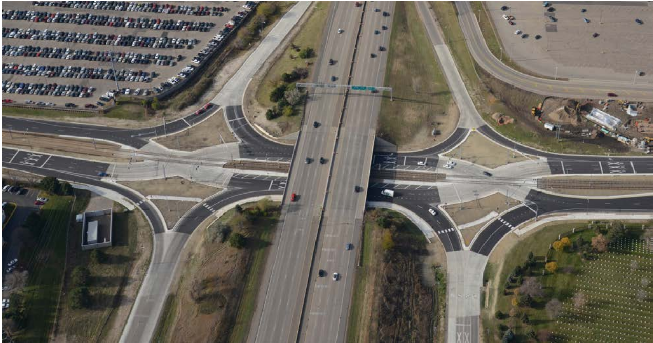
Exhibit 3-28. Aerial view of DDI with center-running light rail at I-494 and 34 th Avenue in Bloomington, MN. (29)
