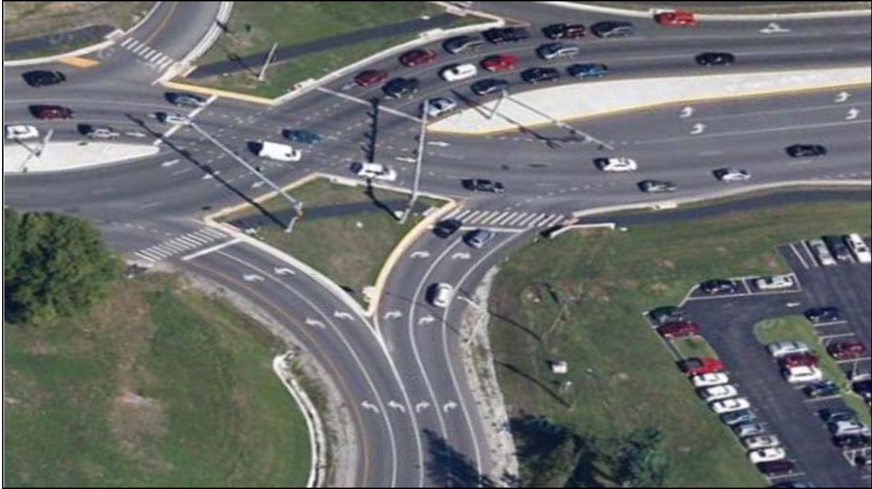
Exhibit 8-23. Lane line markings at crossover and ramp terminal approaches. (26)
