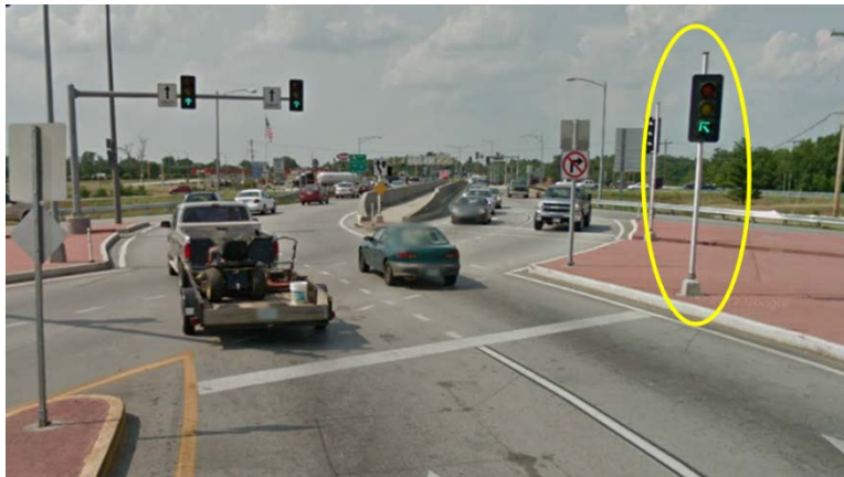
Exhibit 8-6. Supplemental signal on right for an inbound movement at a DDI. (26)
