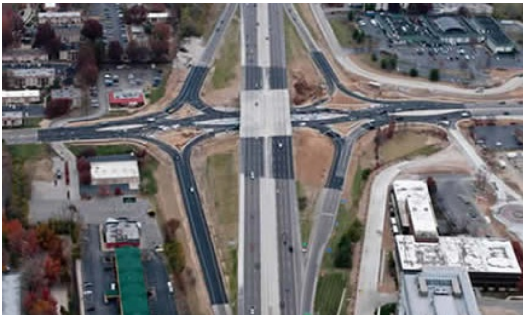
Exhibit 1-12. DDI (underpass) at Dorsett Road and Interstate 270 (St Louis, MO). (7)
