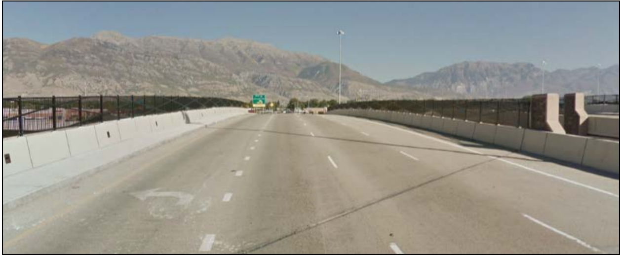
Exhibit 8-24. Use of short skip lines to delineate an exclusive left turn lane onto a limited access facility. (26)
