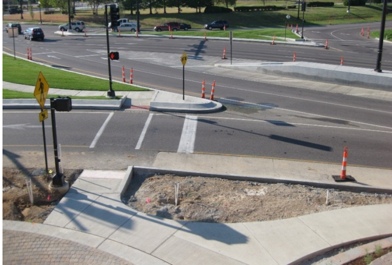
Exhibit 8-14. Pedestrian signal for left-turn onto freeway (pedestrian facilities on outside). (14)
