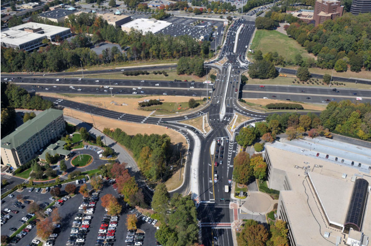
Exhibit 1-4. First constructed DDI in Georgia at Ashford Dunwoody Road near Perimeter Market. (2)
