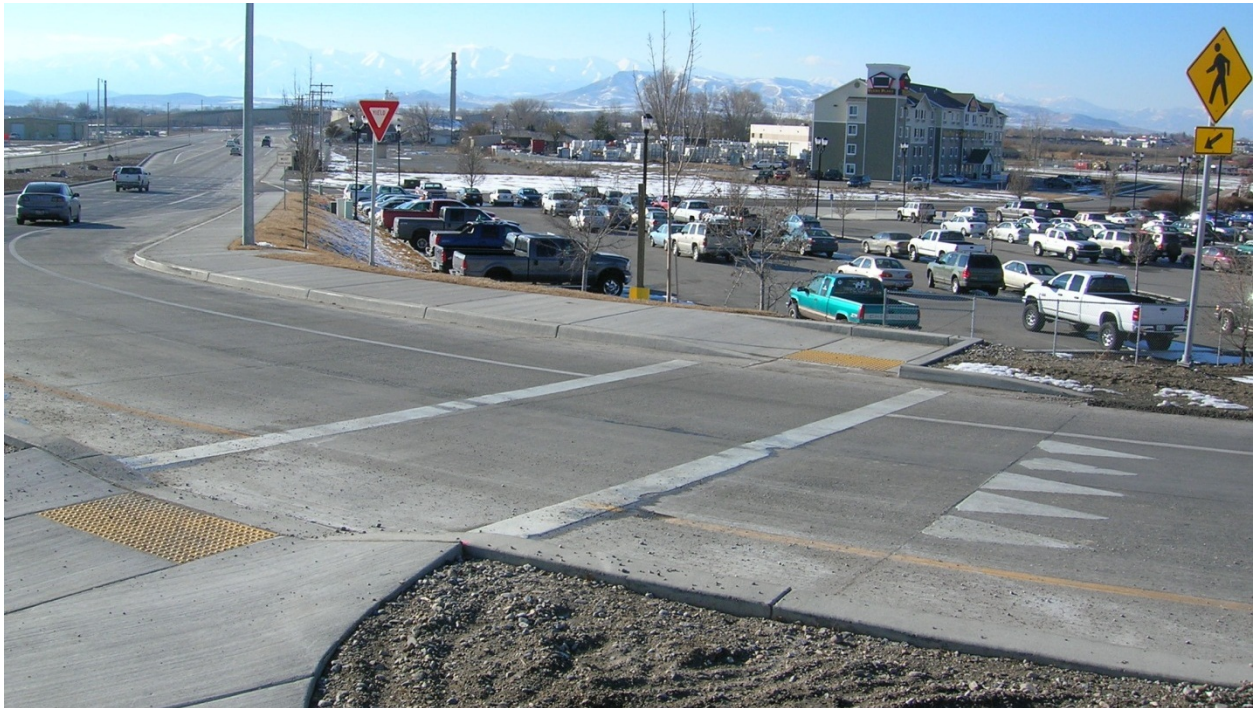
Exhibit 1-9. Pedestrian crossing at the right-turn lane of the exit located at Pioneer Crossing and Interstate 15 DDI (American Fork, UT). (6)
