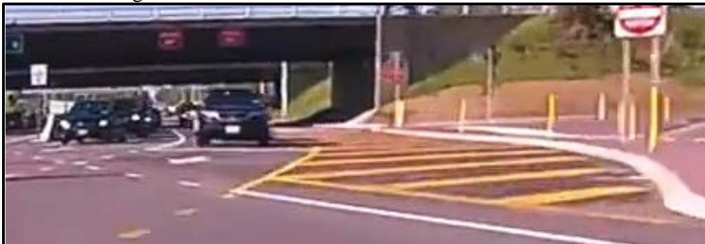
Exhibit 4-8. Southbound outer-most lane closed and marked with pavement markings. (26)
