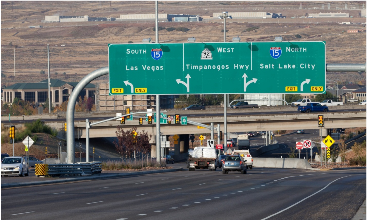
Exhibit 1-8. Overhead signing at the DDI located at SR 92 and Interstate 15 (Utah County, UT). (5)
