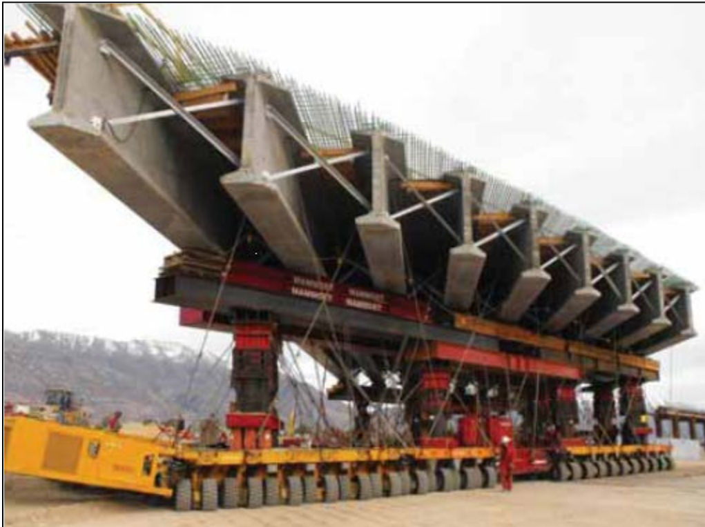
Exhibit 9-2. Self-propelled modular transporter (SPMT) brings superstructure to DDI location. (48)
