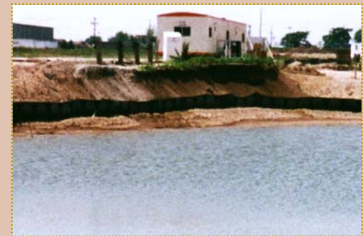
Construction site in summer of 1999.
